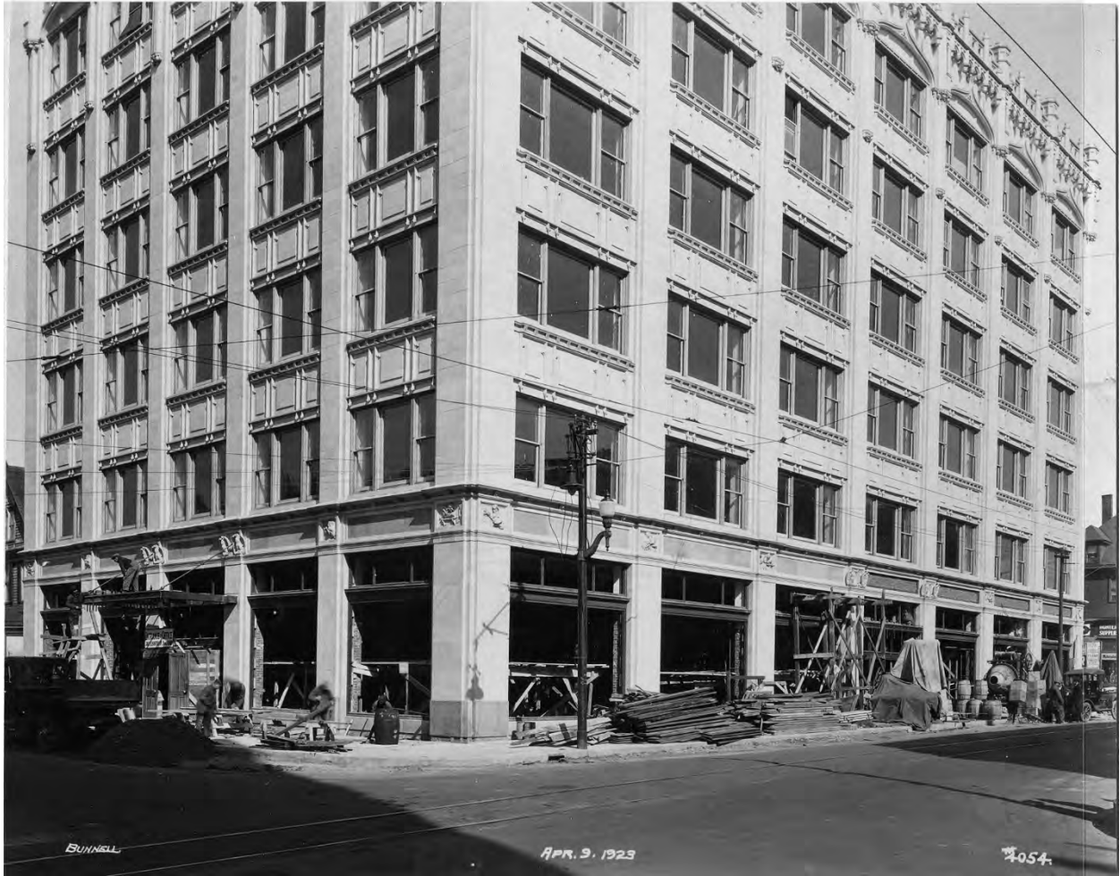
Figure 11 – View of the Stoehr & Fister Building under construction in April 1923.
