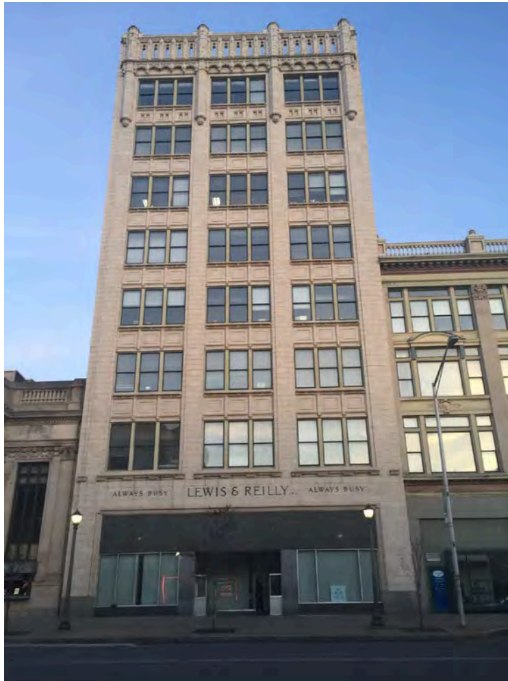
Figure 17 – Current view of the Lewis & Reilly Building (1925) at 114 Wyoming Ave, Scranton, PA..
