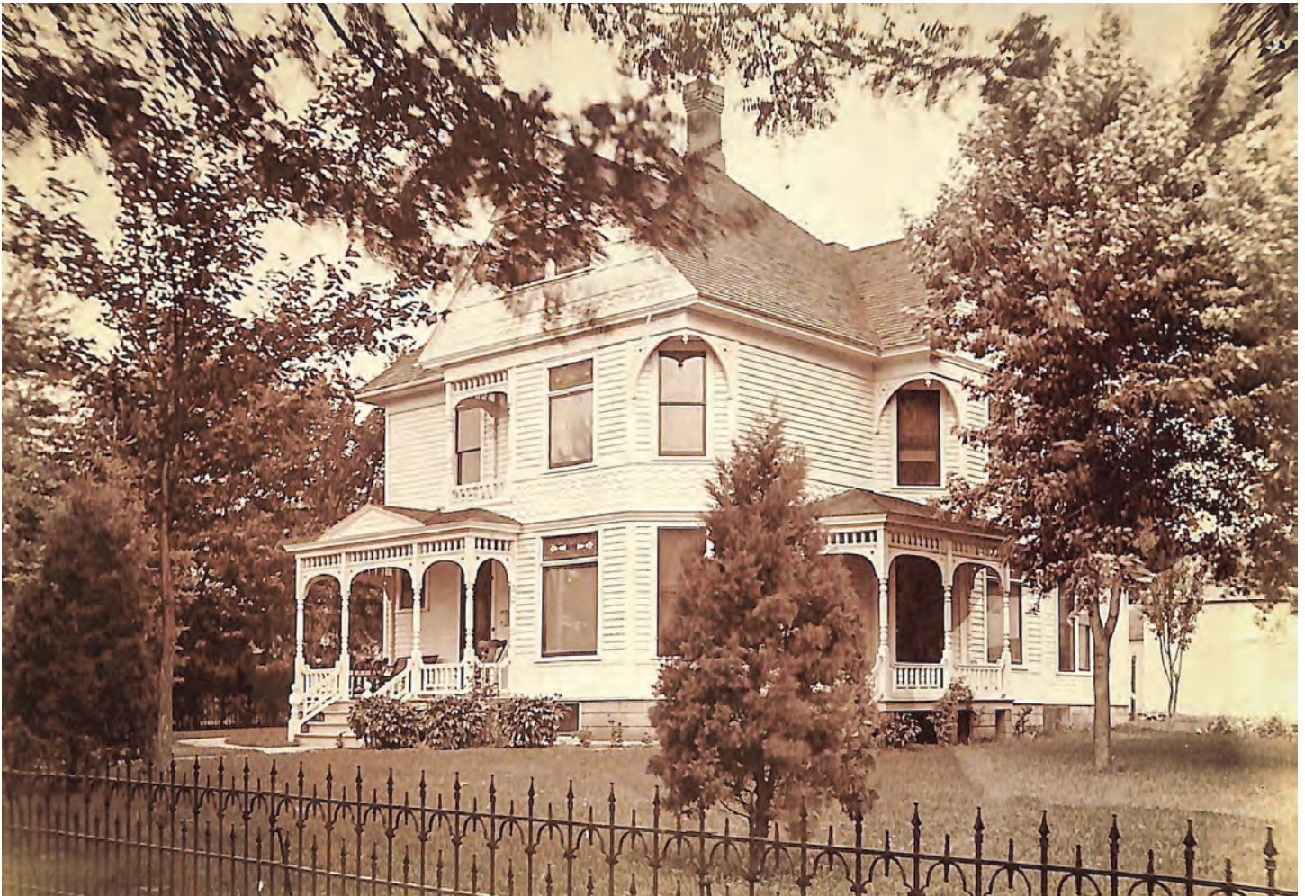
Figure 6. Historical view of the Lemuel C. and Mary (Vaughn) Boughton House, 736 W. Cedar Street. This undated photograph was taken after 1891, when the house was completed, and before 1914, by which time the two small spindlework porches shown here were replaced by the present wraparound porch constructed of concrete blocks. Source: Cherokee Area Archives, Cherokee Public Library, Cherokee, Iowa.
