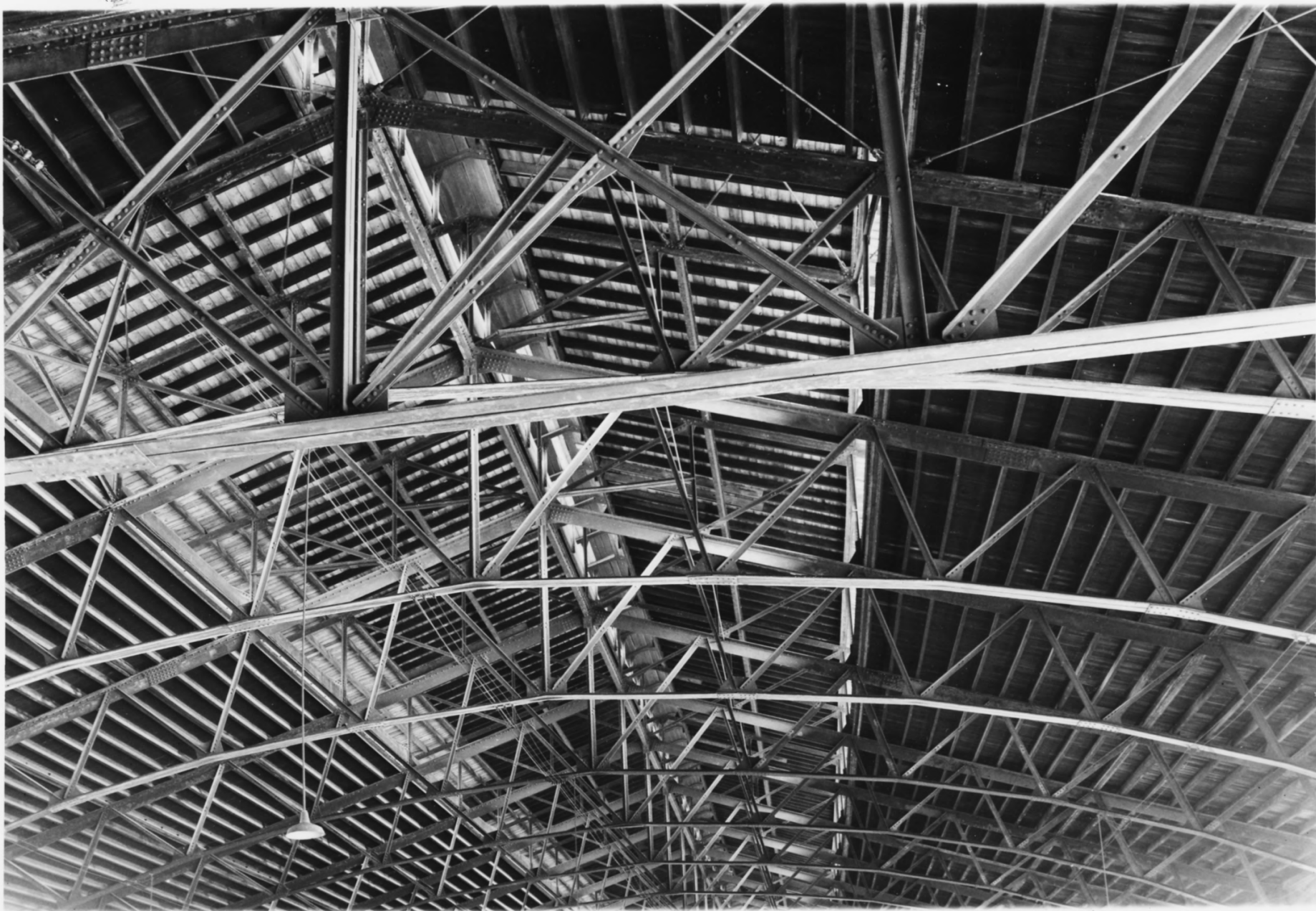
New Union Station, Richmond, Virginia 1520 East Main Street
