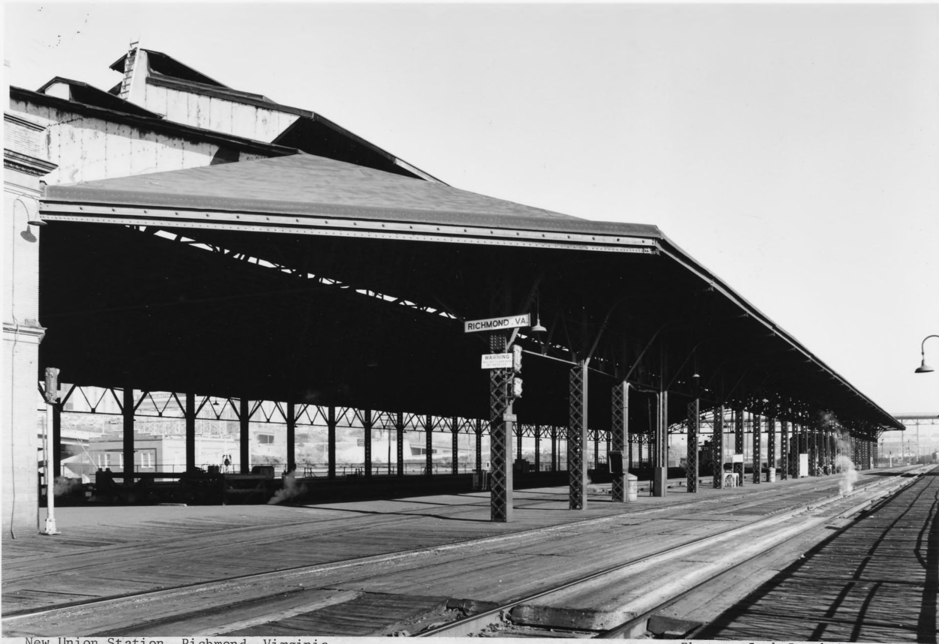
New Union Station, Richmond, Virginia 1520 East Main Street
