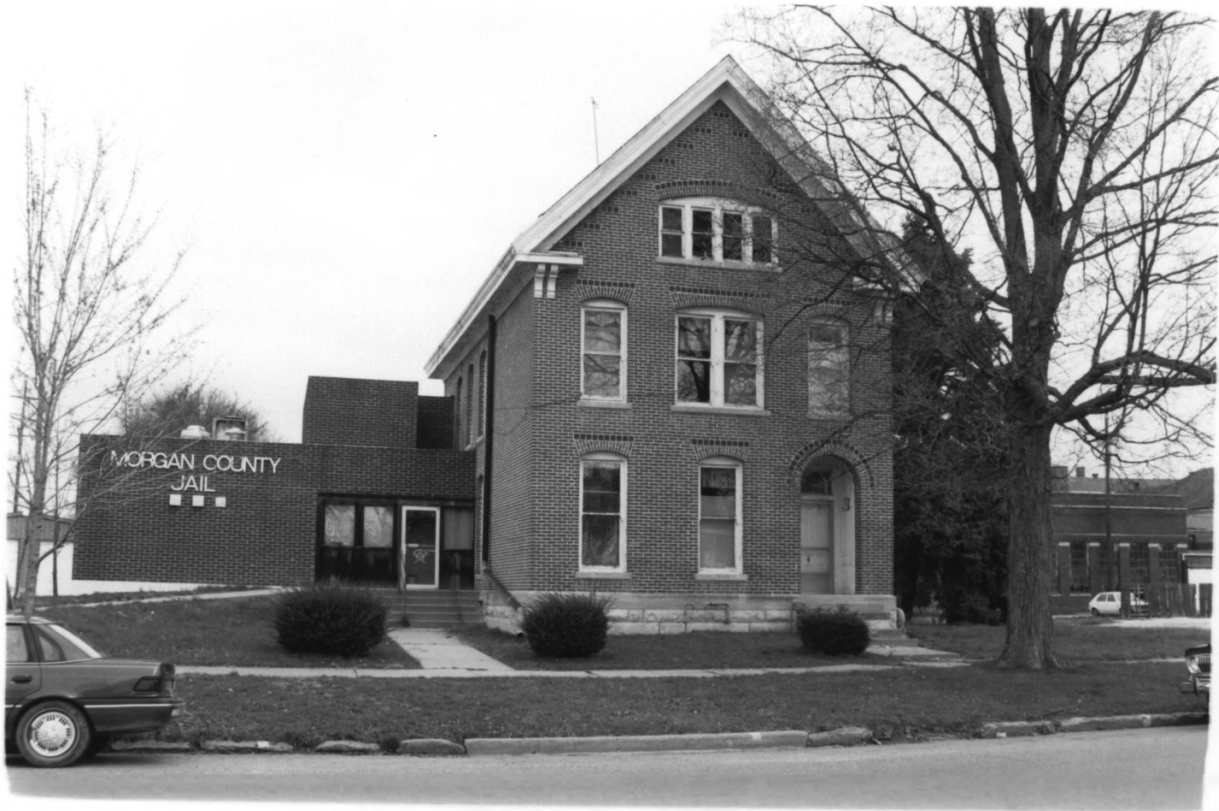
1 Morgan County Sheriff's Residence and Jail Martinville, Indiana
