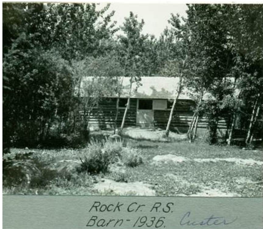
Figure 1. Barn within the Rock Creek Ranger Station complex, ca. 1936 (Image courtesy of CGNF Billings Office).
