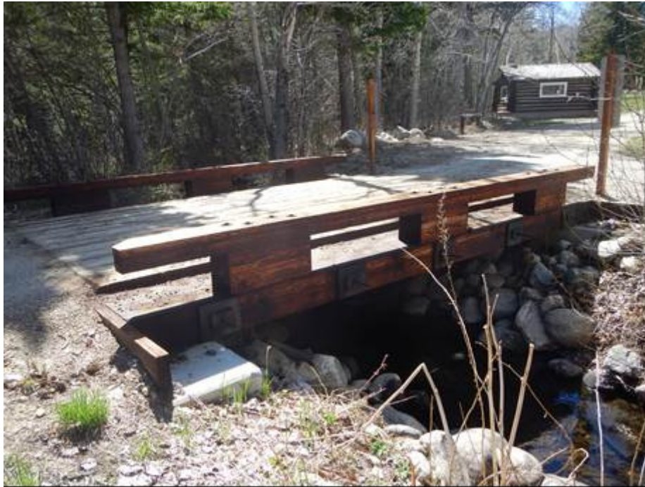
Photograph 14. MT_CarbonCounty_RockCreekRangerStationHD_0014. Bridge, facing southwest (Source: Logan Simpson, 2015).
