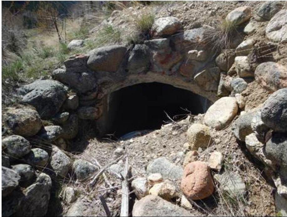
Photograph 17. MT_CarbonCounty_RockCreekRangerStationHD_0017. Maryott Ditch, showing the stone and concrete culvert on the east side of the District's access road, facing west (Source: Logan Simpson, 2015).
