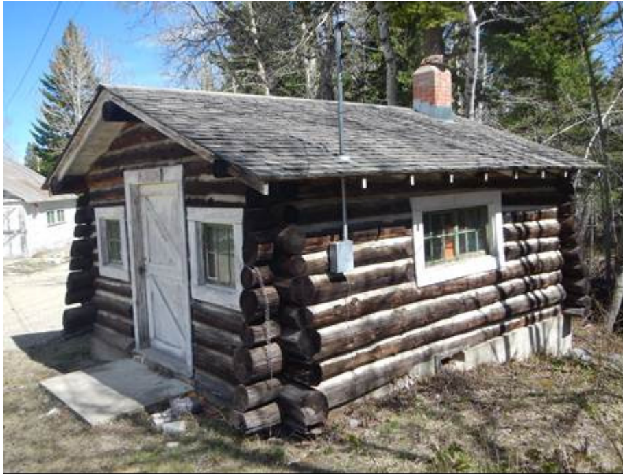
Photograph 3. MT_CarbonCounty_RockCreekRangerStationHD_0003. Storehouse/fire cache building (Building #2301), facing east (Source: Logan Simpson, 2015).
