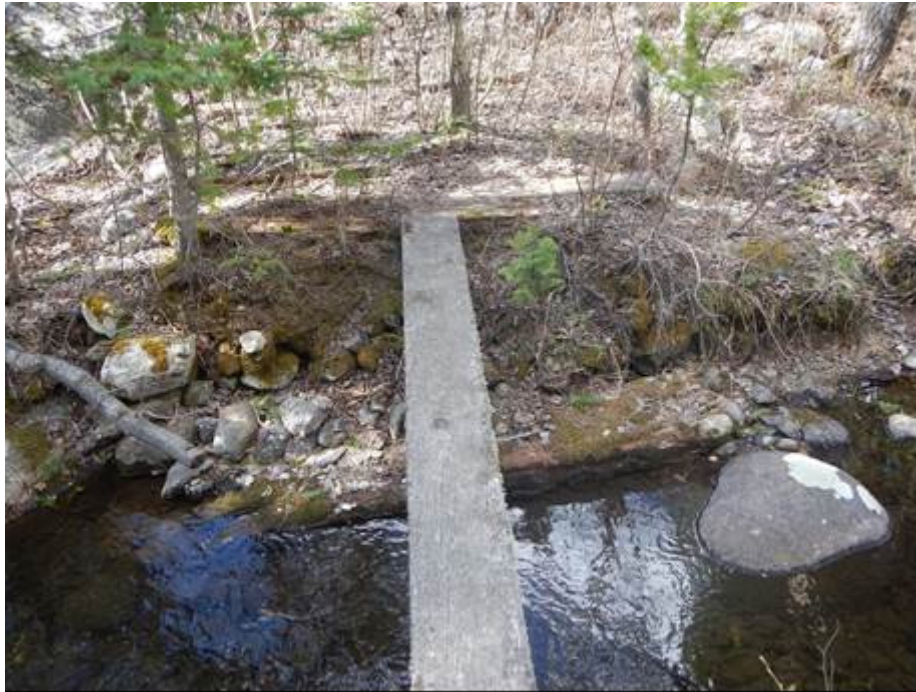
Photograph 21. MT_CarbonCounty_RockCreekRangerStationHD_0021. Remnants of a bridge spanning the West Fork Ditch Company canal, facing north. Note that the former bridge abutments are currently being used to support a wooden plank footbridge.
