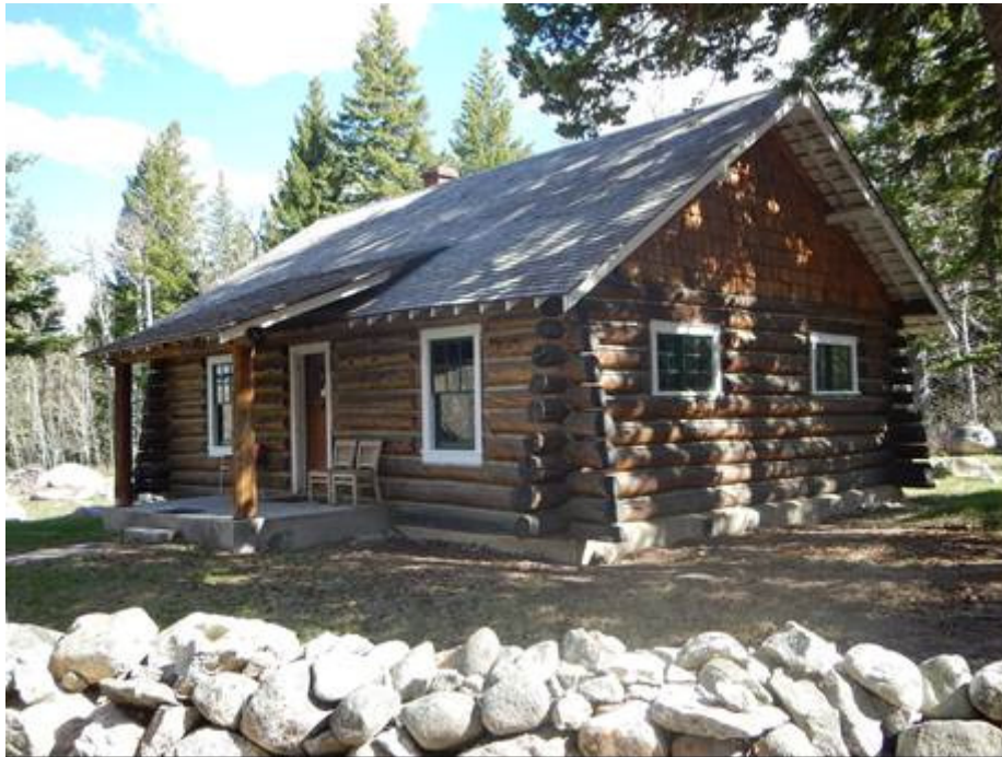
Photograph 1. MT_CarbonCounty_RockCreekRangerStationHD_0001. Northern (main) and western elevations of the Main Cabin (Building #1010), facing southeast (Source: Logan Simpson, 2015).
