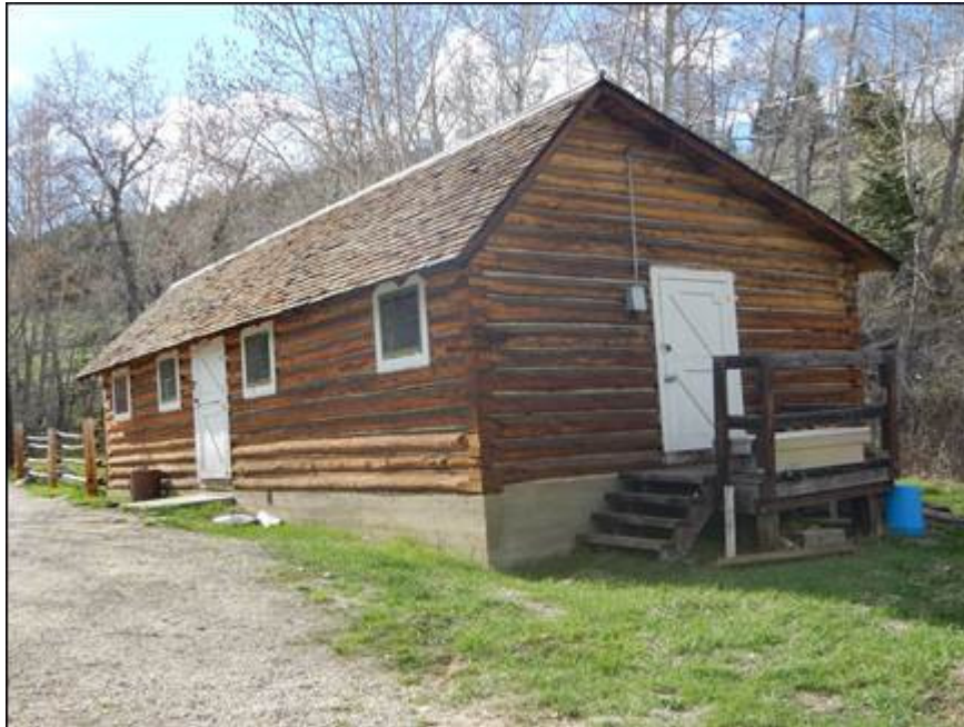
Photograph 4. MT_CarbonCounty_RockCreekRangerStationHD_0004. Barn (Building #2401), facing northwest (Source: Logan Simpson, 2015).
