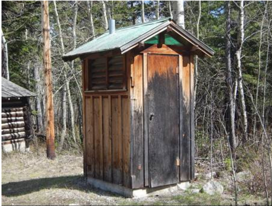
Photograph 8. MT_CarbonCounty_RockCreekRangerStationHD_0008. Outhouse, facing southeast (Source: Logan Simpson, 2015).
