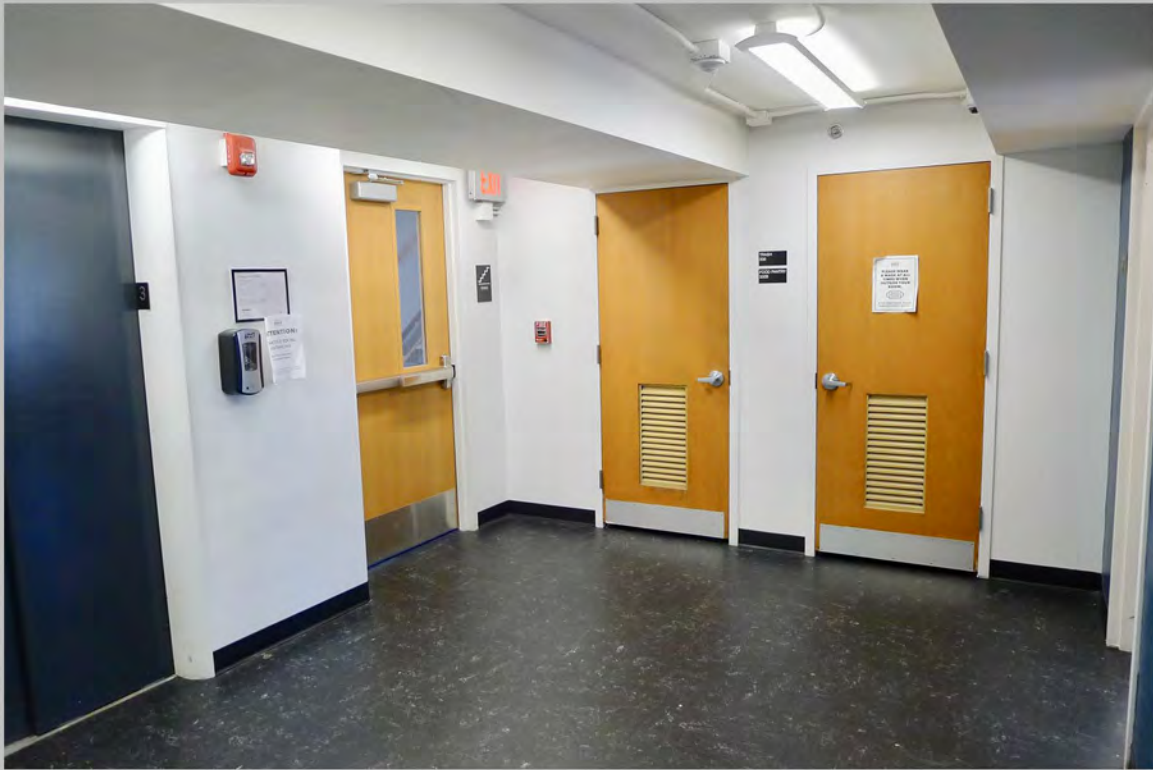
21. Third Floor - view southeast in elevator lobby
