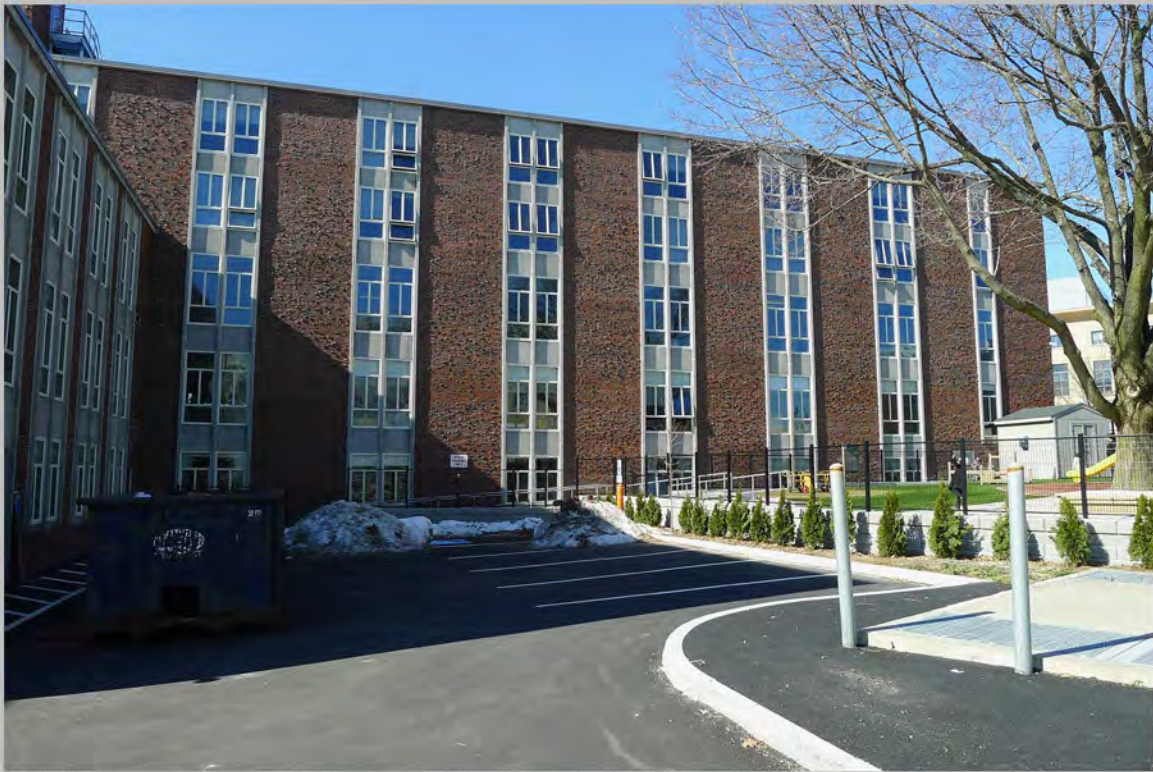
7. View southwest showing rear (northeast) elevation – detail of administrative/ residential wing
