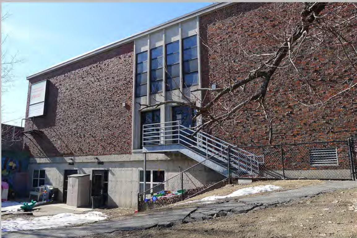
10. View south showing rear (northeast) elevation – detail of gymnasium wing
