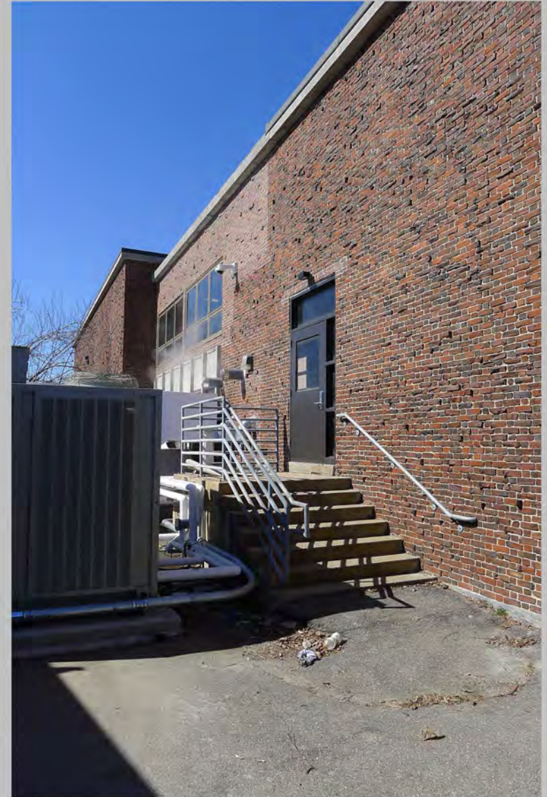
12. View northwest showing southeast elevation – entry to gymnasium wing
