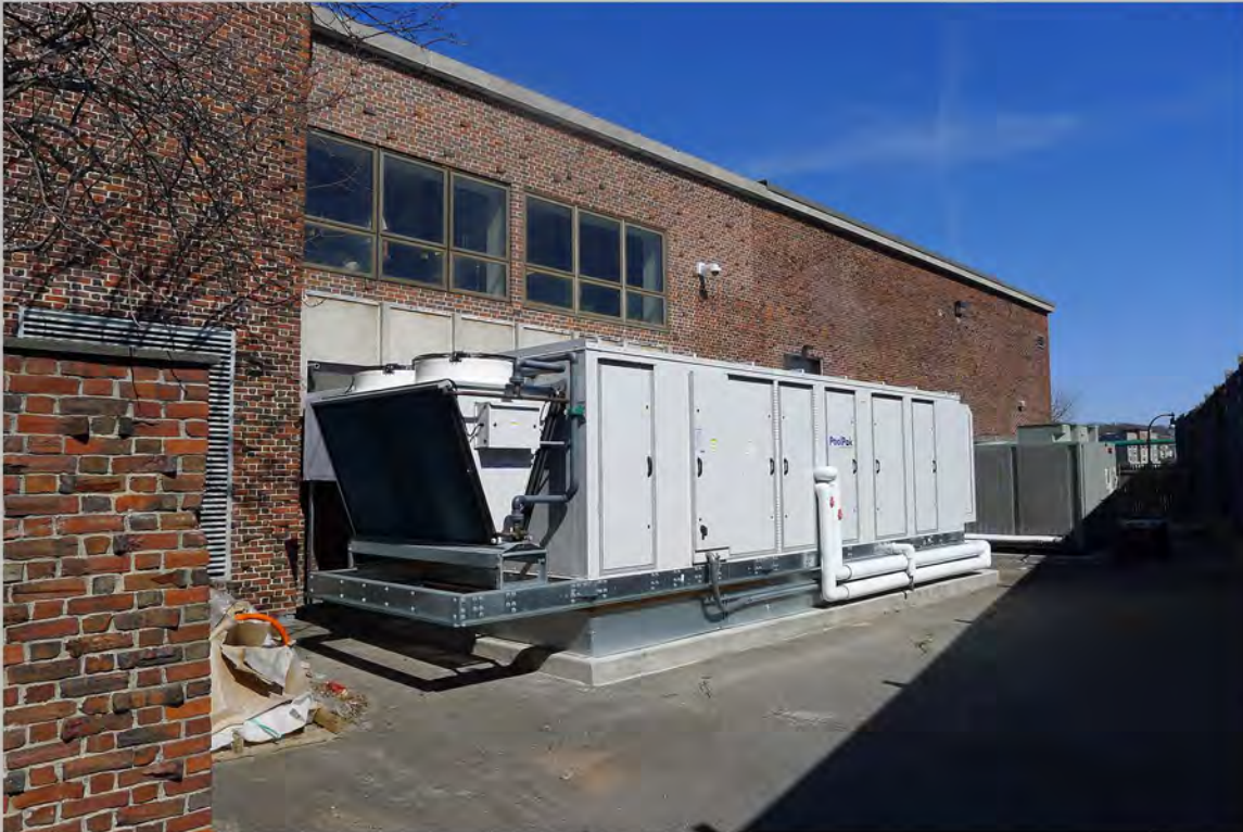
11. View northeast showing southeast elevation – detail of gymnasium wing
