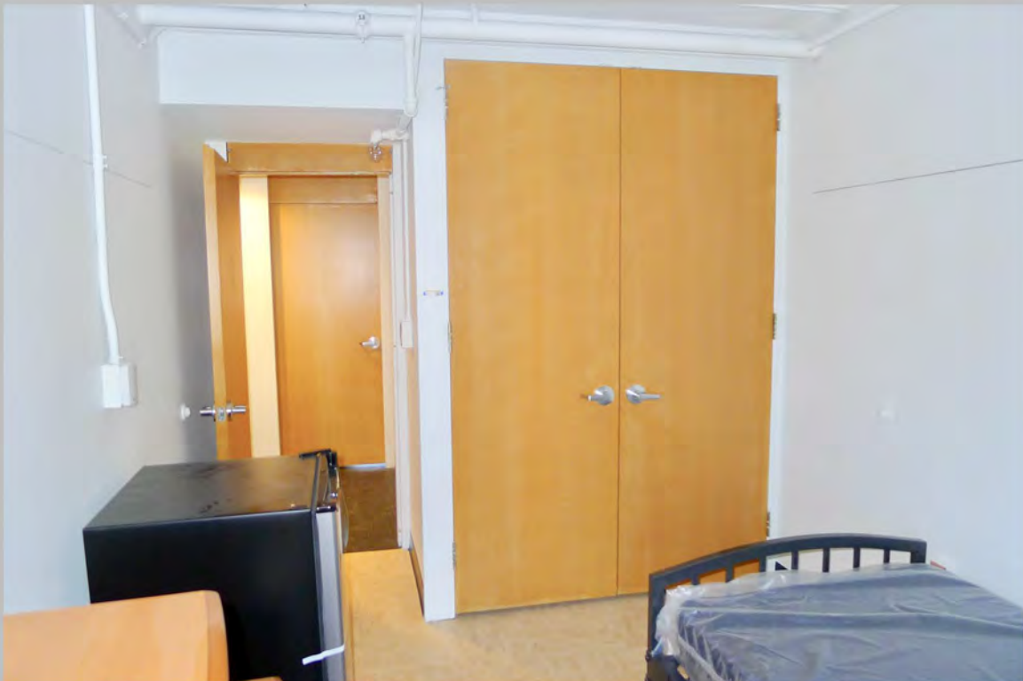
22. Third Floor – view southwest in typical residential room along northeast wall
