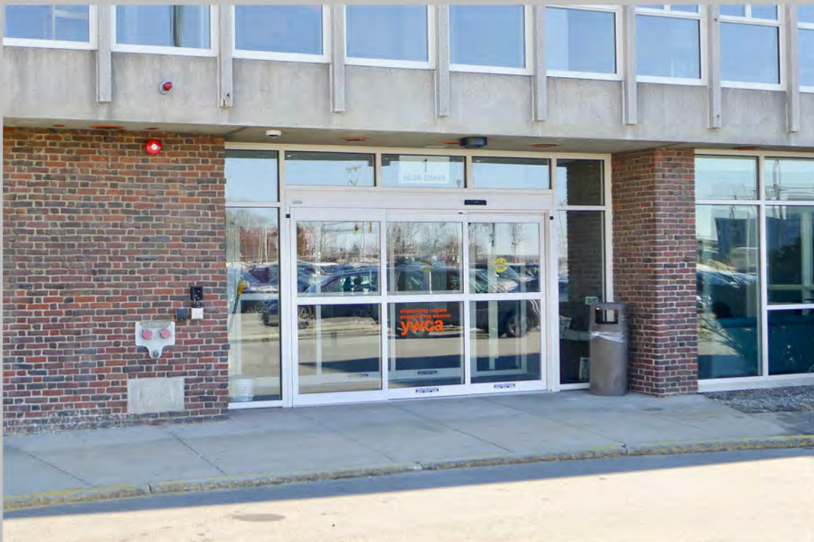
6. View northeast showing façade (southwest elevation) – detail of main entry
