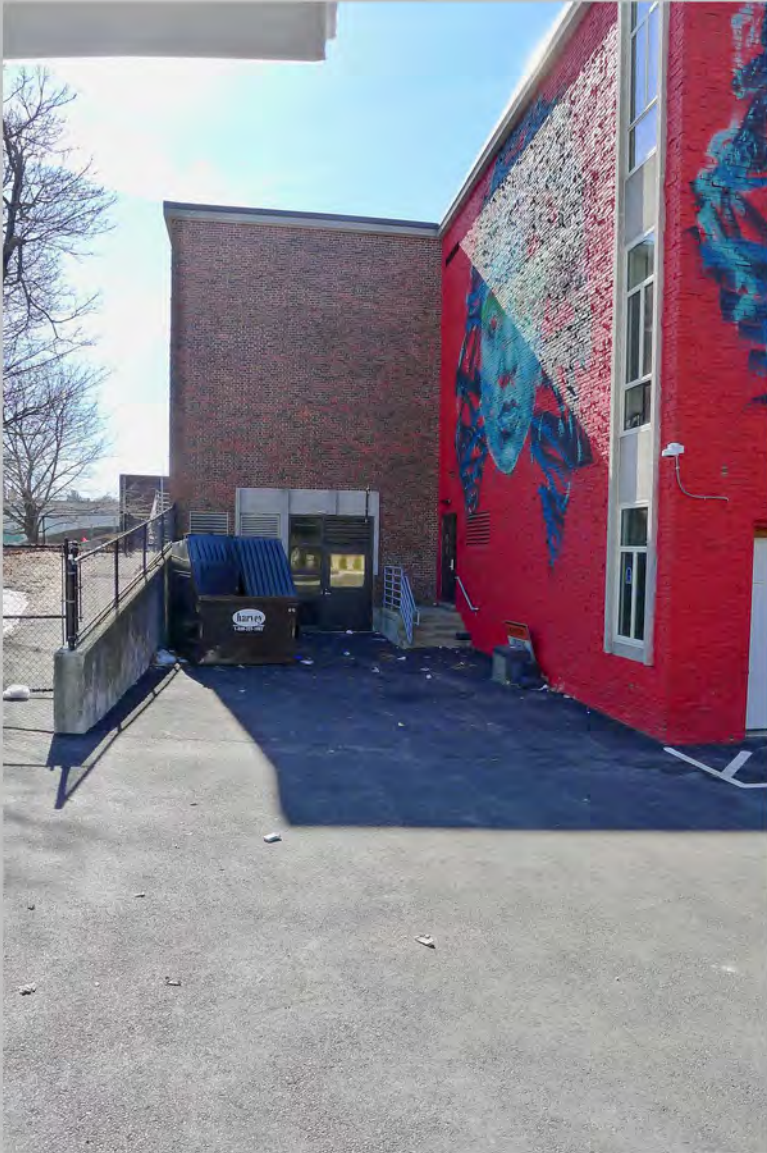
13. View southeast showing northwest elevation of gymnasium wing
