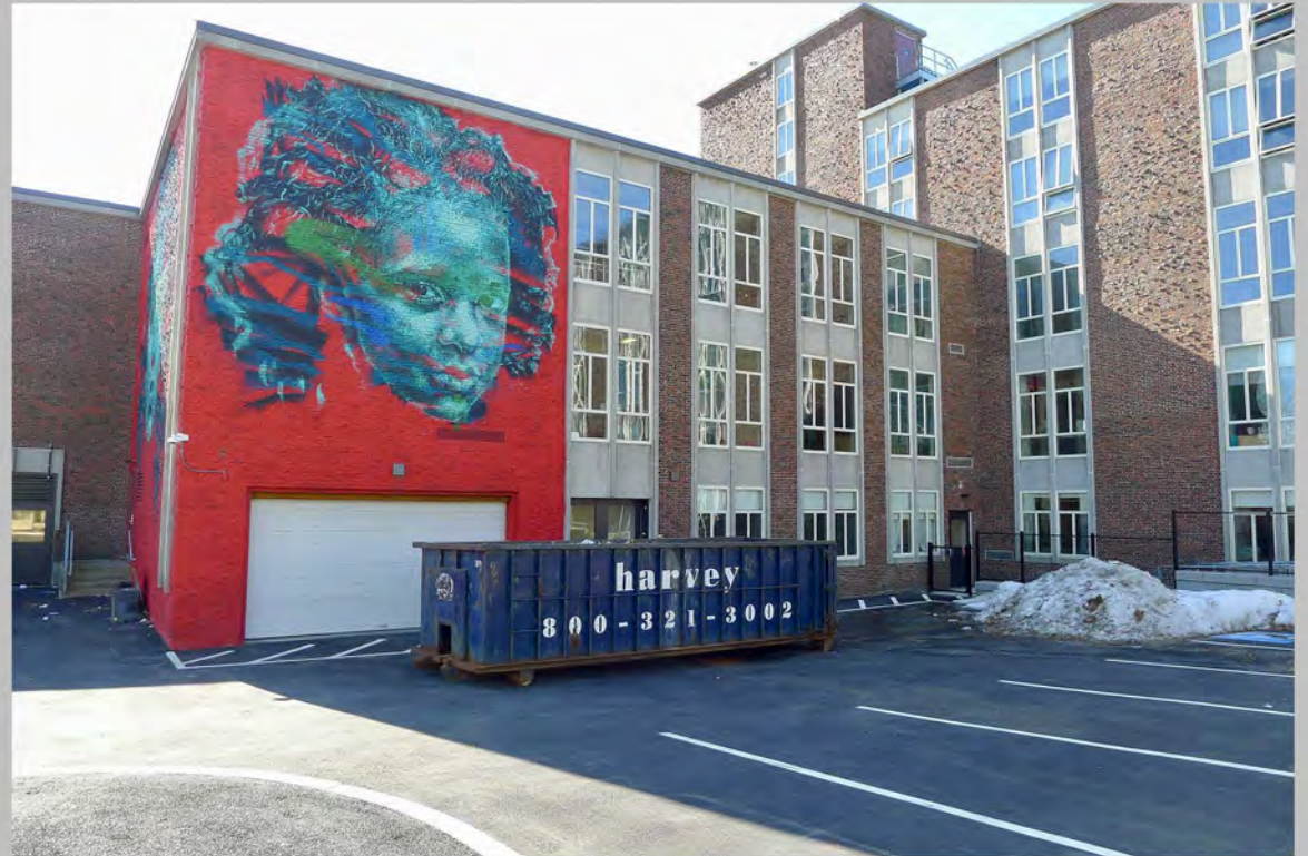
14. View southwest showing northwest elevation of service wing
