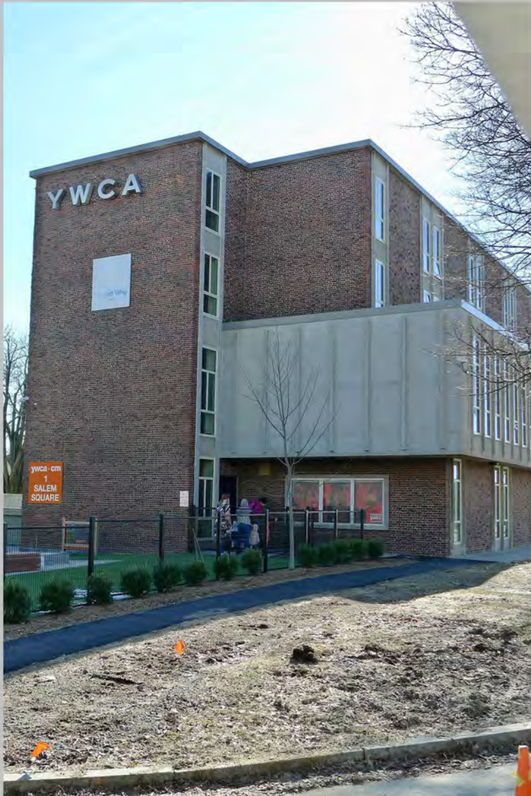
3. View southeast showing northwest elevation
