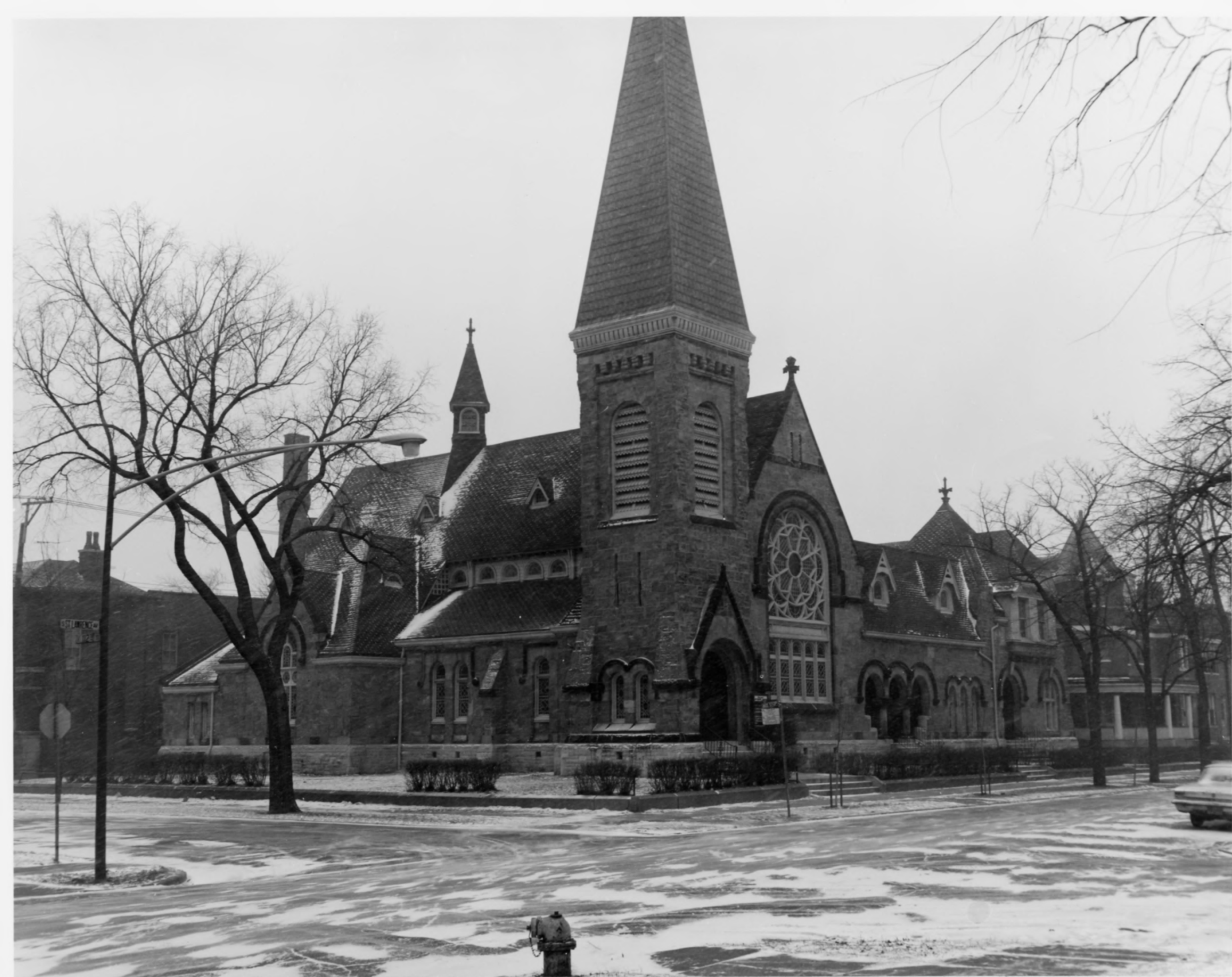
Greenstone Church - Pullman Historic District, Chicago, Illinois
