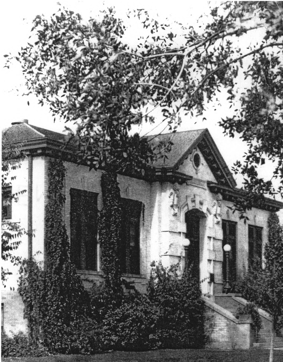
Sterling Public Library East elevation, view to the northwest Date: circa 1930 Source: Sterling Public Library
