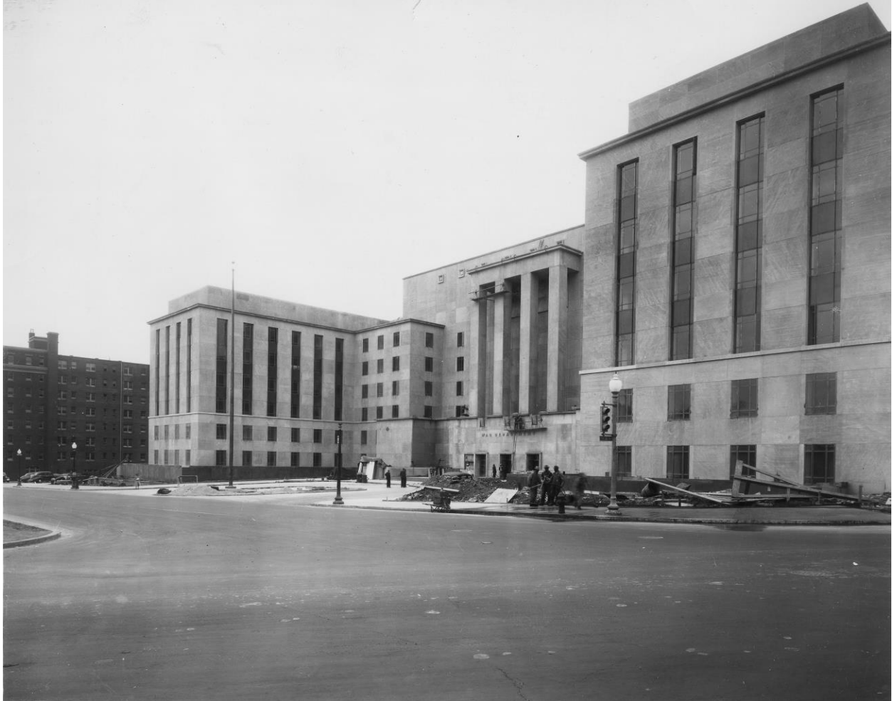
Figure 2 – U.S. Department of War Building, East Elevation, Looking Southwest, April 1941
