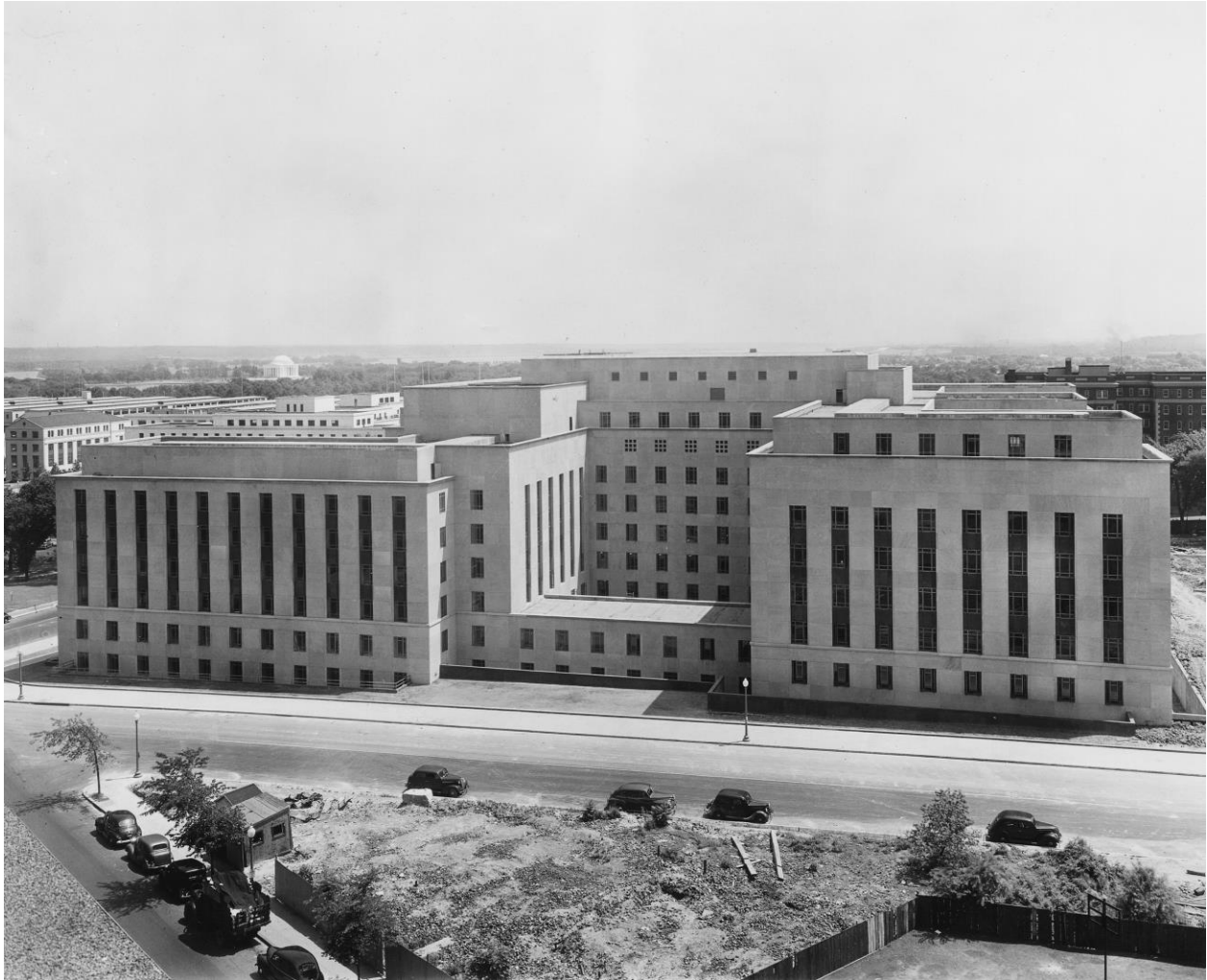
Figure 3 – U.S. Department of War Building, North Elevation, Looking Southeast, June 1941
