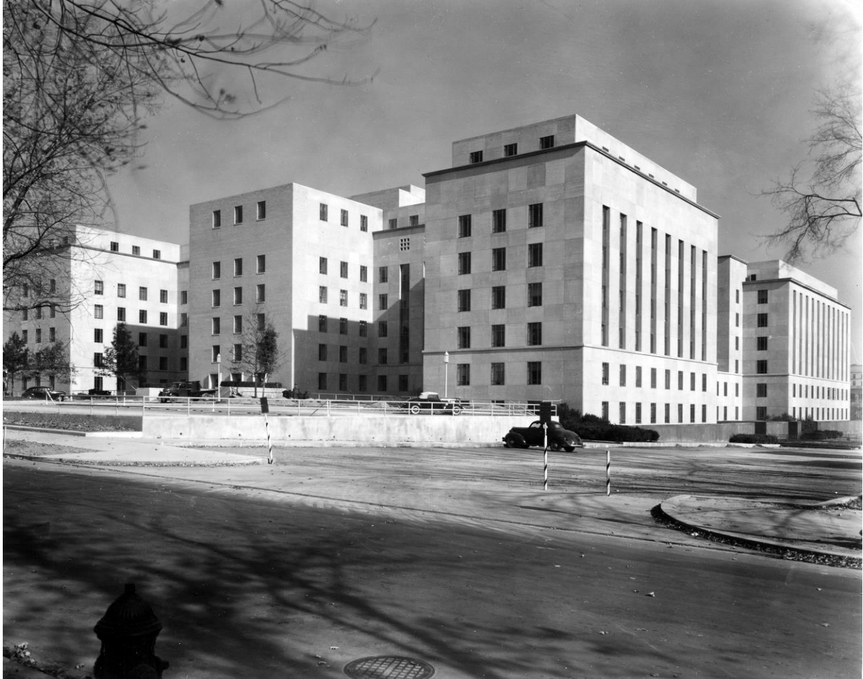
Figure 4 – U.S. Department of War Building, West and South Elevations, Looking Northeast, November 1941
