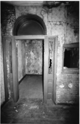
McBryen - Gutwood - Weber House Dawson County, TN
