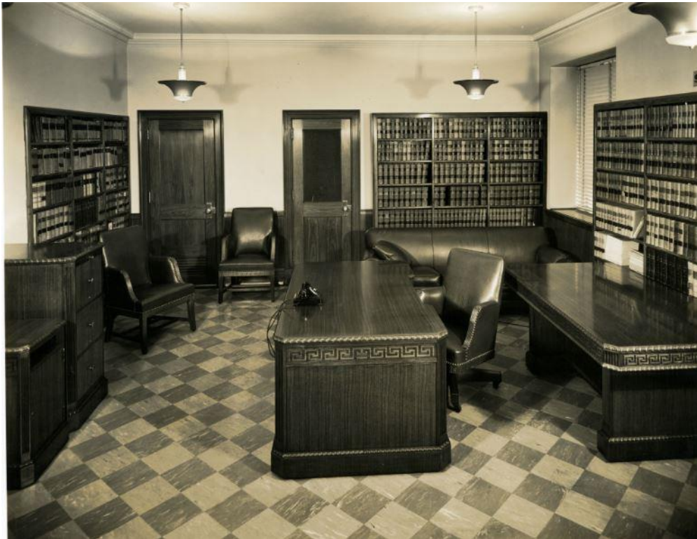
Figure 6. A Second Floor Office in 1938, this office is the same as office 319 in current photos 0064 and 0065. Note the original light fixtures which have been replaced with rectangular fluorescent lights, and the flooring which has been covered with carpet.
