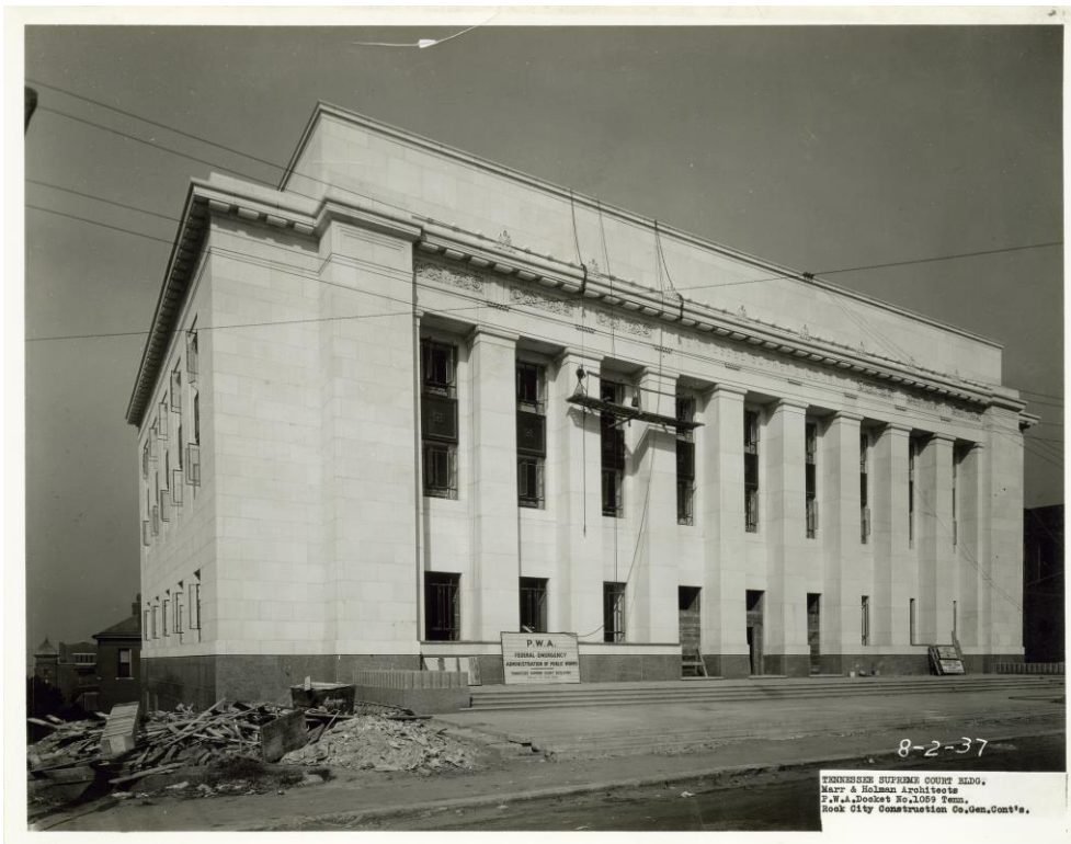
Figure 21. Construction progress August 2, 1937. (Courtesy of Rock City Construction and the Tennessee Supreme Court)
