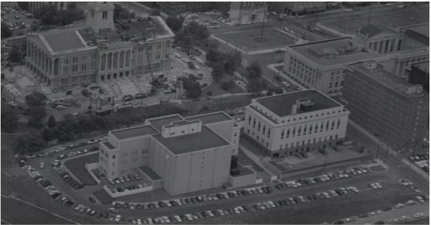
Figure 38. Aerial view of the Tennessee Supreme Court Building, July 1, 1957. (Photo courtesy of Nashville Public Library Digital Collections).
