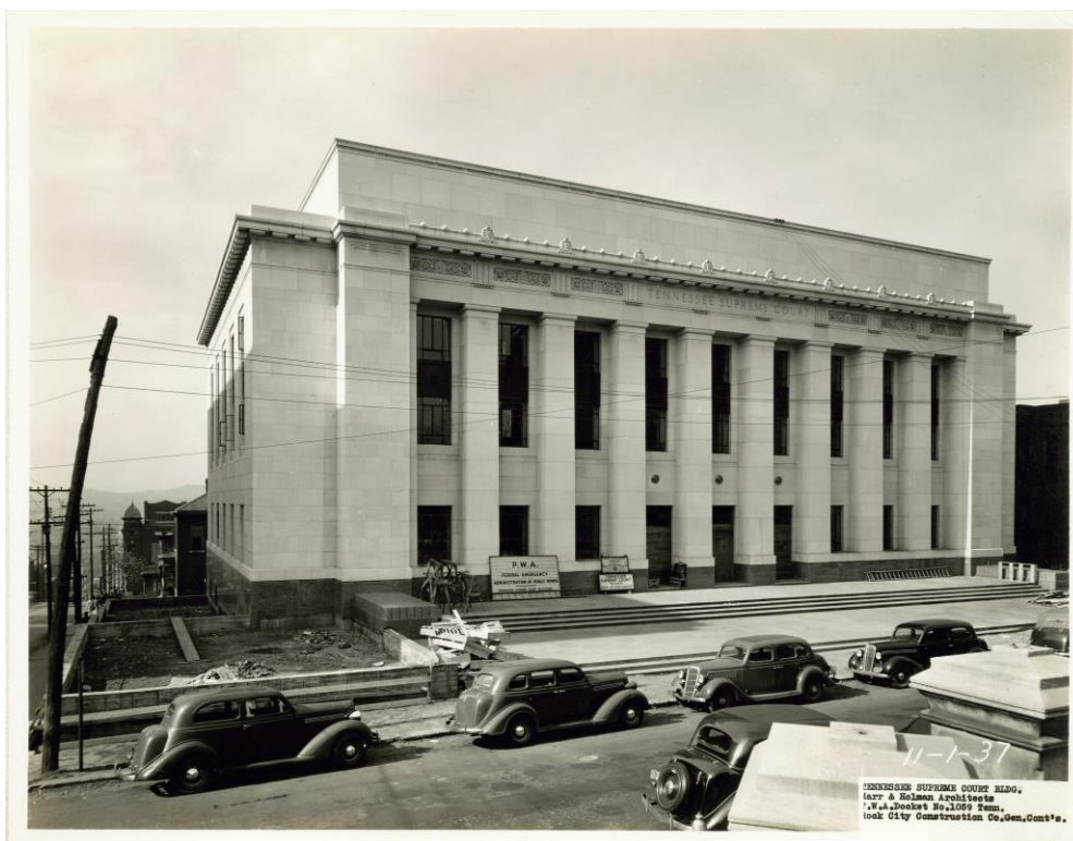
Figure 24. Construction progress November 1, 1937. (Courtesy of Rock City Construction and the Tennessee Supreme Court)
