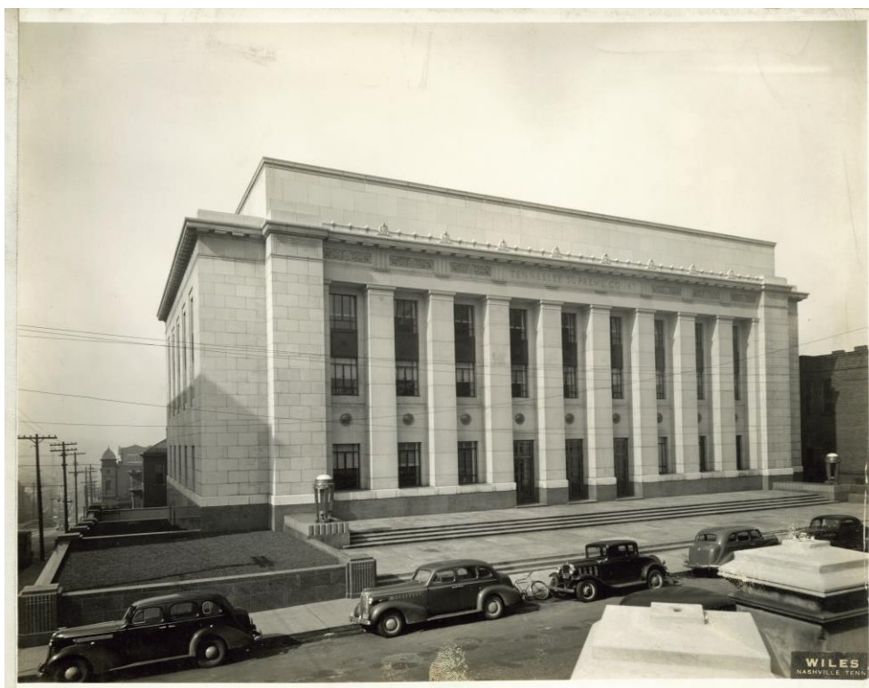
Figure 26. Building on February 1, 1938. (Courtesy of Rock City Construction and the Tennessee Supreme Court)
