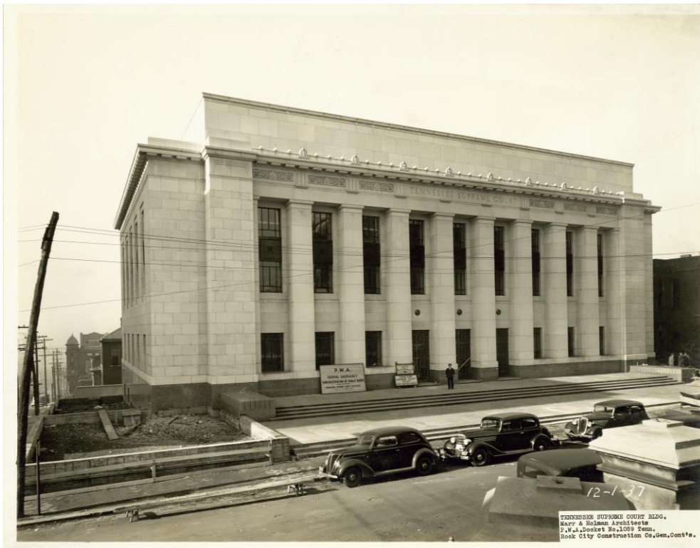
Figure 25. Construction progress December 1, 1937. (Courtesy of Rock City Construction and the Tennessee Supreme Court)
