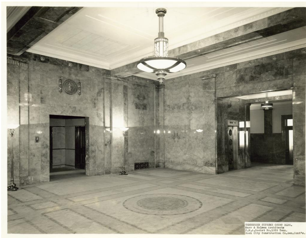
Figure 27. Lobby (Hall of Justice) on February 1, 1938. (Courtesy of Rock City Construction and the Tennessee Supreme Court)
