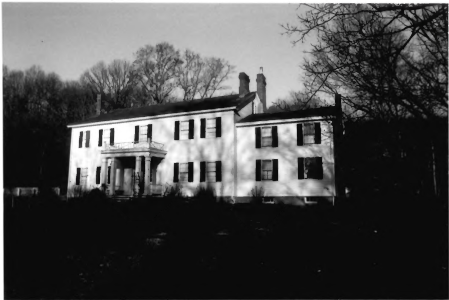
Binsmore House Boone Co., KY 1
