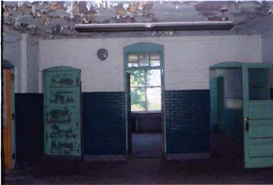
Historic Photograph #14: Looking west in second floor corridor, 2012.
