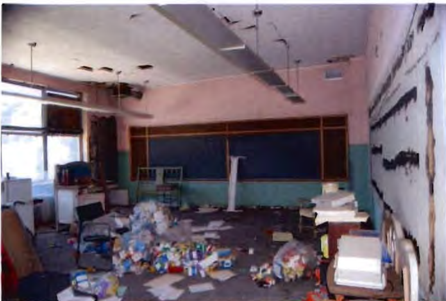
Historic Photograph #21: Typical second floor classroom in 1953 addition, 2012.
