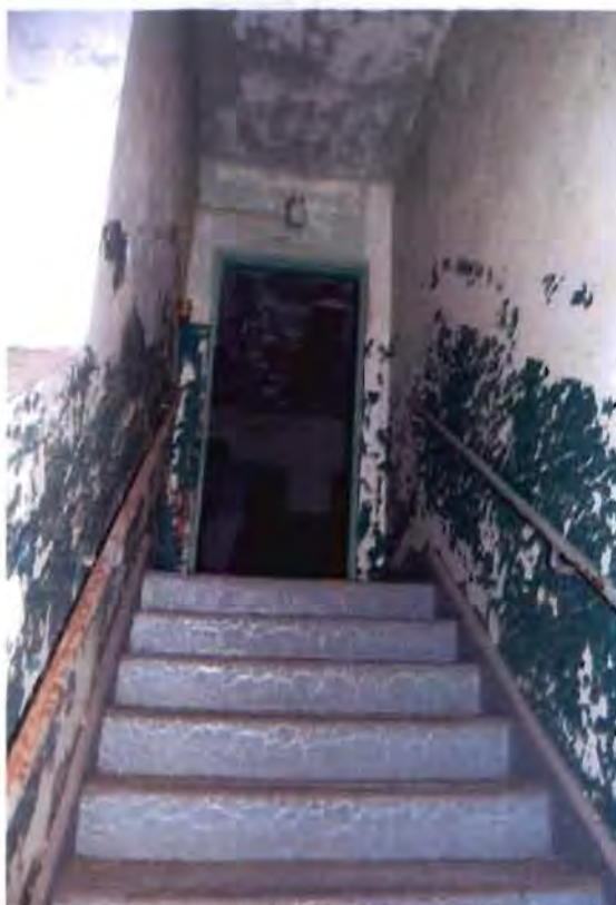
Historic Photograph #9: Looking north in south stair, typical stair condition, 2012.
