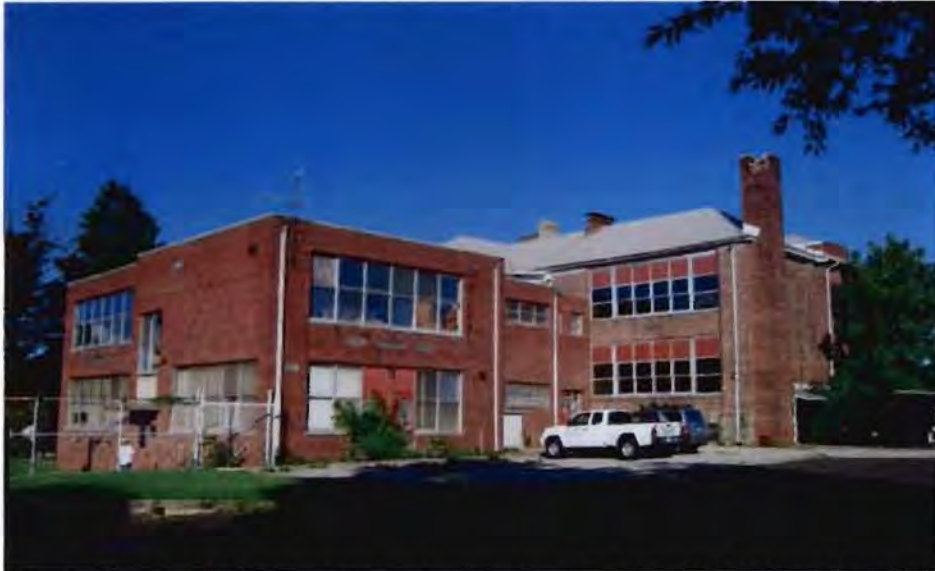
Historic Photograph #6: Looking northwest at rear (east) façade of 1922 addition (left) and rear (east) and south facades of 1953 addition (right), 2012.
