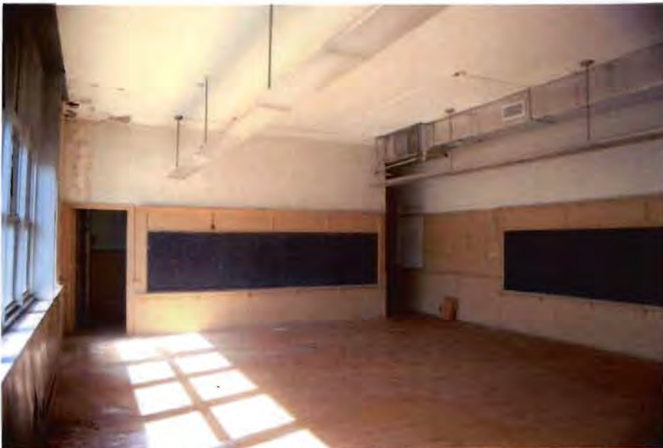
Historic Photograph #13: Typical first floor classroom in 1915 school and 1922 and 1925 additions, 2012.
