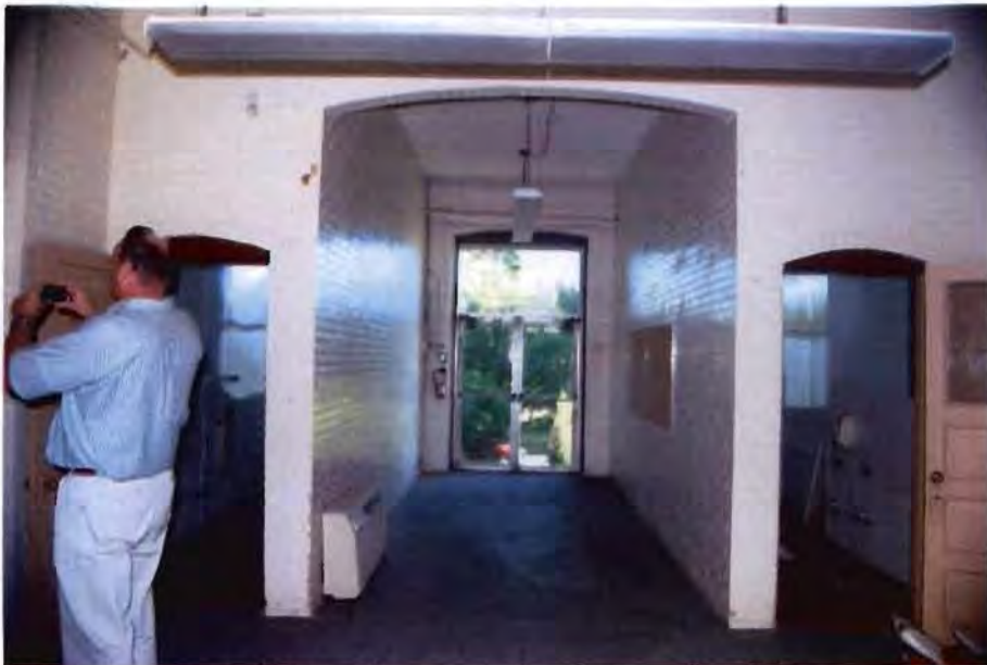
Historic Photograph #11: Looking west in first floor corridor, 2012.
