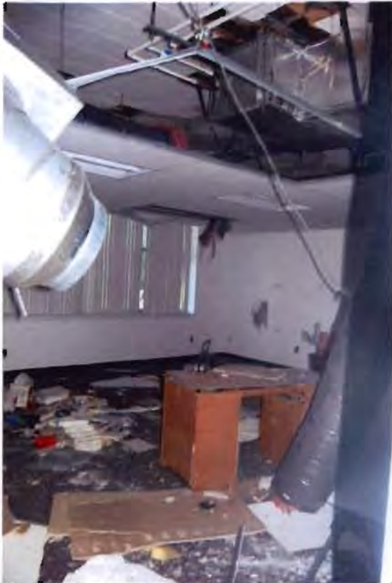
Historic Photograph #18: Typical first floor room in 1953 addition, 2012.
