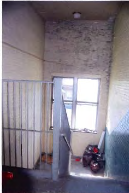
Historic Photograph #19: Southern stair tower in 1953 addition, 2012.
