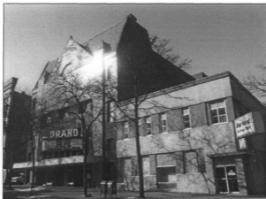
Figure 76: Grand theater, view to the northwest, c.1970
