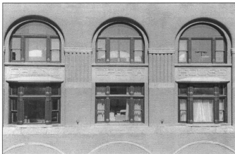
Figure 2: Façade detail (photo by James Jacobsen, August 2001)
