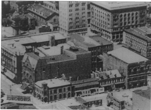
Figure 35: c.1912 bird's eye view to northwest (photo taken from the courthouse roof) Note the penthouse atop the Fly Gallery
