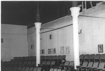
Figure 23: Balcony level and column supports for second balcony (photos by James Jacobsen, August 2001)
