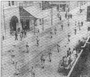
Figure 60: Parade in front of theater, note streetcar tracks on 8 th Street, view to the northeast. This image clearly shows the presence of a recessed foyer with no doorways set within the main arches.
