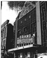
Figure 75: Full Metal Jacket, and the second marquee, 1964
