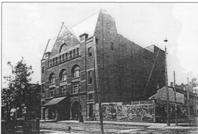
Figure 57: Grand and billboard corner lot, c. pre-1896. Note the frame building to the east later purchased by theater, view to the northwest. Note also commercial office lettering on right-hand second floor office window.
