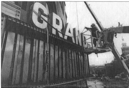
Figure 79: Marquee Removal, pre-1988
