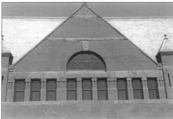
Figure 3: Façade detail (photo by James Jacobsen, August 2001)
