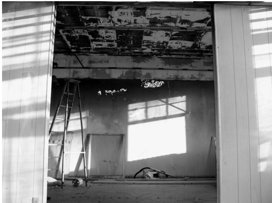
Figure J First Floor Interior. Classroom, 2012, looking into north section.
