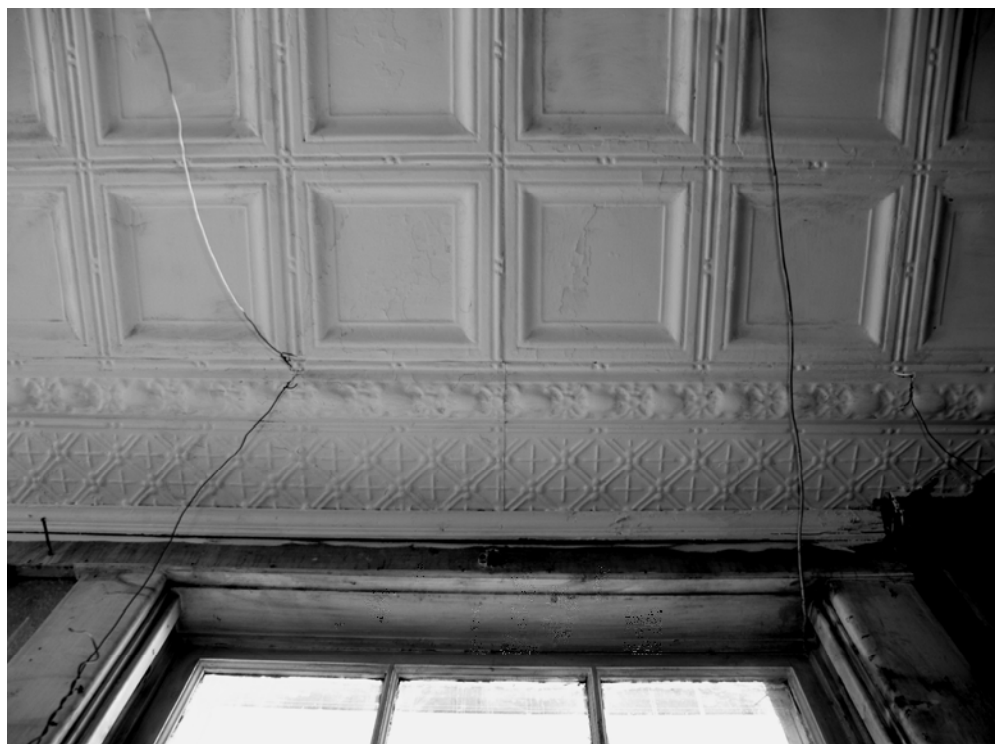
Figure K First Floor Interior. Detail of classroom ceiling, 2012.
