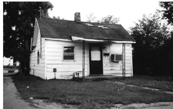
Figure T 415 West Fillmore Street, 2005.
