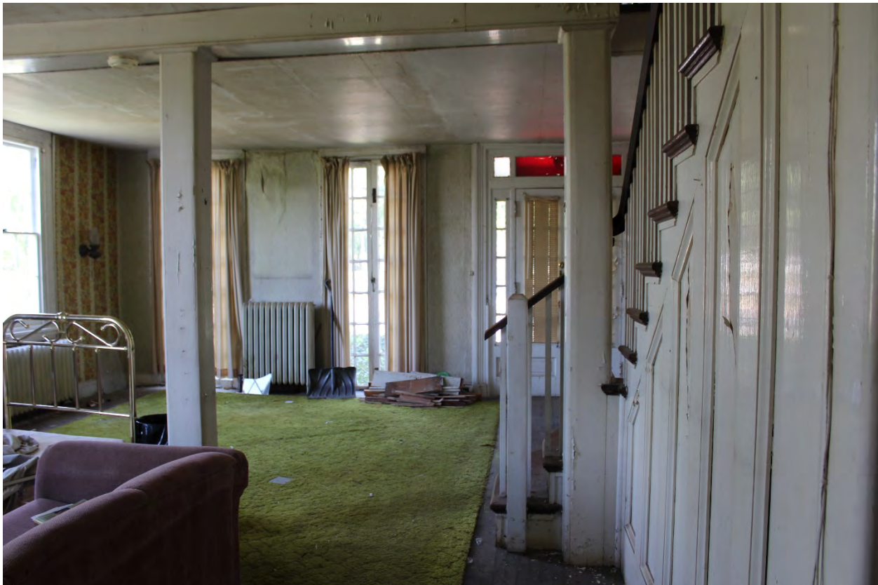
Photo 10: Room 101 looking west is a combination of original fabric (ca. 1852) including most of the stairs, the stair paneling, the doors and window trim with twentieth century upgrades including the narrow-gauge floors, the turn in the stair and the columns and ceiling beam added when an original partition was removed
