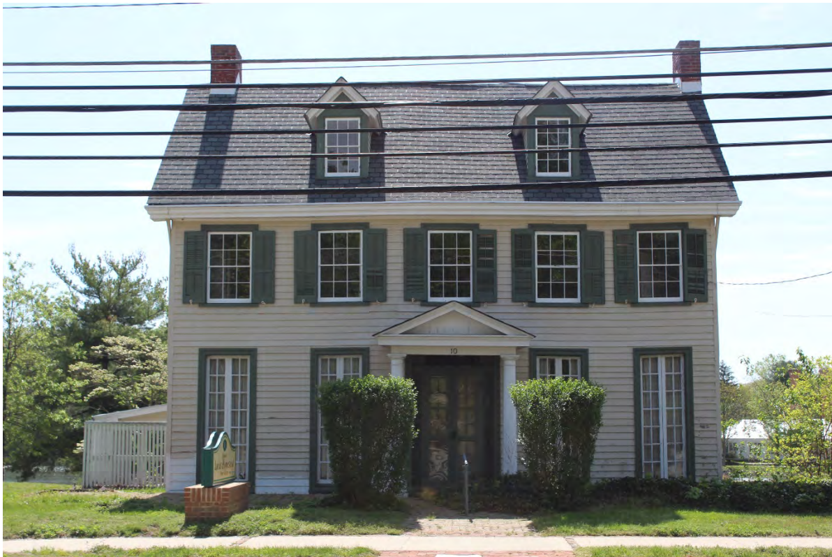
Photo 5: The west façade represents two phases of construction. The south (right) three bays are original ca. 1852 while the two north bays followed ca. 1856. The Colonial Revival entrance porch was added in the twentieth century
