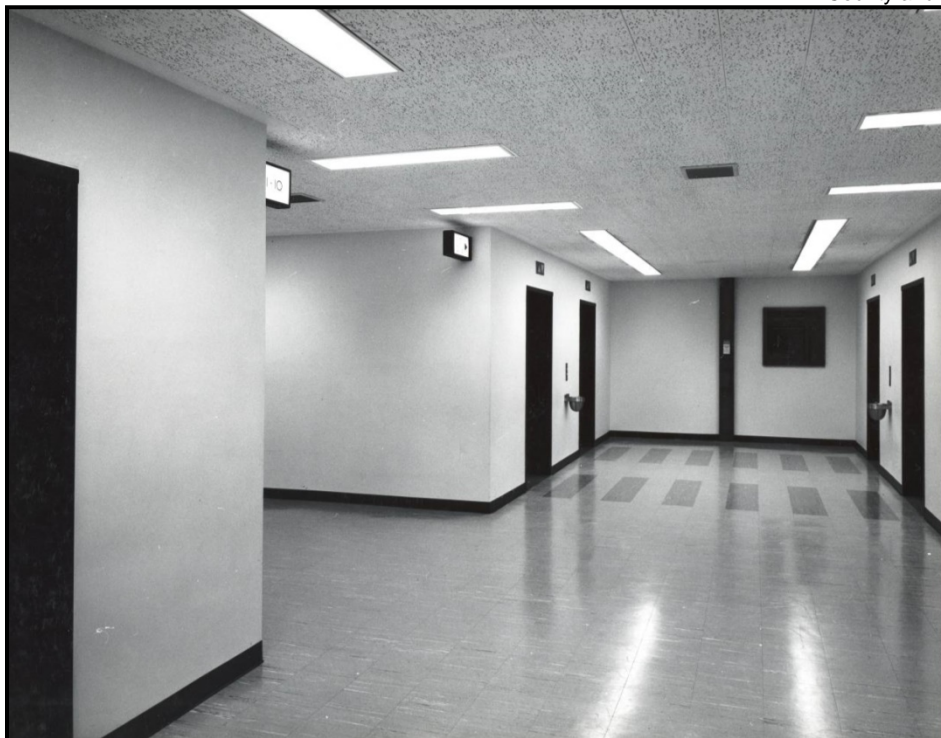
H27. February 2, 1966, photograph of the second floor elevator lobby of the Federal Building.
