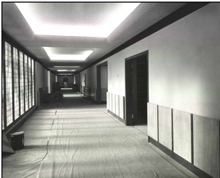
H13. December 1, 1964, photograph of fourth-floor corridor in the U.S. Courthouse.
