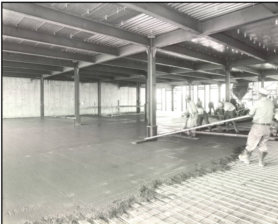
H10. September 3, 1963, photograph of seventeenth floor concrete floor being poured.
