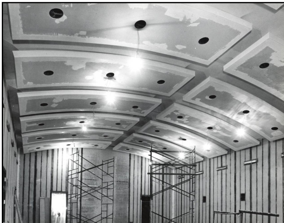
H11. April 1, 1964, photograph of courtroom ceiling construction, U.S. Courthouse.
