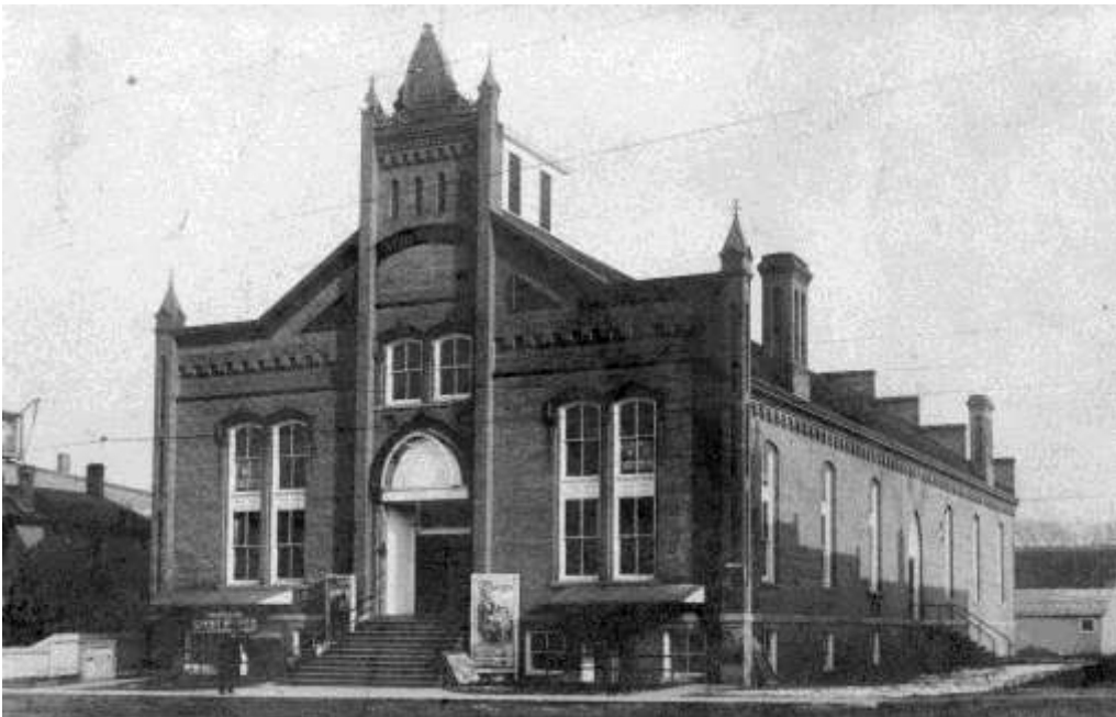
Figure # 13 - Apollo Hall, 455 S. Main St.; photo before 1931 remodeling and conversion to movie theater (photo date unknown).
