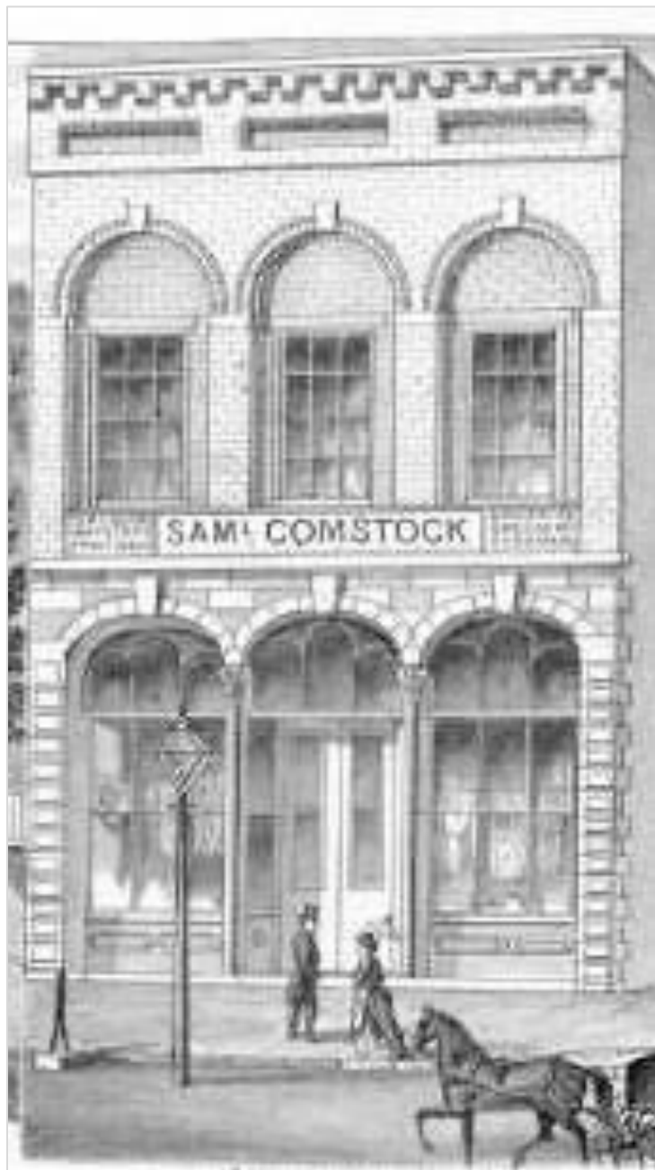
Figure 8. Comstock Building, 2091 Front Street (#31), Historic Image 1874
