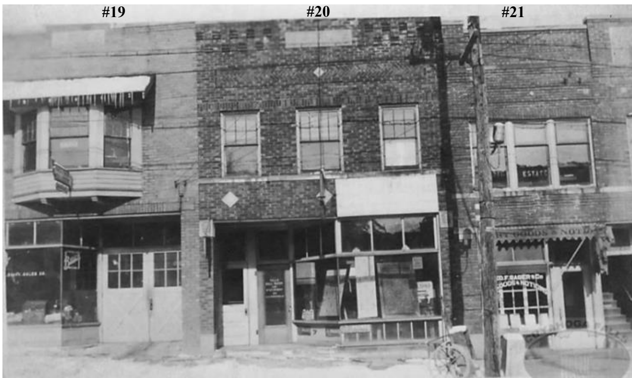
Figure 14. North side Portage Trail, Photo undated 1915 Fox Building, 123 Portage Trail (#19); 1915 Smith Building, 119 Portage Trail (#20); and, 1915 Hedden Building, 111 Portage Trail (#21),
