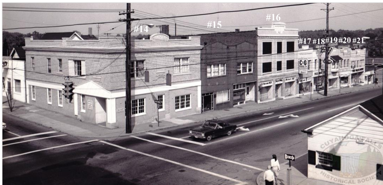
Figure 18. Portage Trail, Intersection with 2 nd Street, facing northeast, Photo 1967 1915 Hachtel Building, 149 Portage Trail (#14); 1916,1926 Bauman Block, 139-143 Portage Trail (#15); 1916 I.O.O.F. Building,133-137 Portage Trail (#16); 1918 Snook Building, 129 Portage Trail (#17); 1918 Porter Building, 127 Portage Trail (#18), 1915 Fox Building, 123 Portage Trail (#19); 1915 Smith Building, 119 Portage Trail (#20); and, 1915 Hedden Building, 111 Portage Trail (#21),
