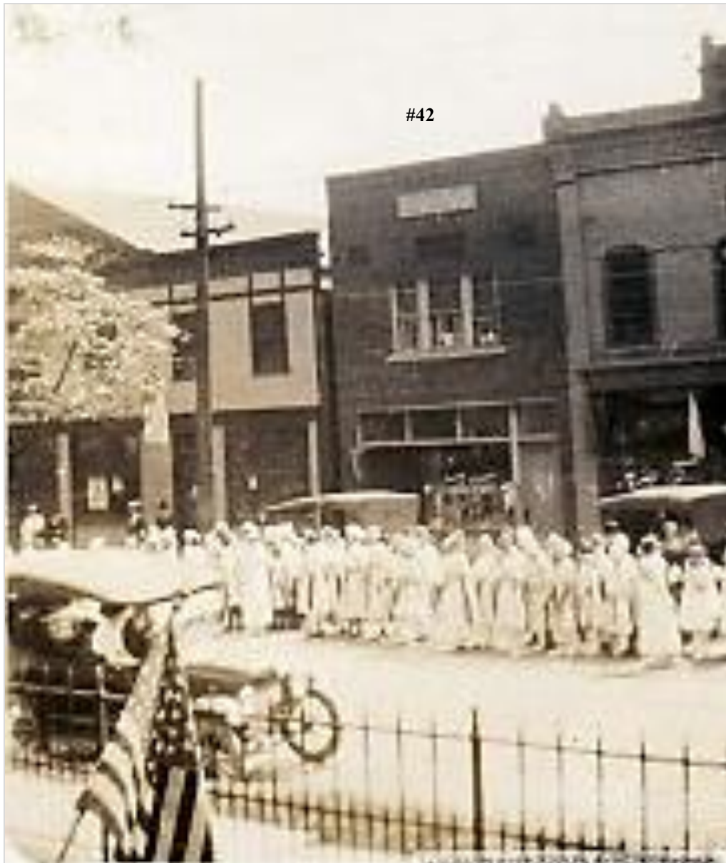
Figure 11. ca. 1900 Kanecky Building, 2241 Front Street (#42), Photo ca. 1912
