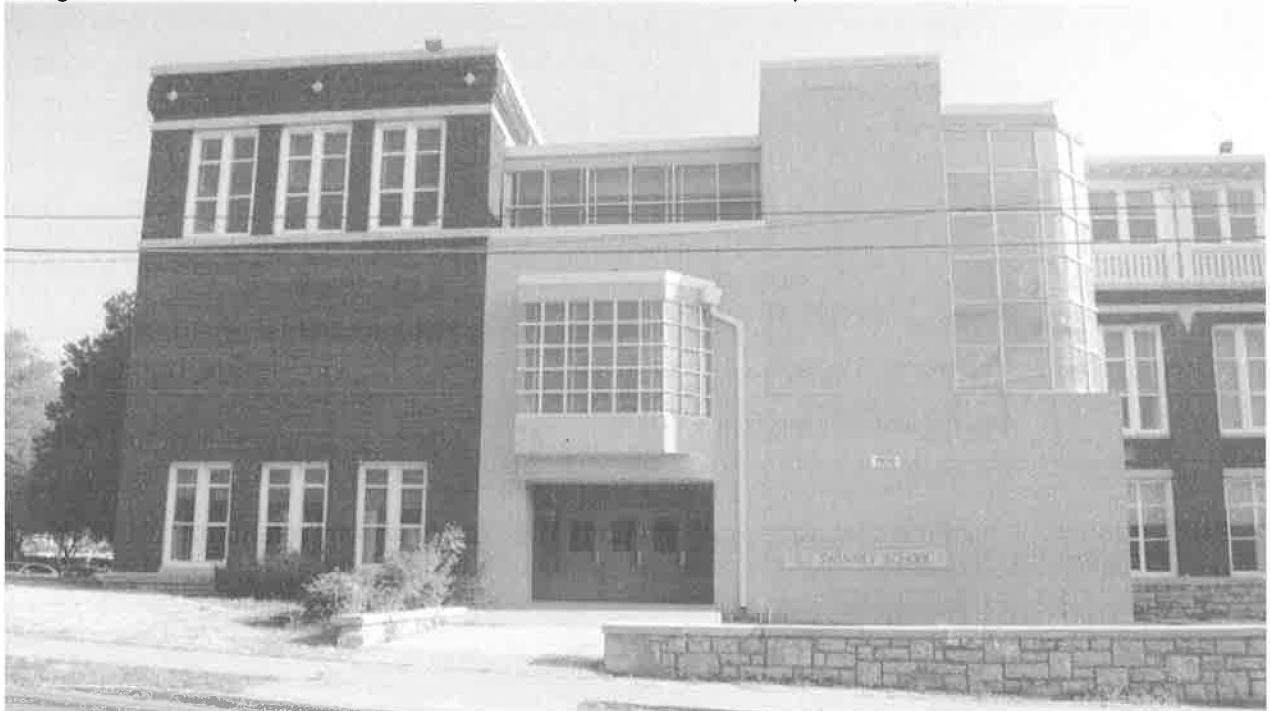
Figure 19. South elevation with the 1987 circulation tower prior to removal, view north. 2012.
