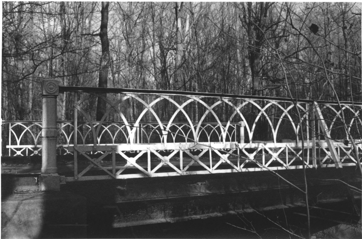
COMBS HOLLOW RD. BRIDGE, COMBS HOLLOW HISTORIC DISTRICT 034/027
