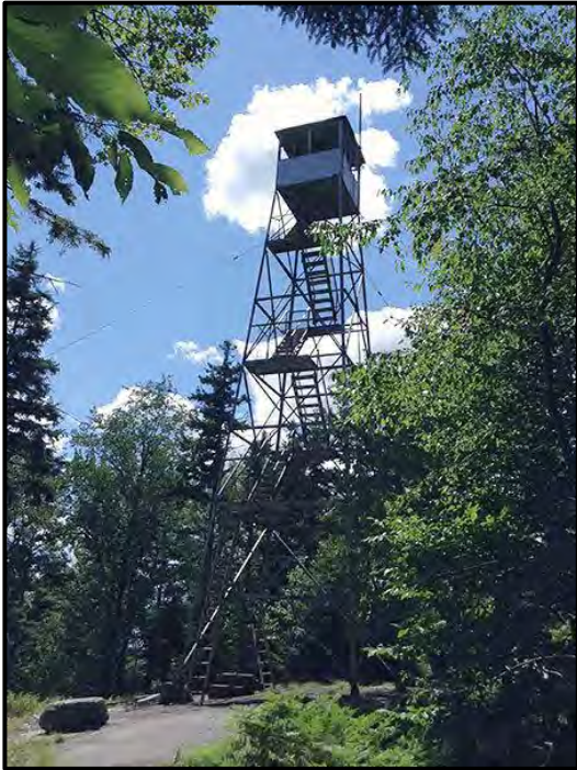
Figure 4. Stillwater Mountain Fire Observation Tower, 2016 (Jim Fox).
