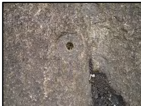
Figure 2. Remains of eyebolt (secured with metal plug) used to steady a short signal tower for the Adirondack Survey of 1882.
