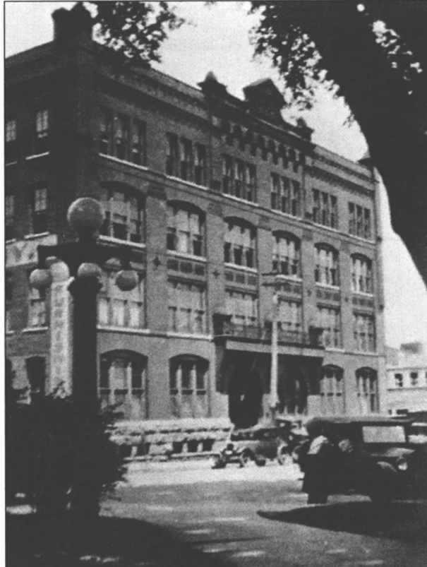
Figure 14: Rider-Wallis south façade, looking northeast from Washington Park (Loras College, Center for Dubuque History, Photo NGL-1673)
