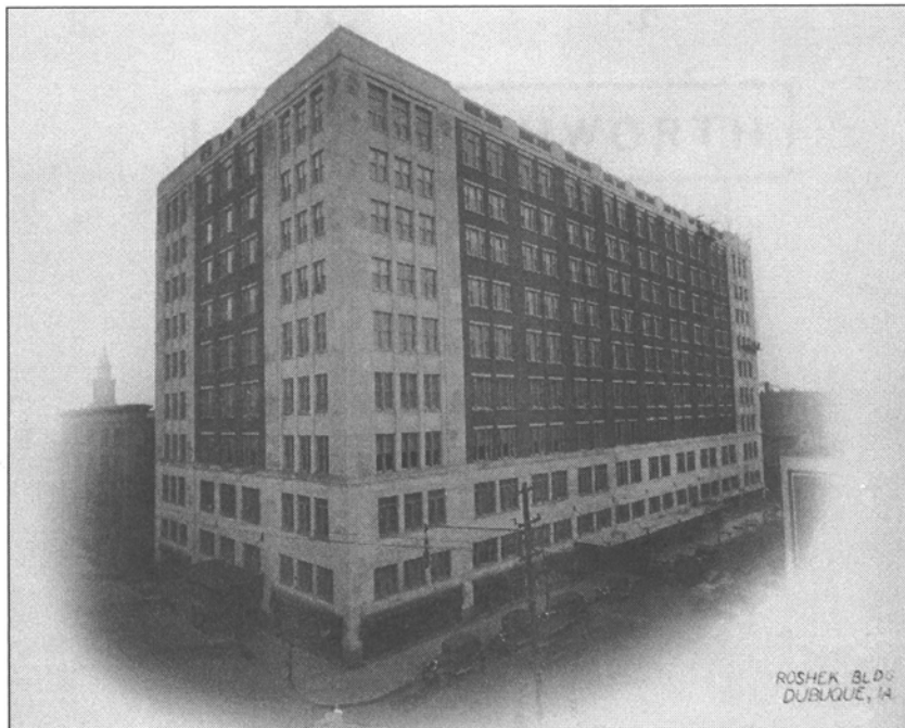
Figure 32: Construction completion photo, view southeast, 1931
