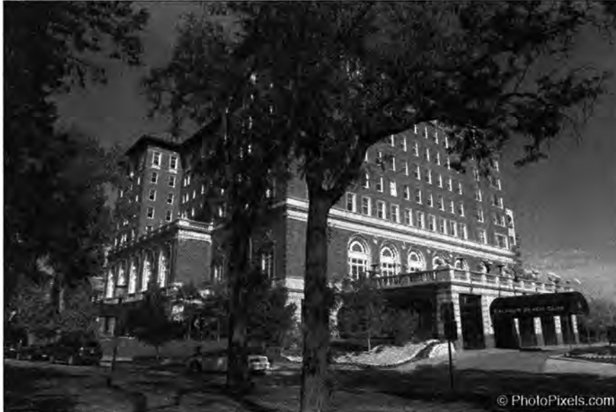
Figure 45: Vintage Apartments, Dean Parkway and West Lake Street, Minneapolis, Nicol was not the principal designer, nine stories, 1929, completed 1946 ( www.photopixels.com/cbc/pages )
