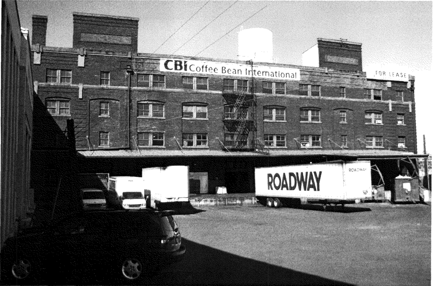
Photo 4 of 23: Southwest façade. View to NE.
