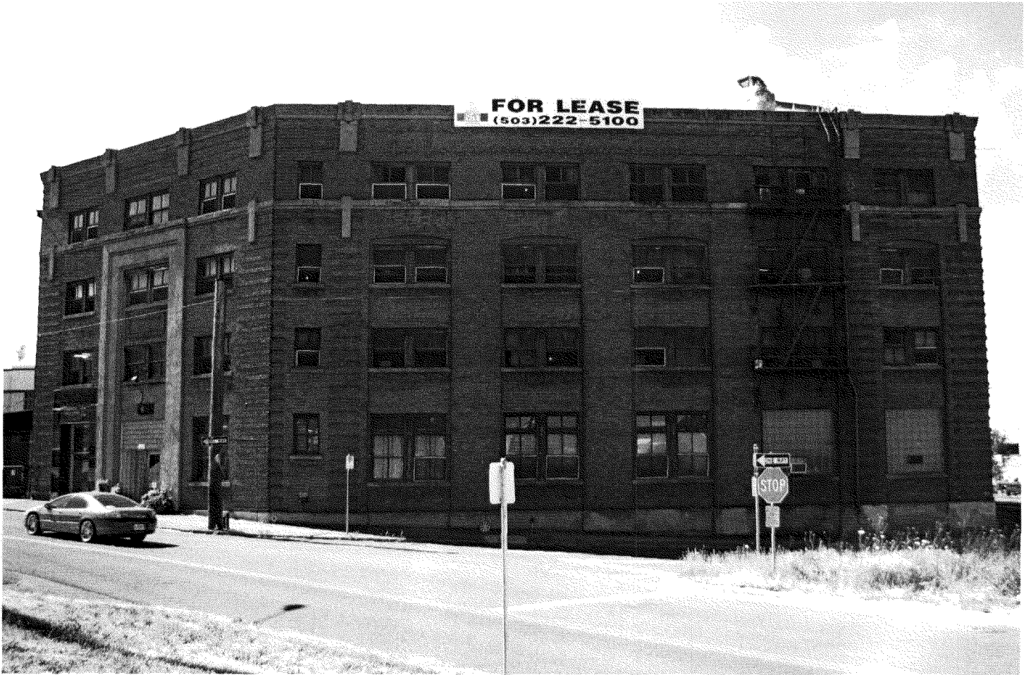
Photo 3 of 23: South façade and southeast façade. View to NW.
