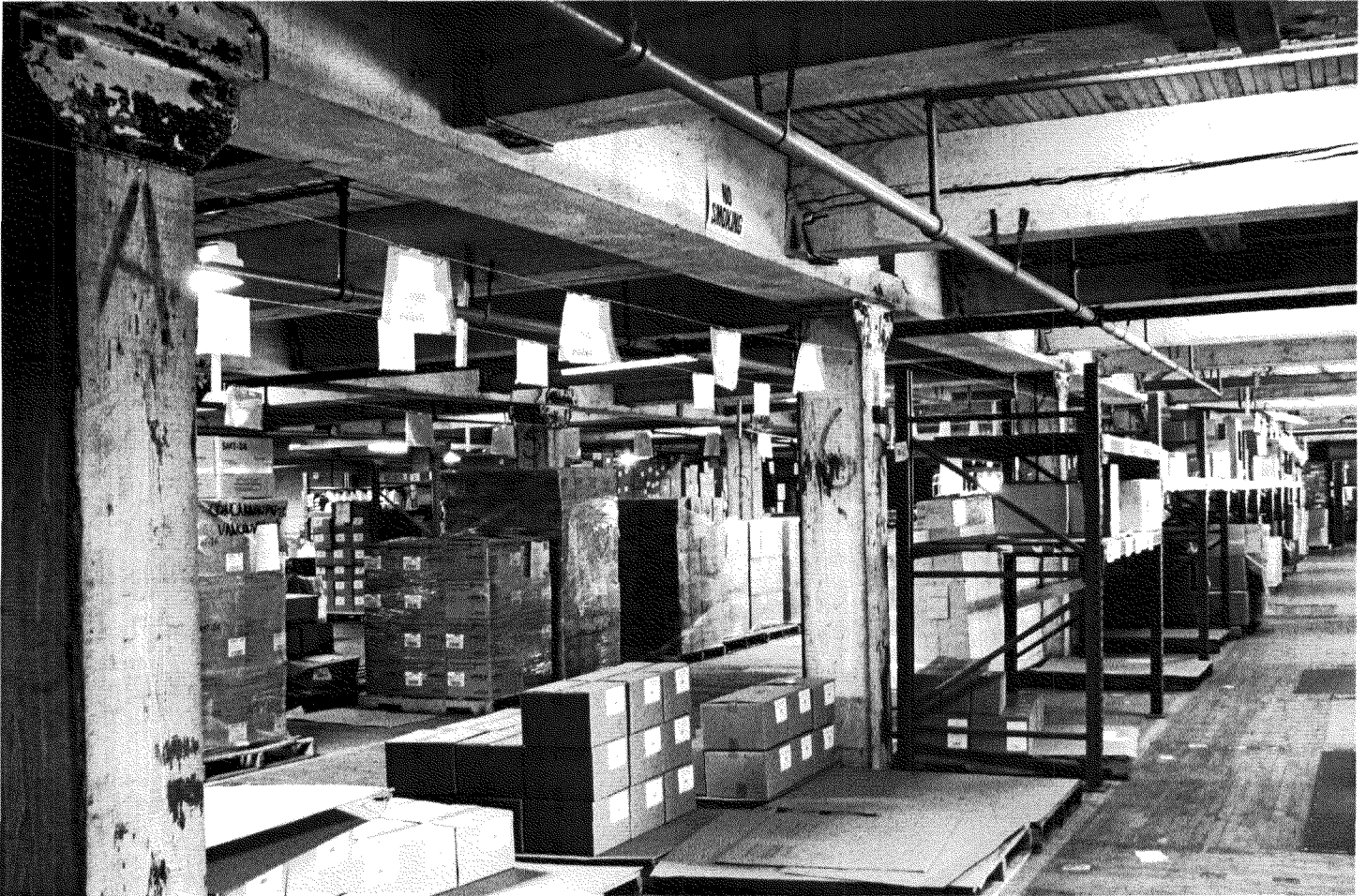
Photo 19 of 23: Third floor: warehouse View to W.
