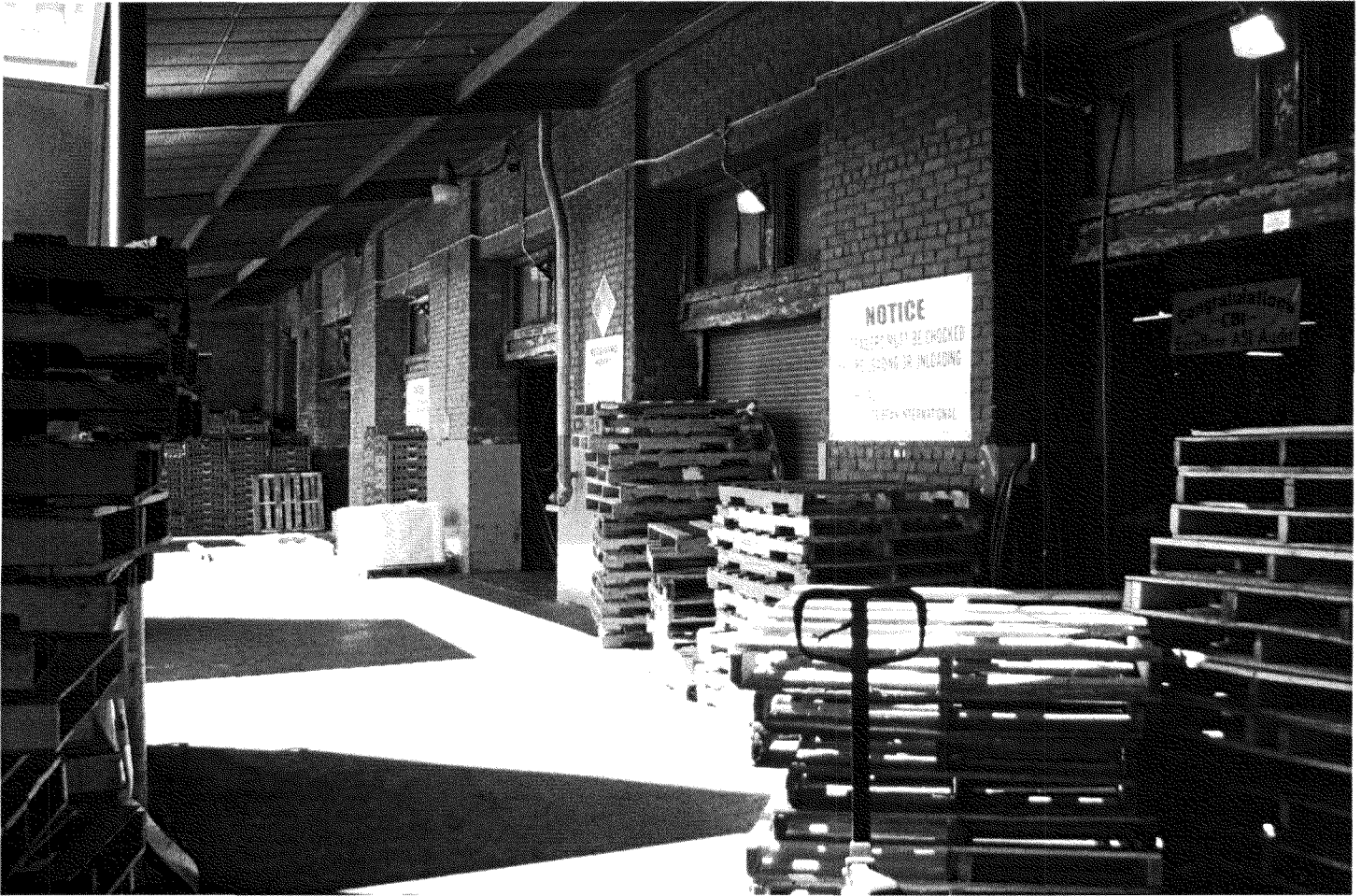
Photo 8 of 23: Southwest façade: loading dock. View to NW.
