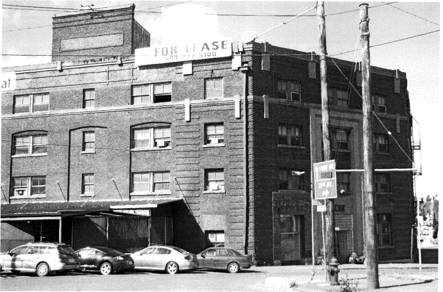
Photo 2 of 23: South and southwest façade. View to N.
