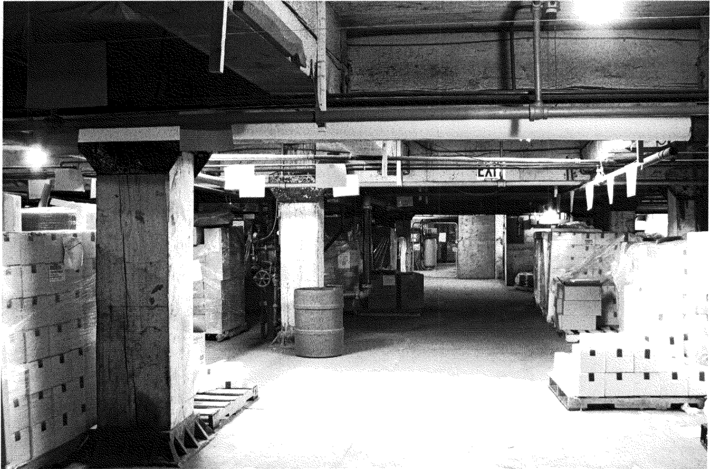
Photo 21 of 23: Basement: warehouse. View to SW
