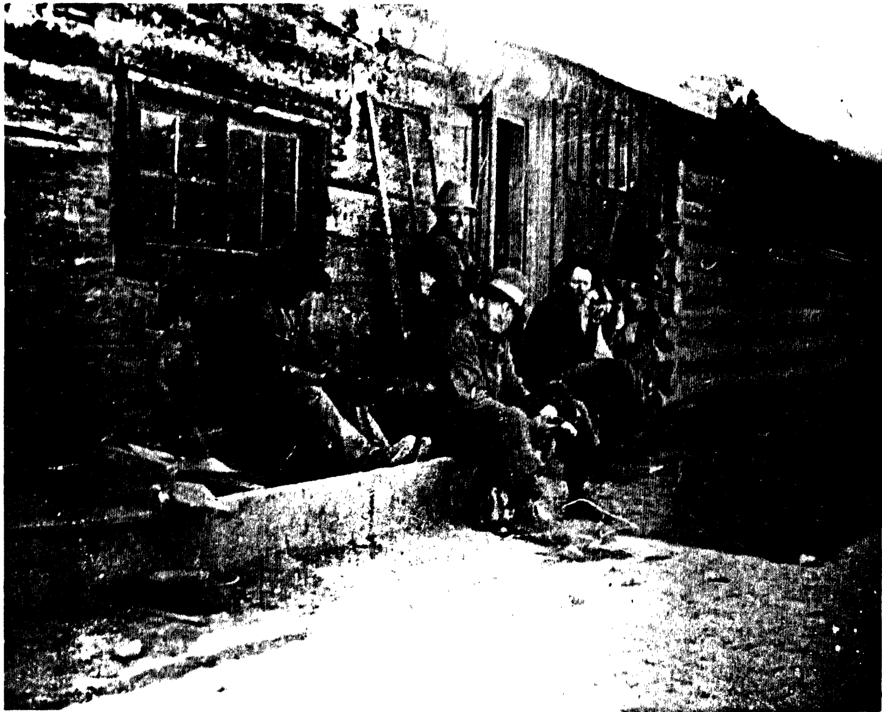
20... Bunkhouse with crew, to NE (west and center cabins)
