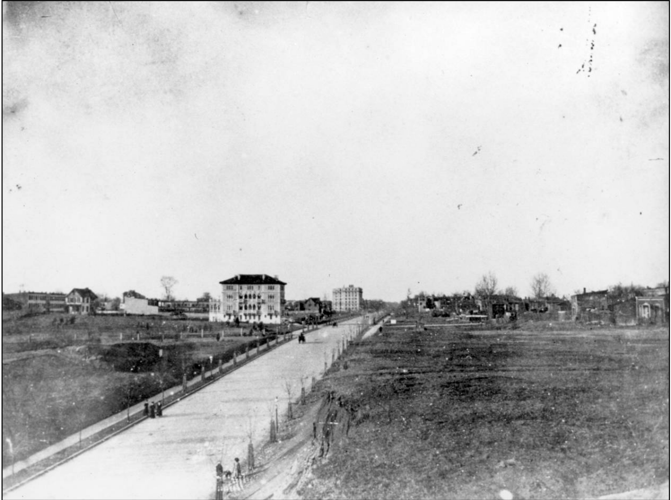
View Looking north on Sixteenth Street from east side of street south of Euclid Street at site of Meridian Hill Park, circa 1906, and showing the Venetian (Pink) Palace (1905) in center and the Kenesaw Apartments (1905) at center background. (Courtesy Historical Society of Washington CHS 08001)
