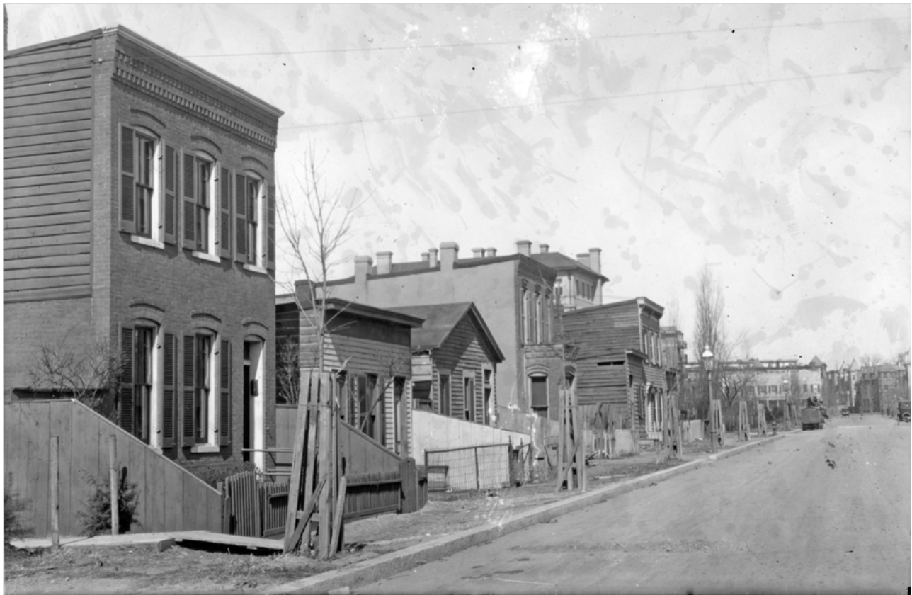
Houses on 15 th Street (Columbia Avenue on plat) in the Meridian Hill Subdivision prior to demolition in 1915. The MacVeagh House (later Embassy of Mexico), built 1910, is visible at the center of photo rising above and behind the still extant frame houses. (Courtesy of Historical Society of Washington CHS 5203)
