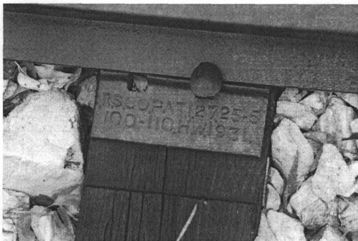
Figure 2: Tie plate, tie, rail and ballast
