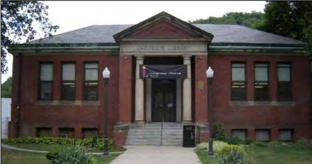
Figure 13: West End Branch Library (1899), Pittsburgh, Pennsylvania. Image from Google Streetview.
