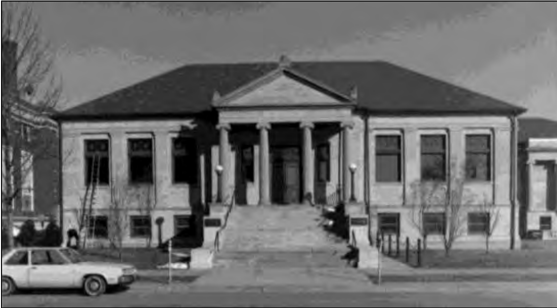
Figure 11: Kellogg Public Library, Green Bay, WI. Designed by Henry A. Foeller in 1901, Completed 1903. 1987 photograph included in the Wisconsin Historic Preservation Database (WHPD), Available online at www.wisconsinhistory.org , Accessed October 2016.
