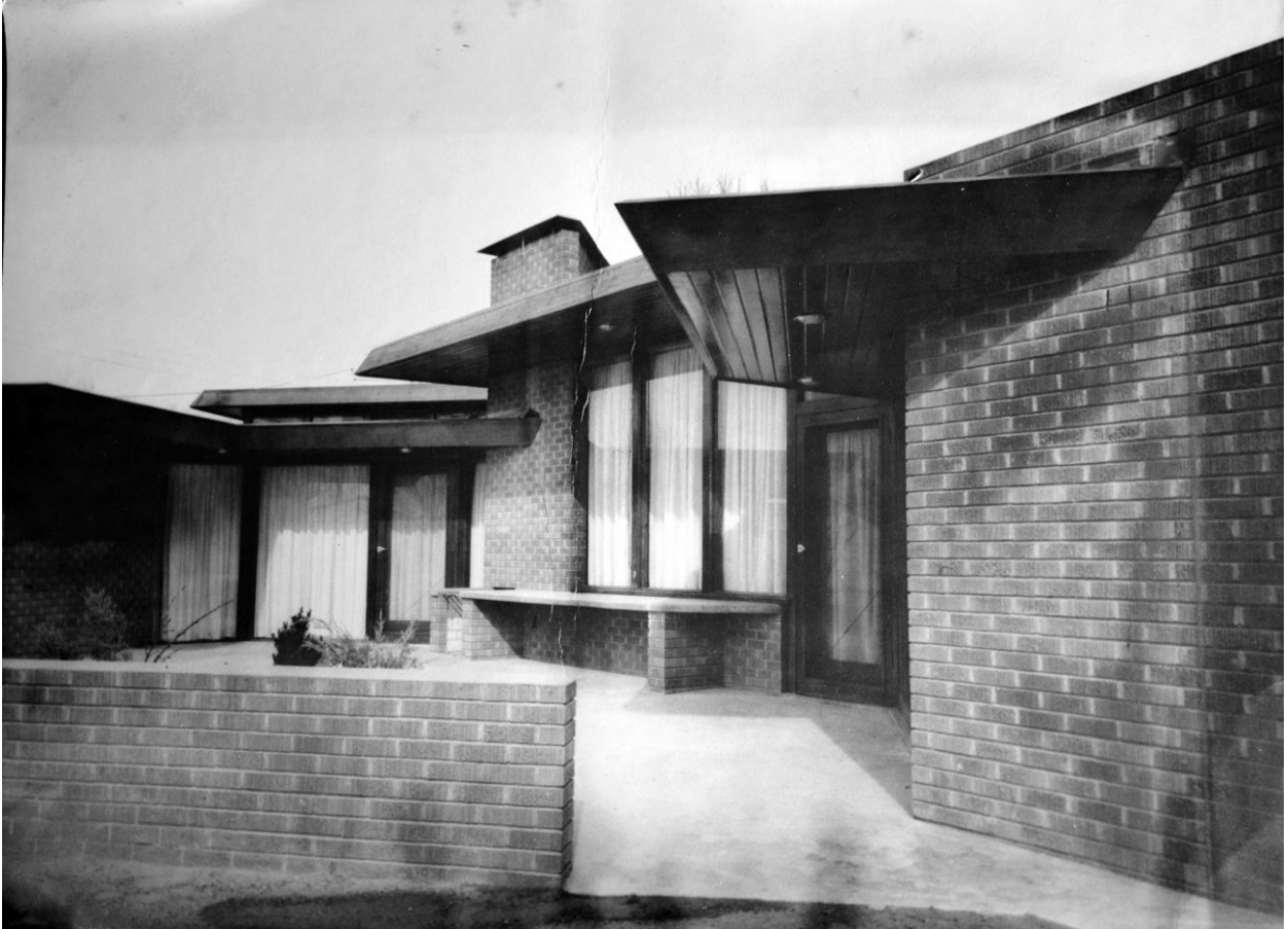
Fig. 6 – Rear patio of the Tweedy-Puntch House, looking north, ca. 1952 (courtesy of Robyn Puntch)
