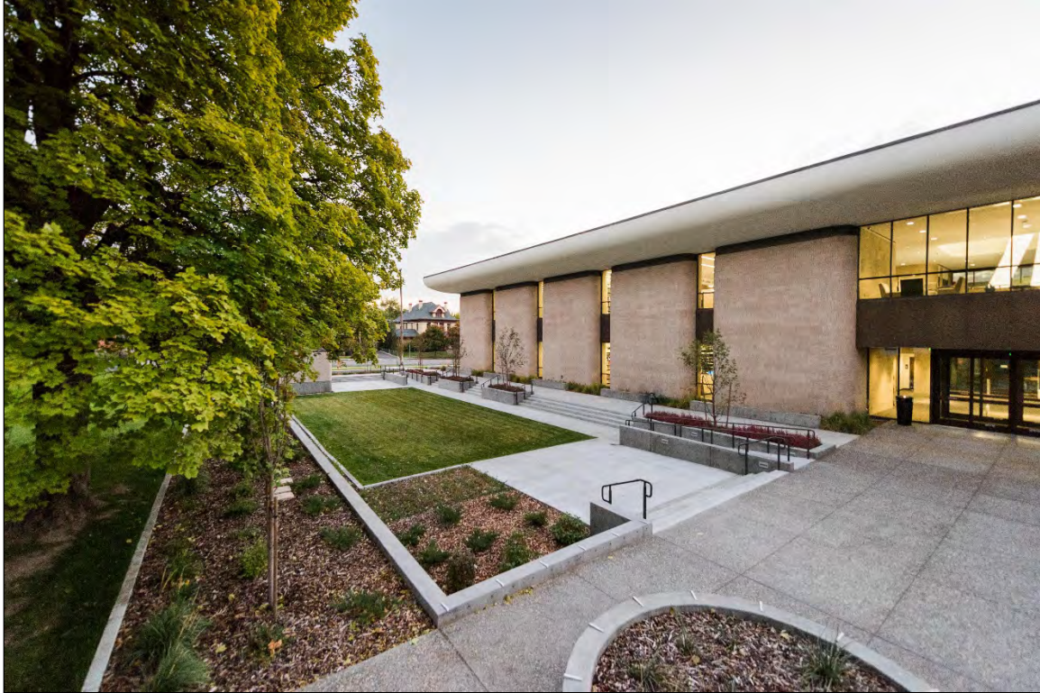
13 of 18 East side of building. Camera facing southwest.
