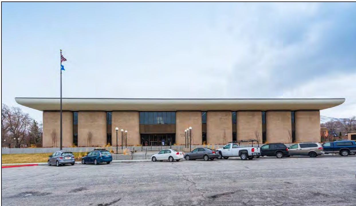
3 of 18 West side of building. Camera facing east.
