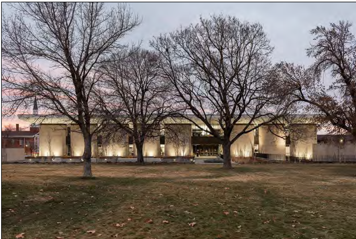
5 of 18 East side of library. Amphitheater on left. Camera facing west.
