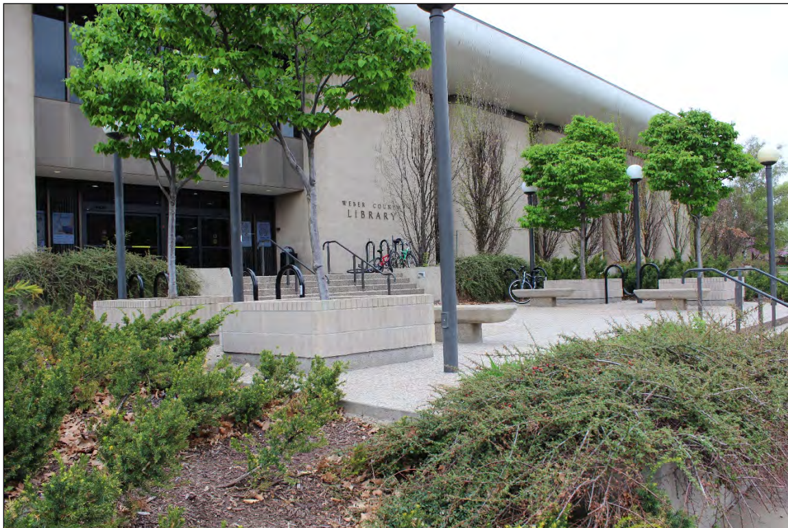
Figure 3. Main entrance to Weber County Main Library as it existed prior to 2018 rehabilitation, west side of building. Note that built features and landscaping have been retained. Camera facing southeast. Photograph by Anne Oliver, April 30, 2014.
