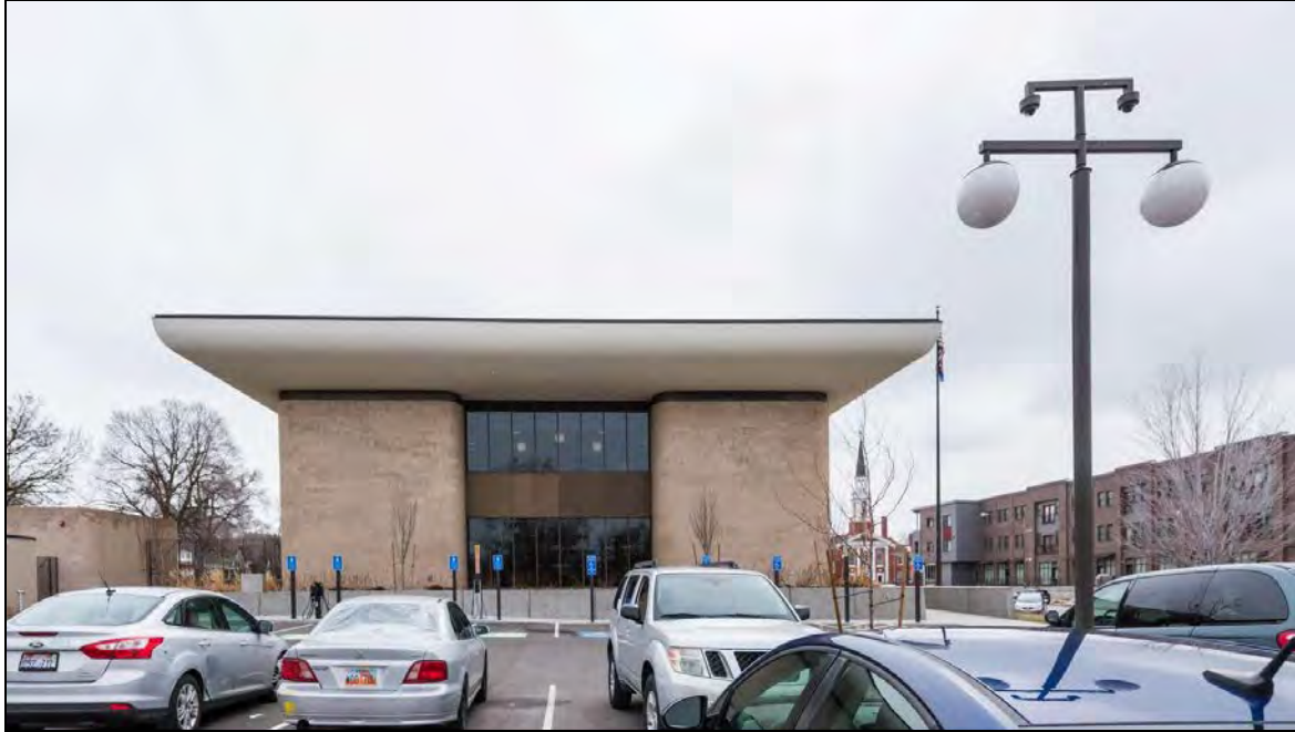
7 of 18 North side of building with parking lot in foreground. Camera facing south.
