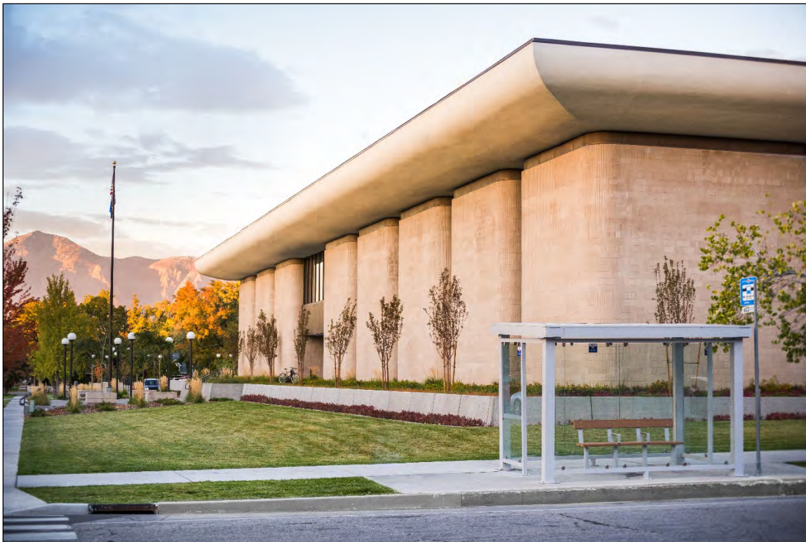
4 of 18 West and south sides of library. Note landscaping and built features leading to main entrance. Camera facing north-northeast.
