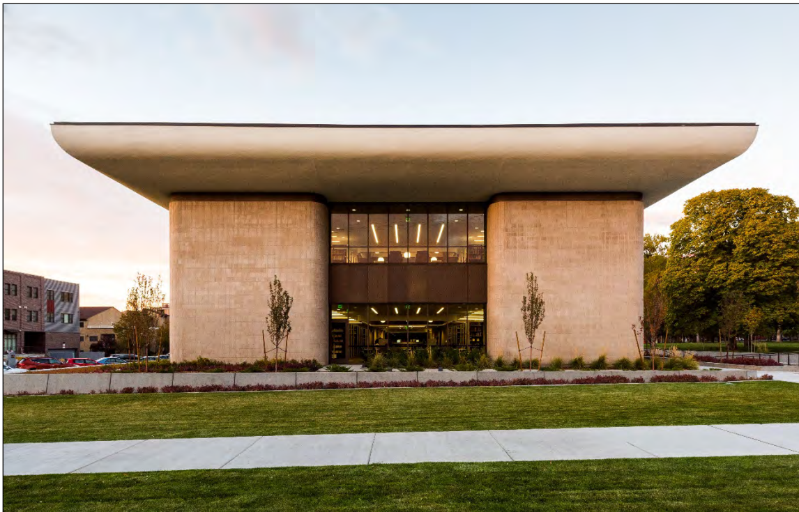
11 of 18 South side of building. Camera facing north.
