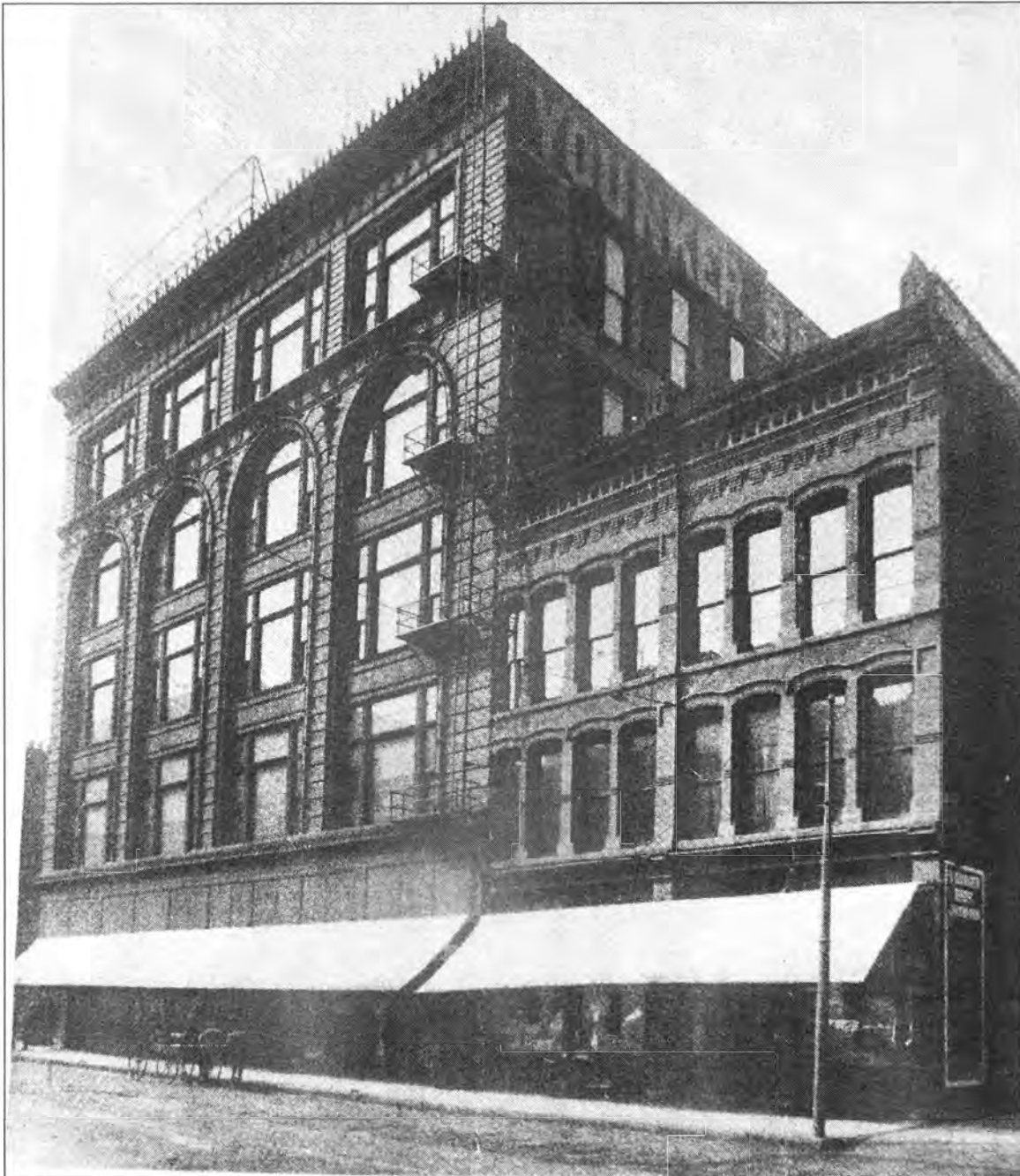
Figure 16, original building, 1899, view southwest on 7 th from alleyway, Meek Block to the right ( Downtown Magazine , December 16, 1981)
