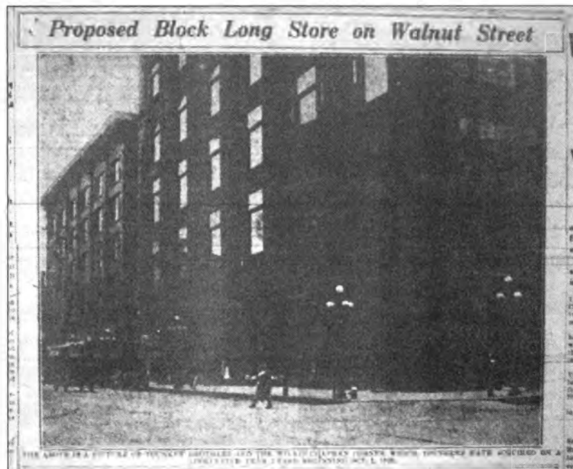
Figure 35: The two buildings, viewing to the northwest from the corner of 7 th and Walnut (note the street lights and the infamous hydrant) ( Tribune , October 16, 1922)
