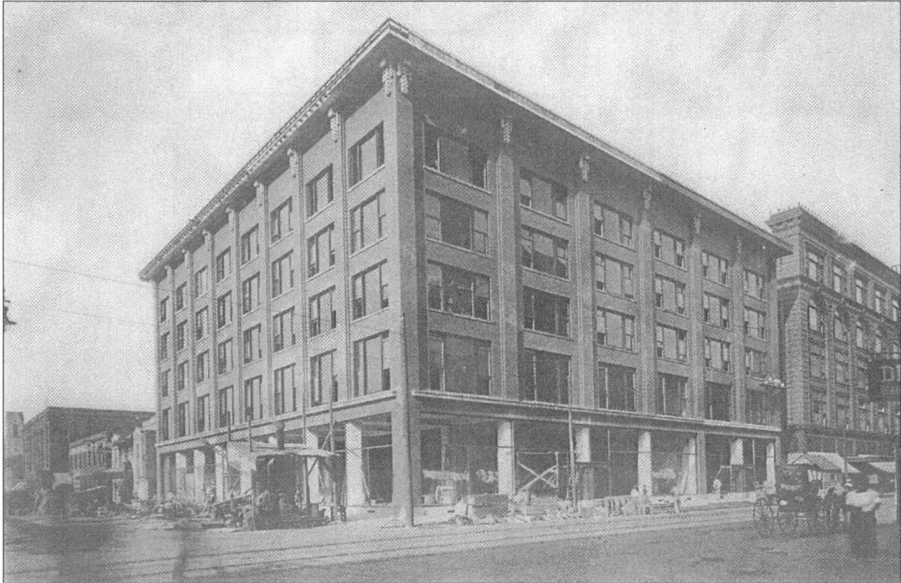
Figure 27: Wilkins Building construction, view northeast, 1908, note the storefront division point between the easternmost two bays and the rest of the building front (original image found in building by architects Kirk Blunk & Associates)
