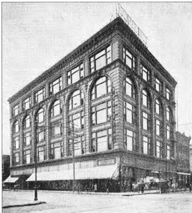
Figure 18, original building, 1904, view northwest from the corner of Walnut and 7 th streets
