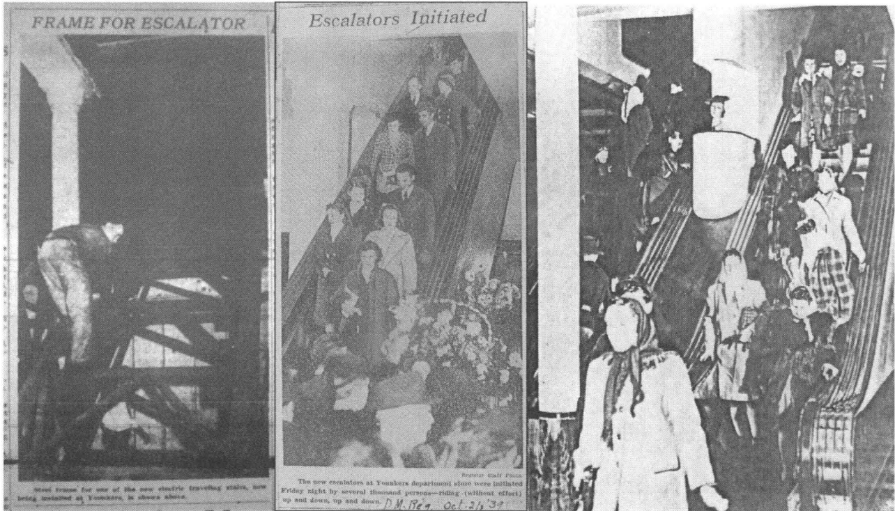
Figure 48: Three escalator images, left to right, installing the frame for the new escalator ( Tribune , June 7, 1939), middle, electric stairway opens, right, in operation 1944 ( Des Moines Register , October 21, 1939; 1944 booklet)
