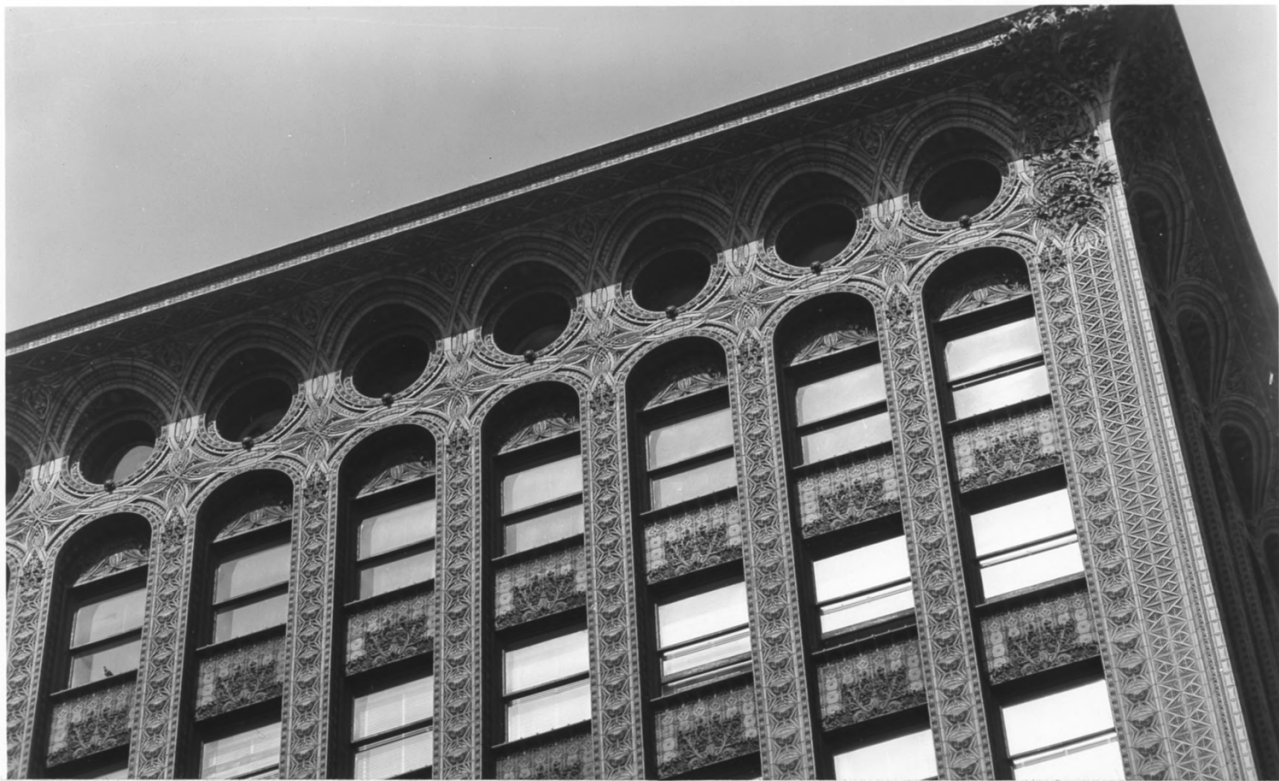
Guaranty (Prudential) Building, Buffalo, New York South cornice
