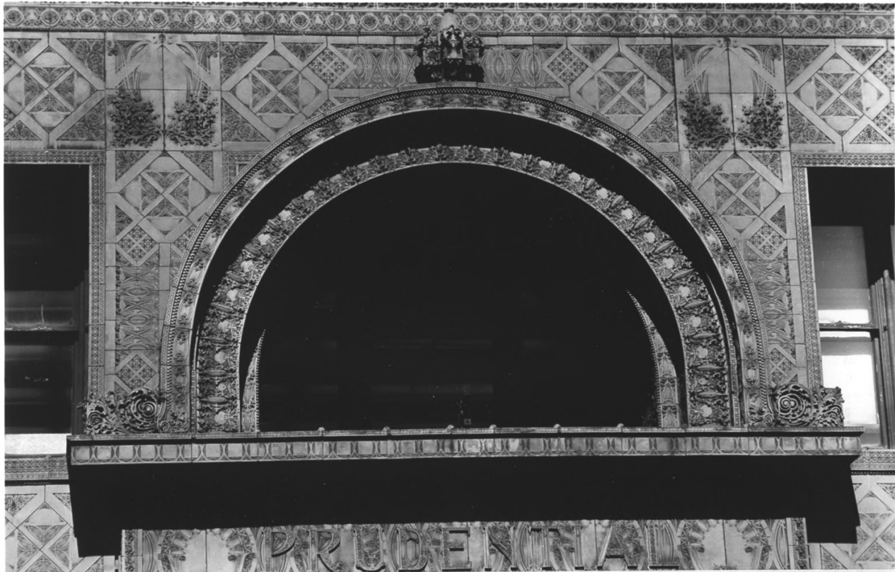
Guaranty (Prudential) Building, Buffalo, New York South entrance, detail
