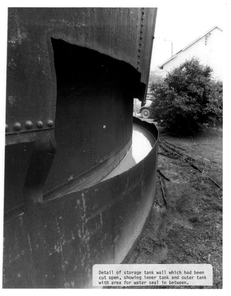
Detail of coal gas storage tank, the side of which had been cut open preliminary to demolition, showing inner tank and outer tank with water seal area between two sections.
