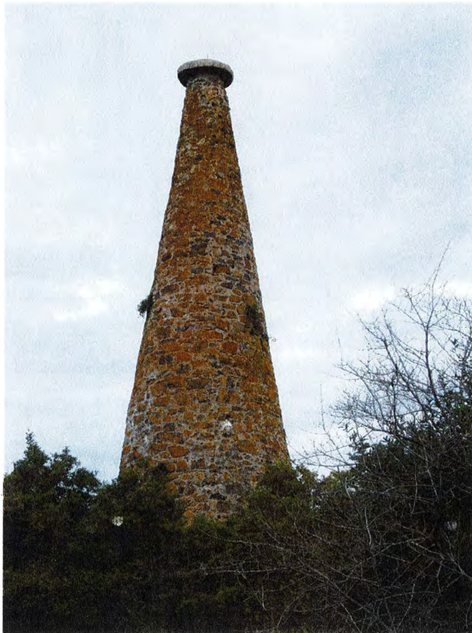
PHOTO 2: TOWER EXTERIOR, CAMERA FACING WEST
