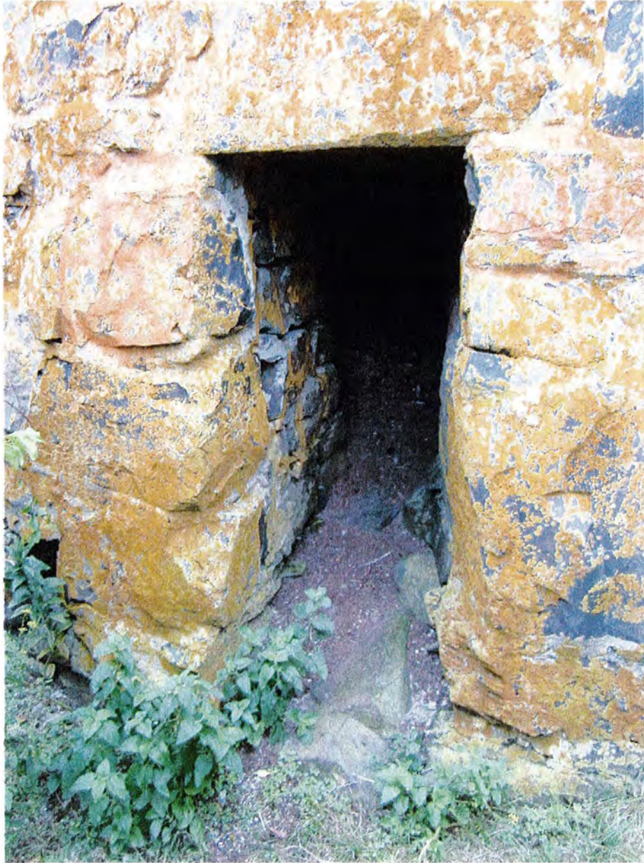
PHOTO 3: TOWER ENTRY, CAMEA FACING EAST
