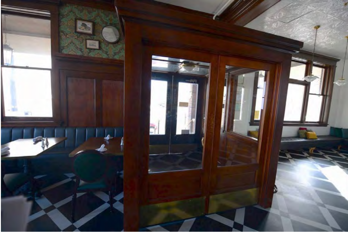
Photo No. 17 of 30, First floor level front double door and vestibule. Camera facing east.
