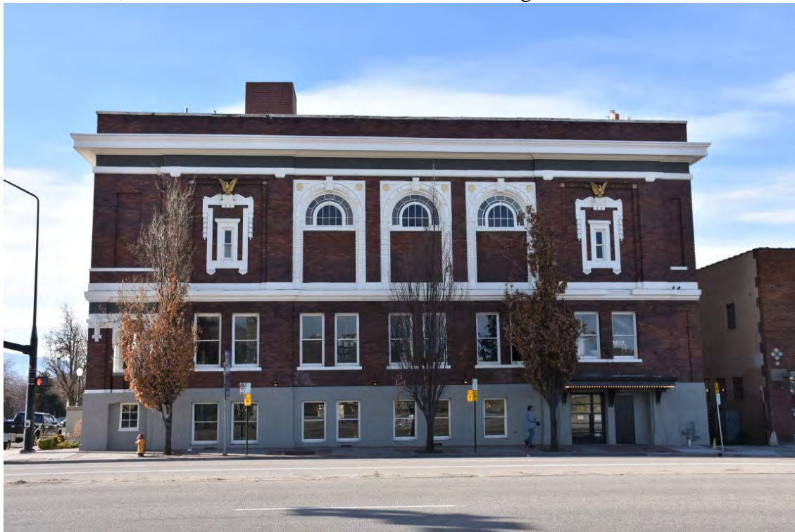
Photo No. 4 of 30, North elevation with context. Camera facing south.
