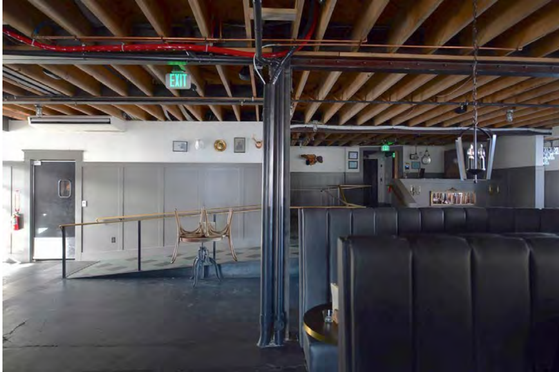
Photo No. 15 of 30, Basement level interior. Camera facing west.
