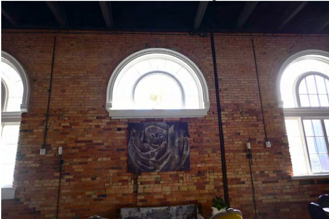
Photo No. 24 of 30, Second floor level interior. Camera facing east.
