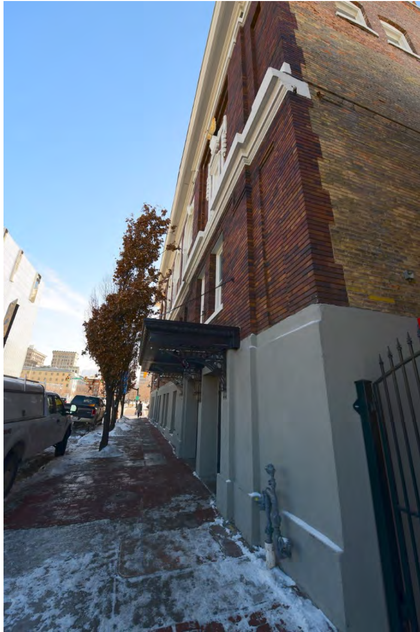
Photo No. 5 of 30, North elevation. Camera facing east.
