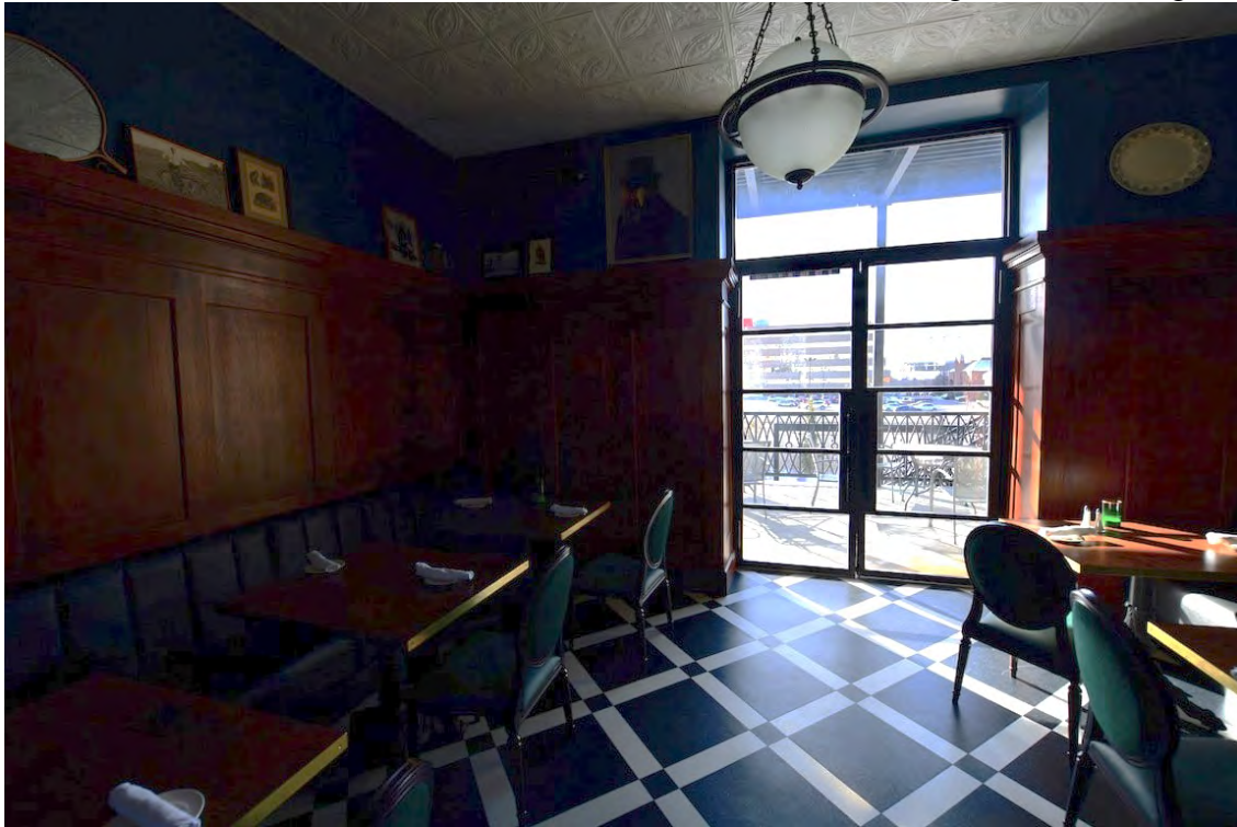
Photo No. 19 of 30, First floor level interior, new exit to exterior decking. Camera facing south.
