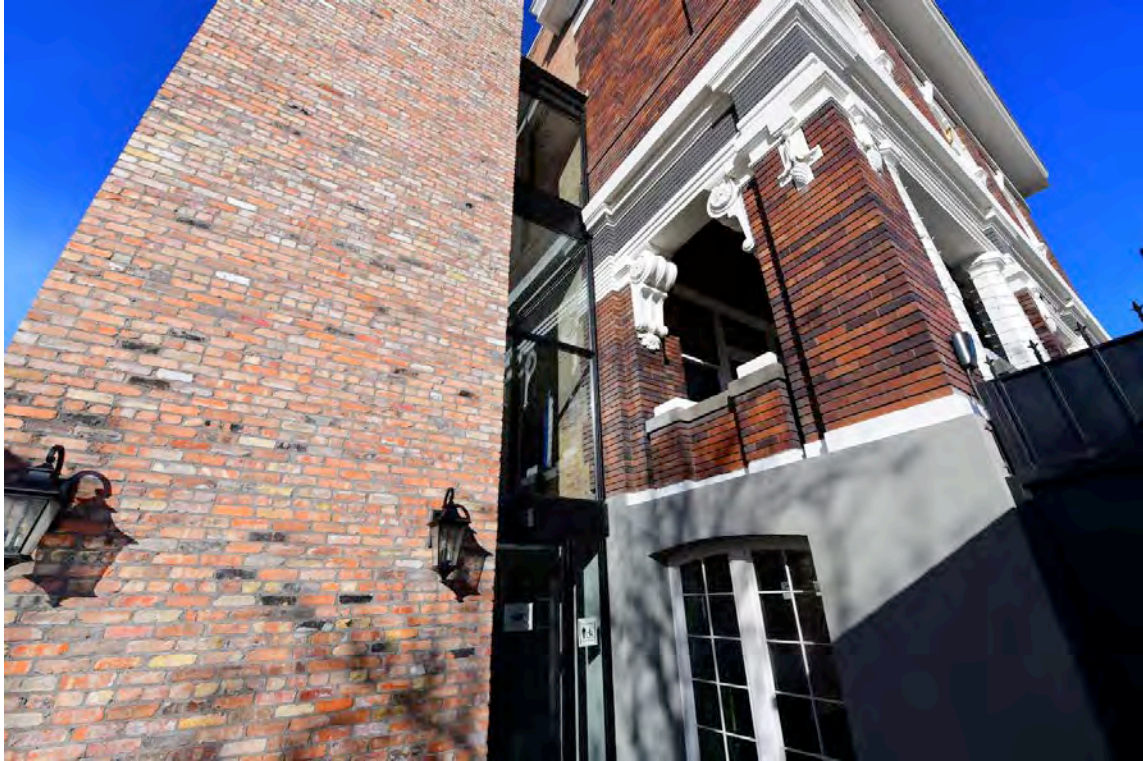
Photo No. 11 of 30, Elevator/stair tower and connection. Camera facing northwest.
