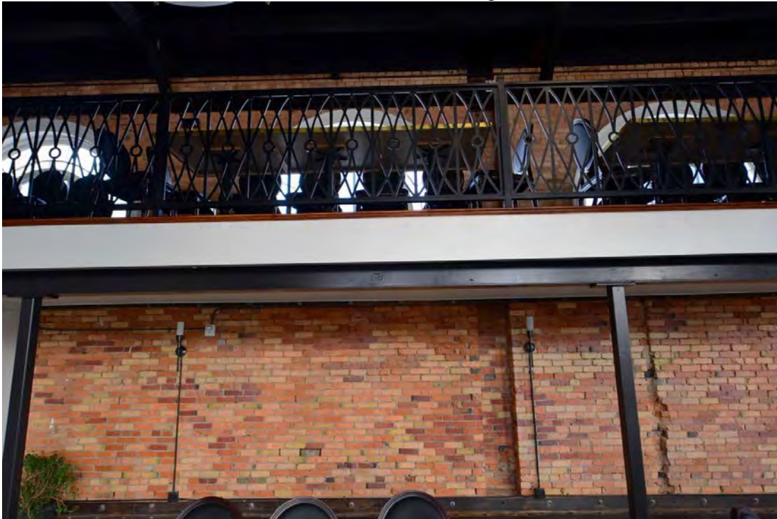
Photo No. 26 of 30, Mezzanine level interior. Camera facing north.
