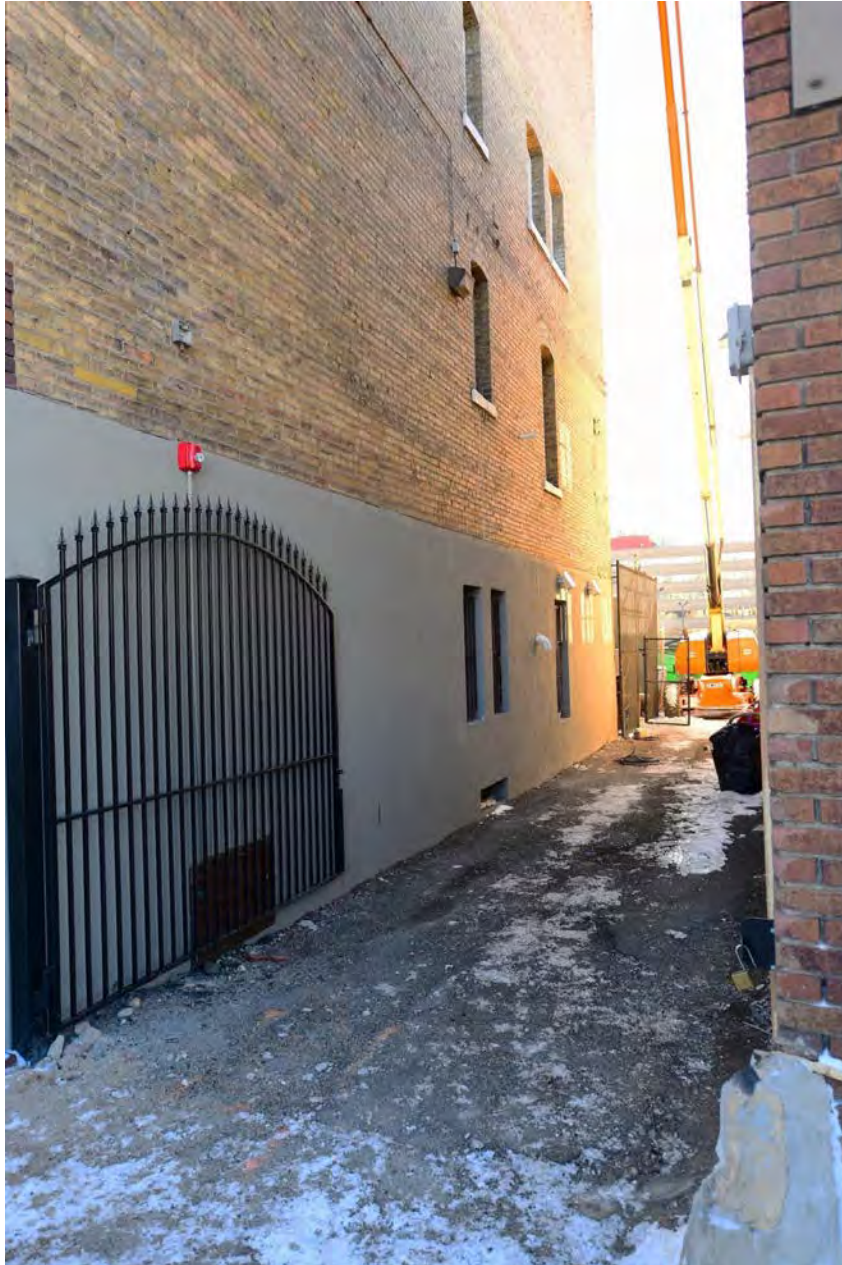
Photo No. 6 of 30, West elevation. Camera facing southeast.
