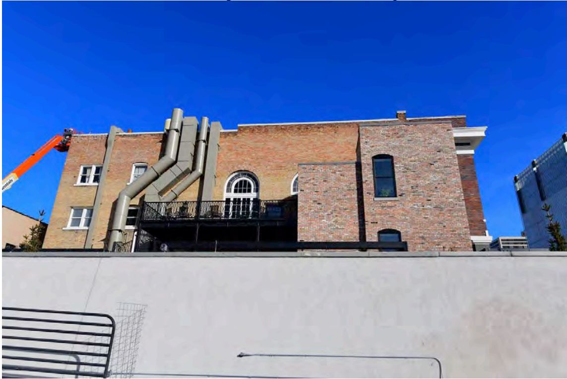
Photo No. 7 of 30, South elevation and plaza fence. Camera facing north.
