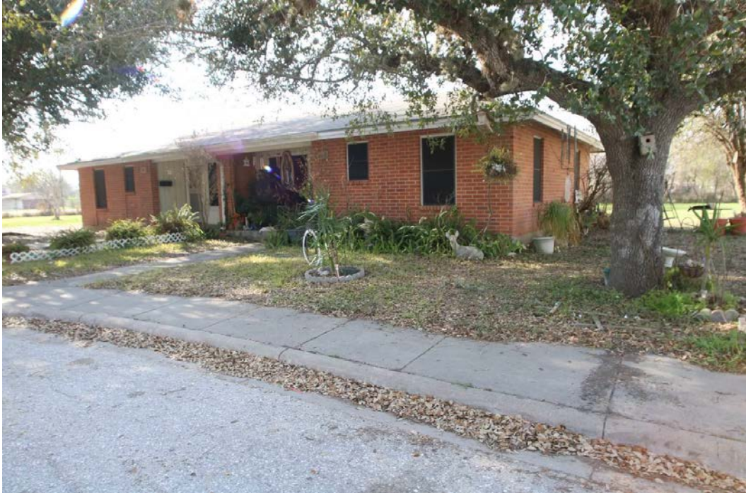
View of Building 21, looking west
