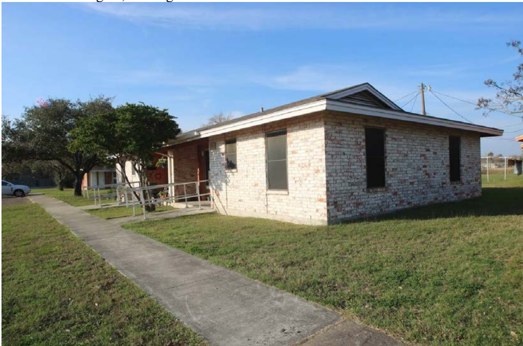
View of Building 25, looking northwest
