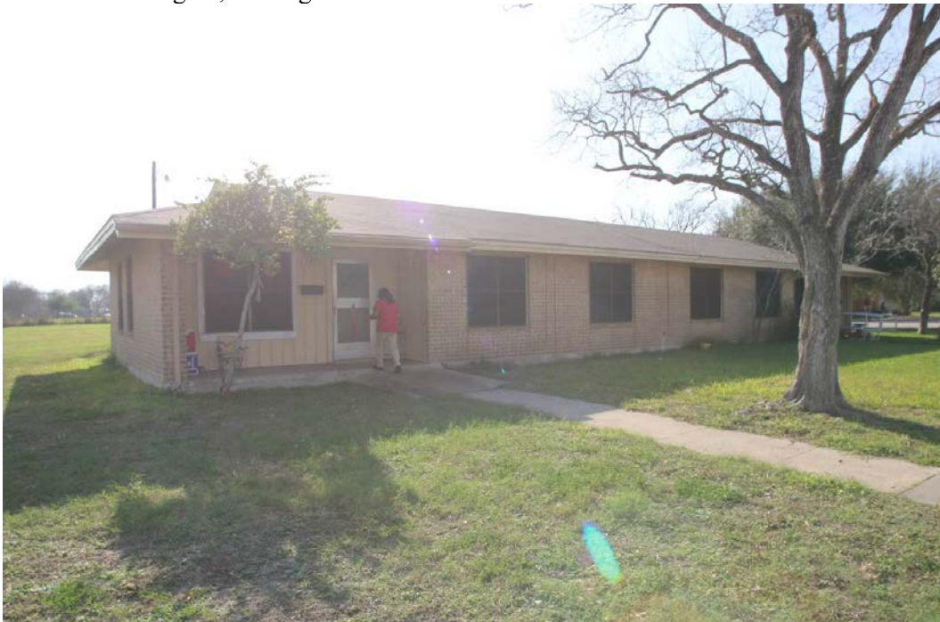
View of Building 17, looking west
