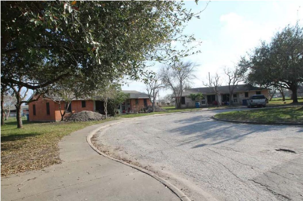
View of Building 18 (left) and Building 19 (right), looking south
