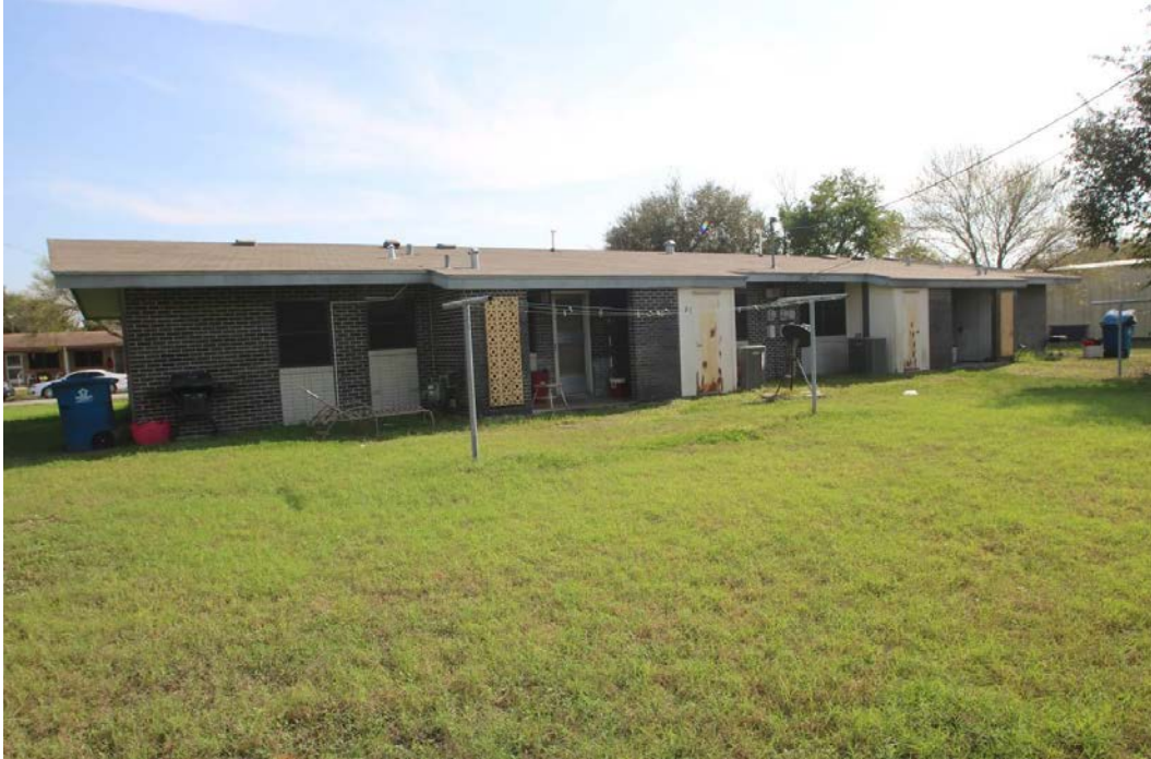
View of Building 15, looking southeast
