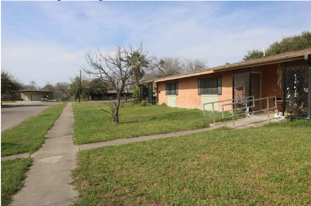
View of Building 13, looking west
