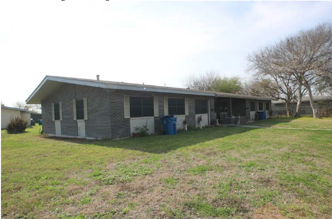
View of Building 16, looking west
