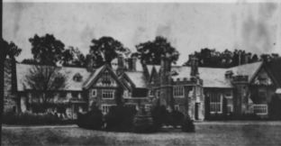
NEW HOME OF THE GENERAL DRAFTING COMPANY AT CONVENT STATION, NEW JERSEY. RECONSTRUCTION BY JOSEPH DOLBE, INC., BERNARDVILLE.
