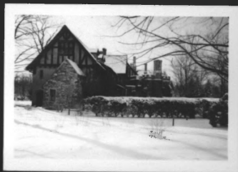
Left, Glynallyn as it appeared in the American Architect, February 4, 1920. The photo below shows the chimney at the extreme left has disappeared. This was removed because workmen were not able to find and repair a leak. Though not visible in these pictures, another chimney at the west end of the house was also removed. Smaller photo was taken January 1953.
