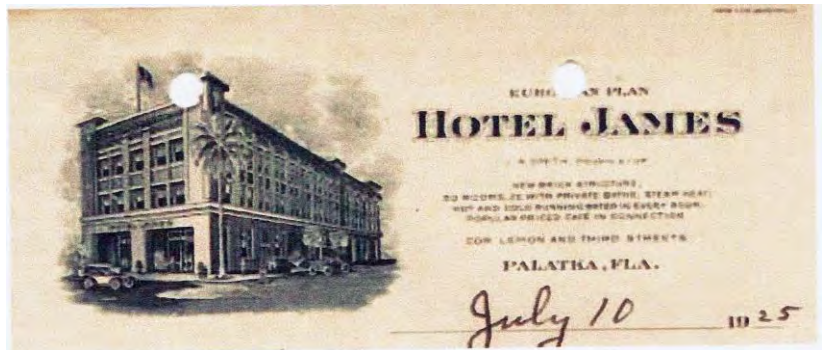
Business card of Hotel James shortly after completion of 1924 addition, circa 1925
