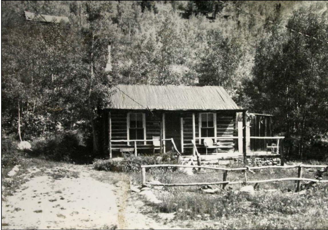
Figure 5. This ca. 1970s-80s view north shows the front of the cabin. Courtesy of Chaffee County Assessor, appraisal photograph, Salida, Colorado.
