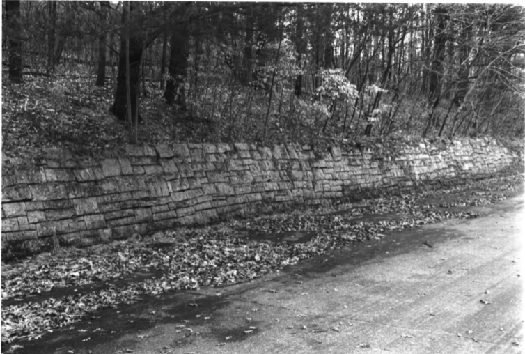
WHITEWATER STATE PARK WINONA CO., MN STRUCTURE #9 PHOTO I.D. 09342#1
