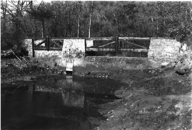
WHYMEWATER STATE PARK WINONA CO., MN STRUCTURE # 16 PHOTO I.D. 09342 #16
