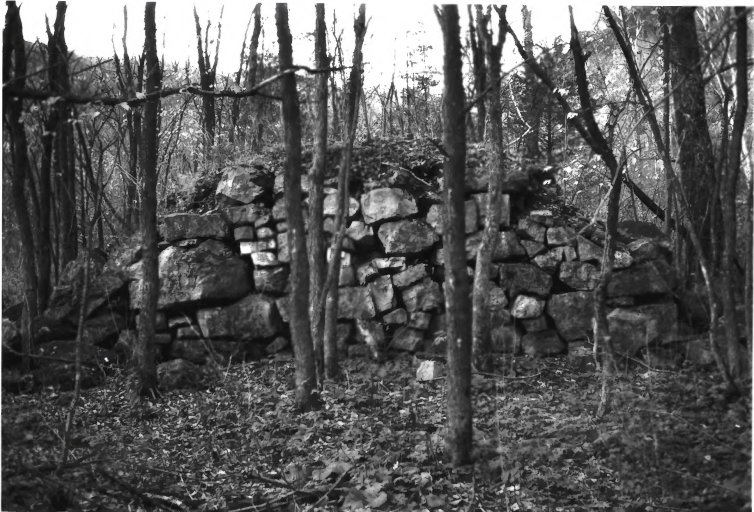
WHITEWATER STATE PARK WINONA CO., MN STRUCTURE #30 PHOTO I.D. 09344#11
