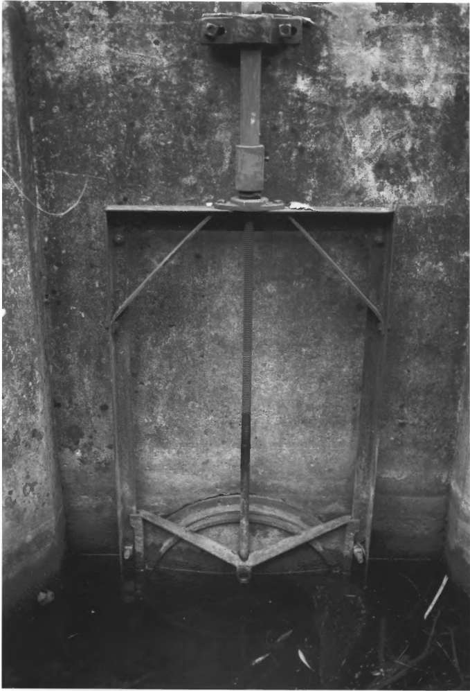
WHITEWATER STATE PARK WINONA CO. MN. STRUCTURE # 14 PHOTO I.D. 09341 # 7
