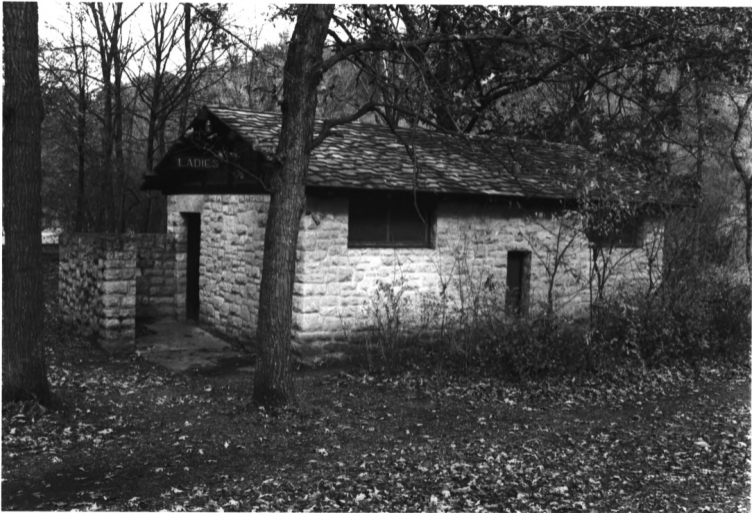
WHITEWATER STATE PARK WINONA CO., MN BLDG # 10, PHOTO I.D. 09342 #8
