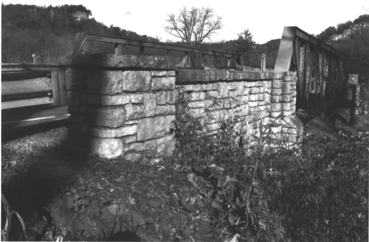
WHITEWATER STATE PARK WINONA CO. MN STRUCTURE # 4 PHOTO I.D. 09342 # 23
