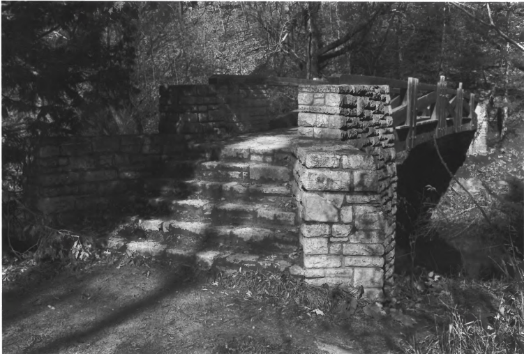
WHITEWATER STATE PARK WINONA CO., MN STRUCTURE #18 PHOTO I.D. 09342#15
