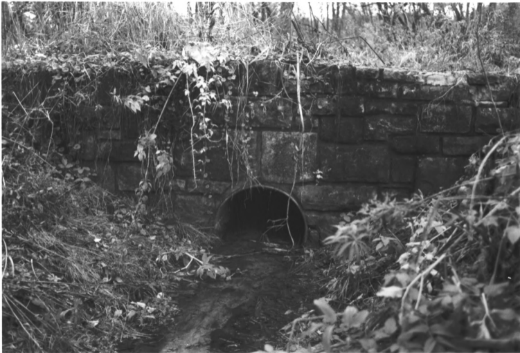
WHITEWATER STATE PARK WINONA CO., MN STRUCTURE # 21 PHOTO I.D. 09341 #21
