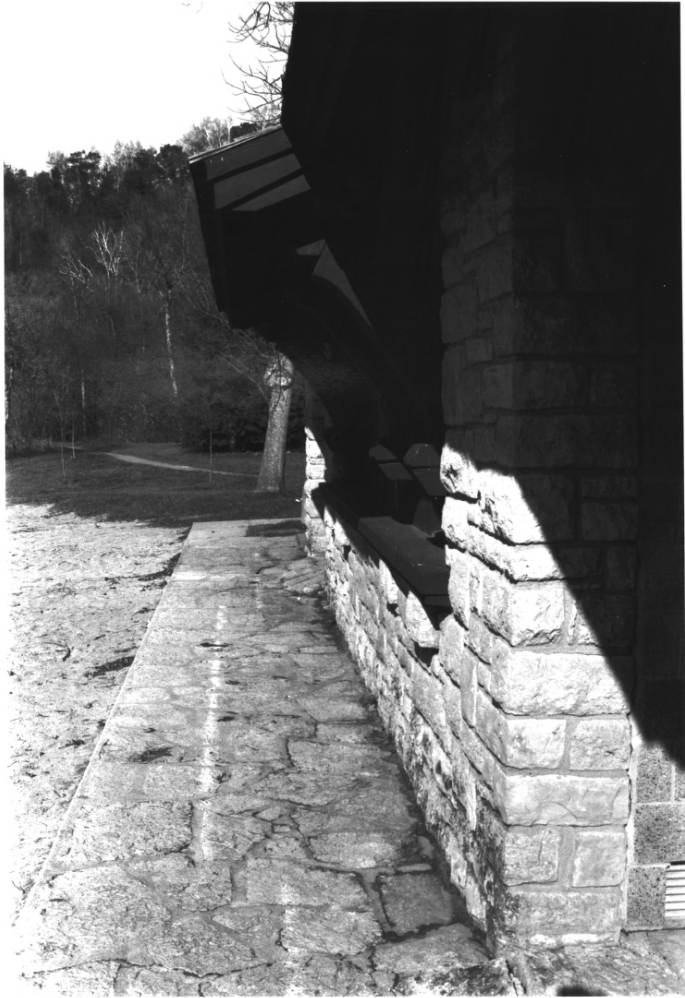
WHITEWATER STATE PARK WINONA CO., MN BLDG #17, PHOTO I.D. 09342 #18
