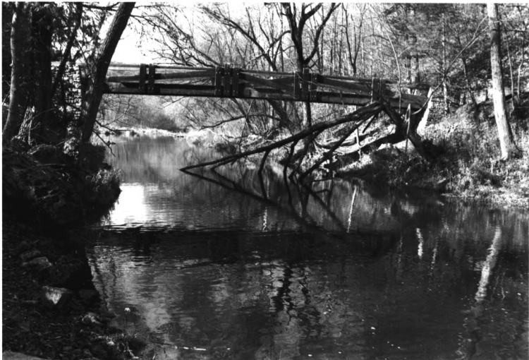
WHITEWATER STATE PARK WINONA CO. MN STRUCTURE #18 PHOTO I.D. 09342 #14
