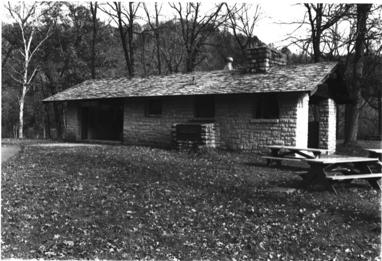
WHITEWATER STATE PARK WINONA CO., MN BLDG # 12' PHOTO I.D. 09342 #10
