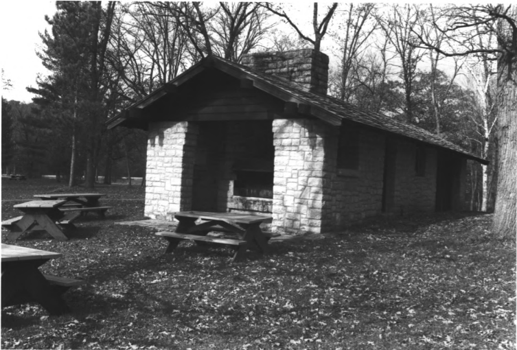
WHITEWATER STATE PARK WINONA CO., MN BLDG # 12 PHOTO I.D. 09342#9
