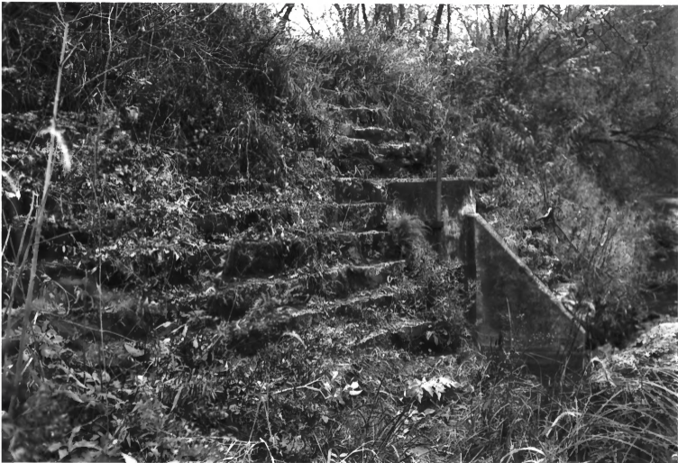
WHITEWATER STATE PARK WINONA CO, MN STRUCTURE #14 PHOTO I.D. 09341#8
