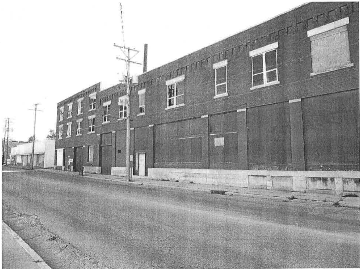
Photo 5. Façade from the north.
