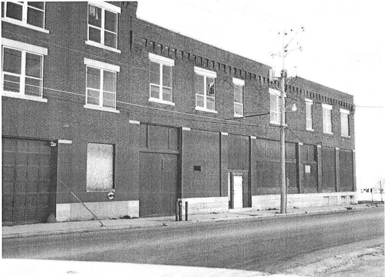
Photo 3. North end of façade.
