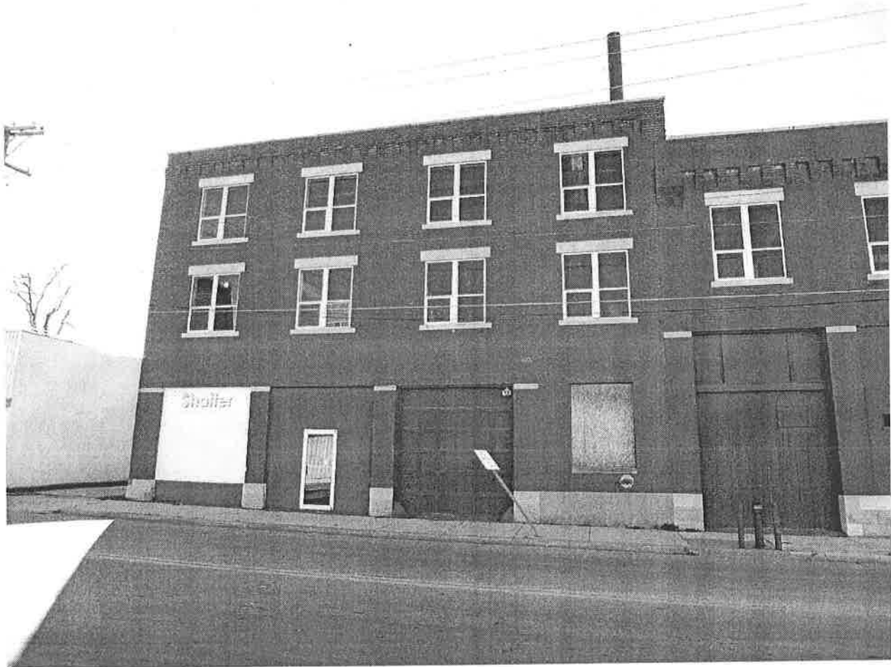
Photo 2. South end of façade. (East wall)
