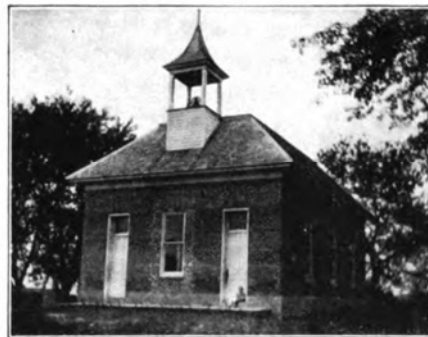
Rochester Schoolhouse After Rebuilding
