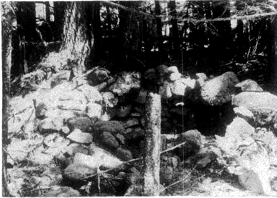
Fig. 21 1996 photo Stone dome oven collapsed at Tunnel Creek camp site, segment W723A.
