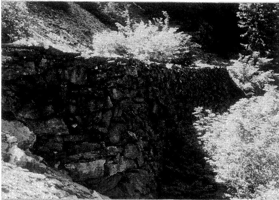
Fig. 19 1996 photo Stone wall supports grade on segment W710B. This wall was built by G.B. Hunt's workers in 1887.
