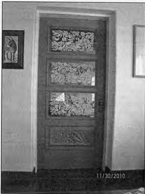
Photograph #11 Leonie Salter painted door, camera facing east.
