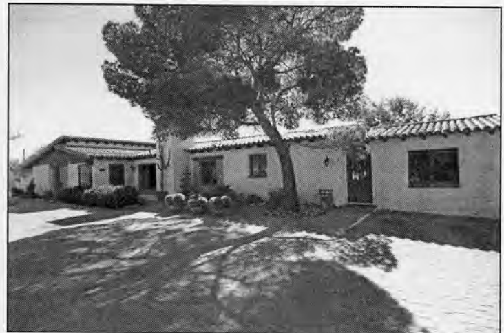
Photograph #4 North façade, camera facing southeast.
