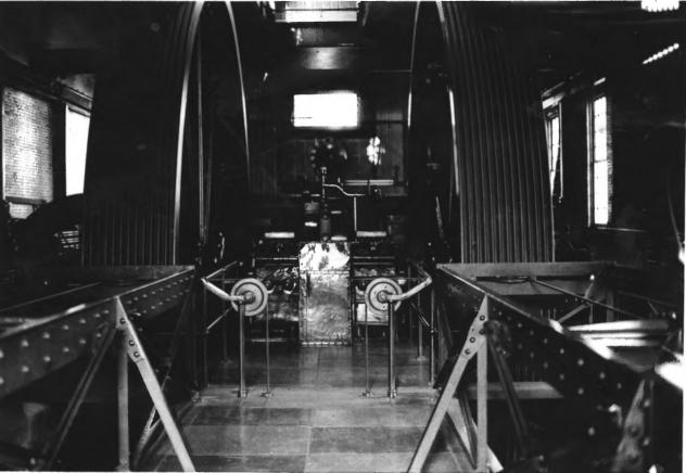
BIG HOLE PUMP STATION Near Divide, MT Silver Bow COunty Pump #2, showing double wheels strung with 1800 continuous feet of manilla hemp. Photo: Miles Tutthell 1 5 1980
