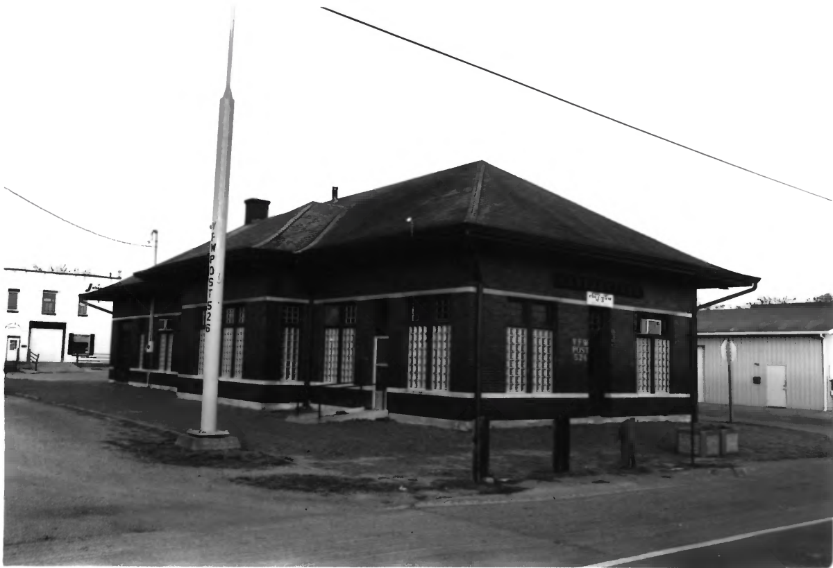
CHICAGO BURLINGTON & QUINCY PASSENGER DEPOT APPANOOSE COUNTY, IA # 2
