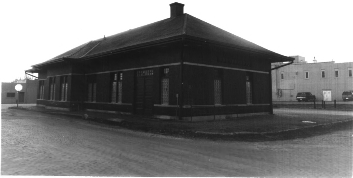
CHICAGO BURLINGTON & QUINCY PASSENGER DEPOT APPANOOSE COUNTY, IA #5
