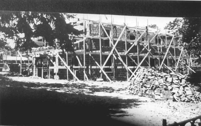
3 of 16 Historic view, 1924, south and east elevations. Curtis Cross construction photo, showing tile block being laid up for exterior walls.
