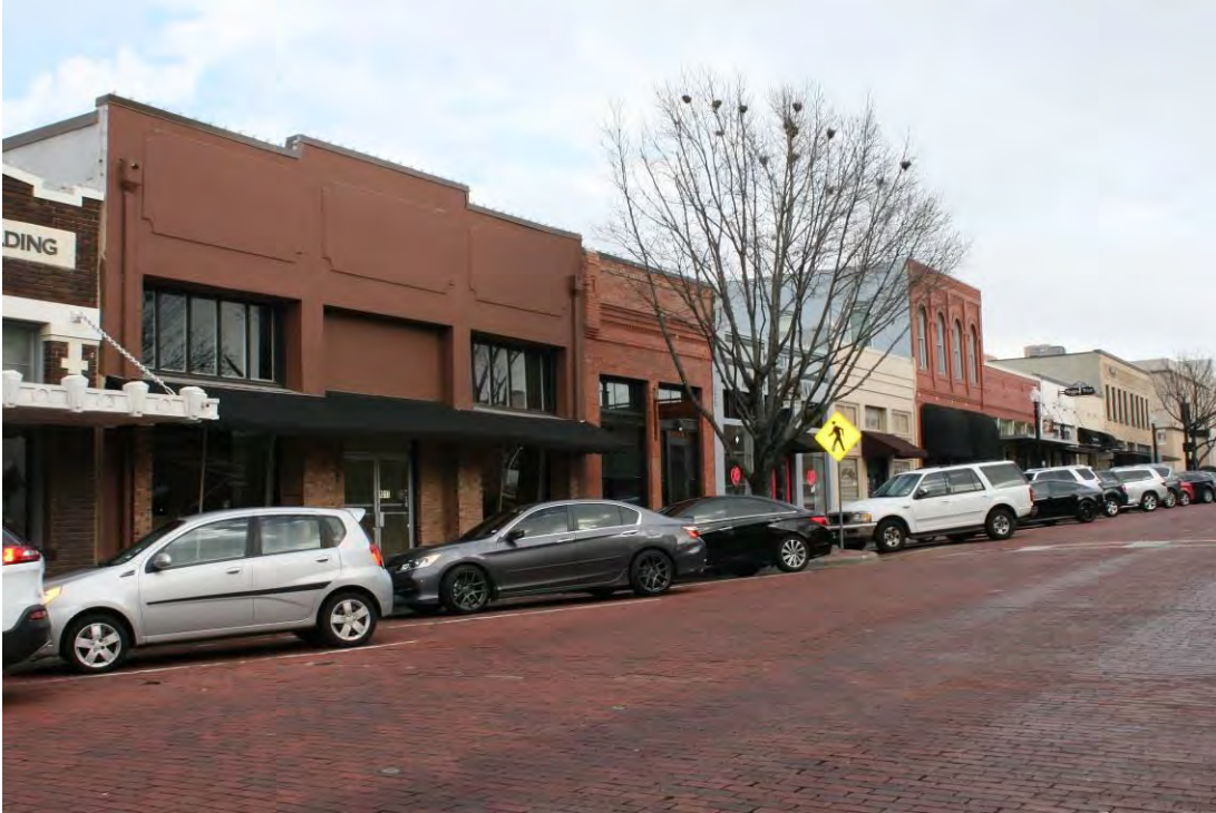
Photo 5: Looking northeast at left to right, 1017, 1021, 1023-25, 1027, 1029, 1031-33, 1035, and 1039 E. 15 th Street.
