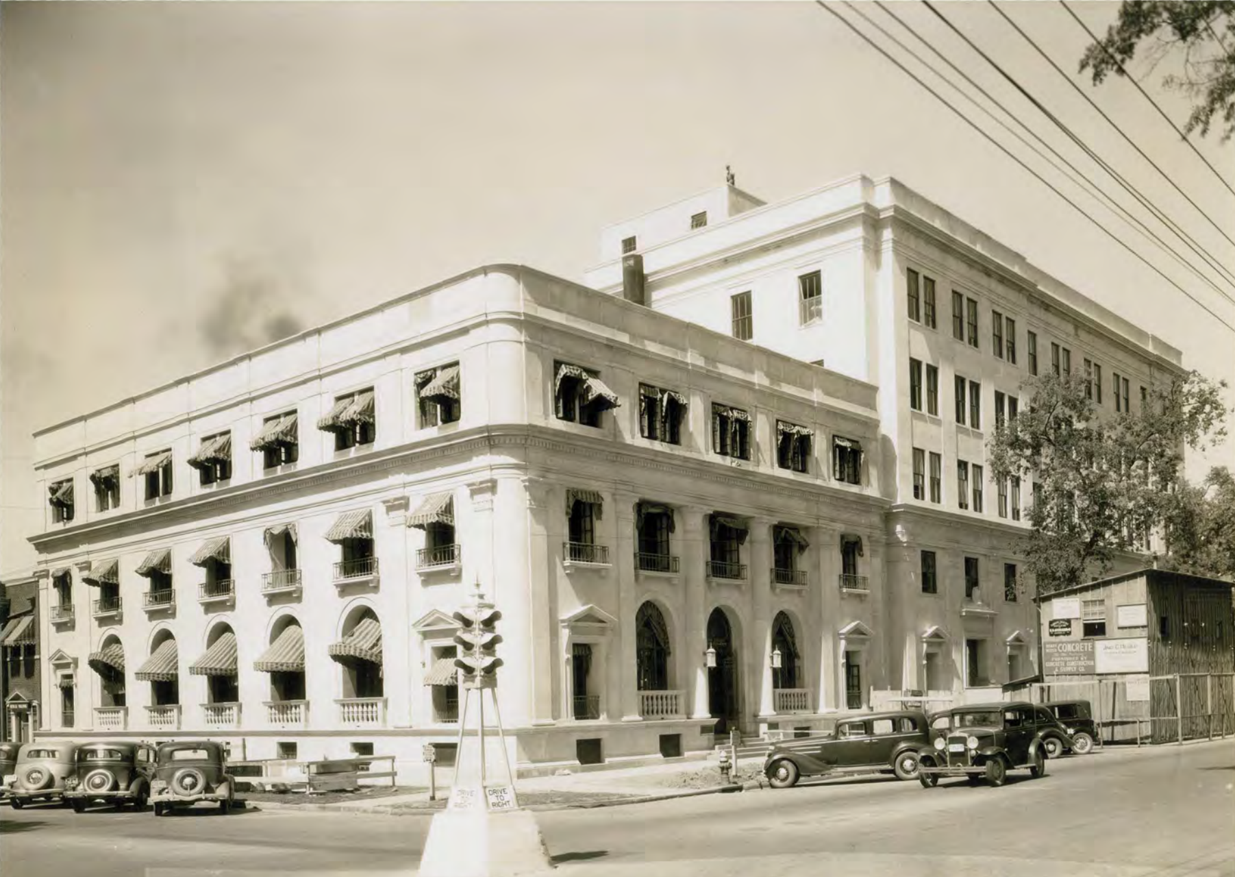
FEDERAL LAND BANK BUILDING · COLUMBIA, S. C. J. C. HESLEP, CONTRACTOR - 30-35 LAFAYE & LAFAYE, ARCHT.
