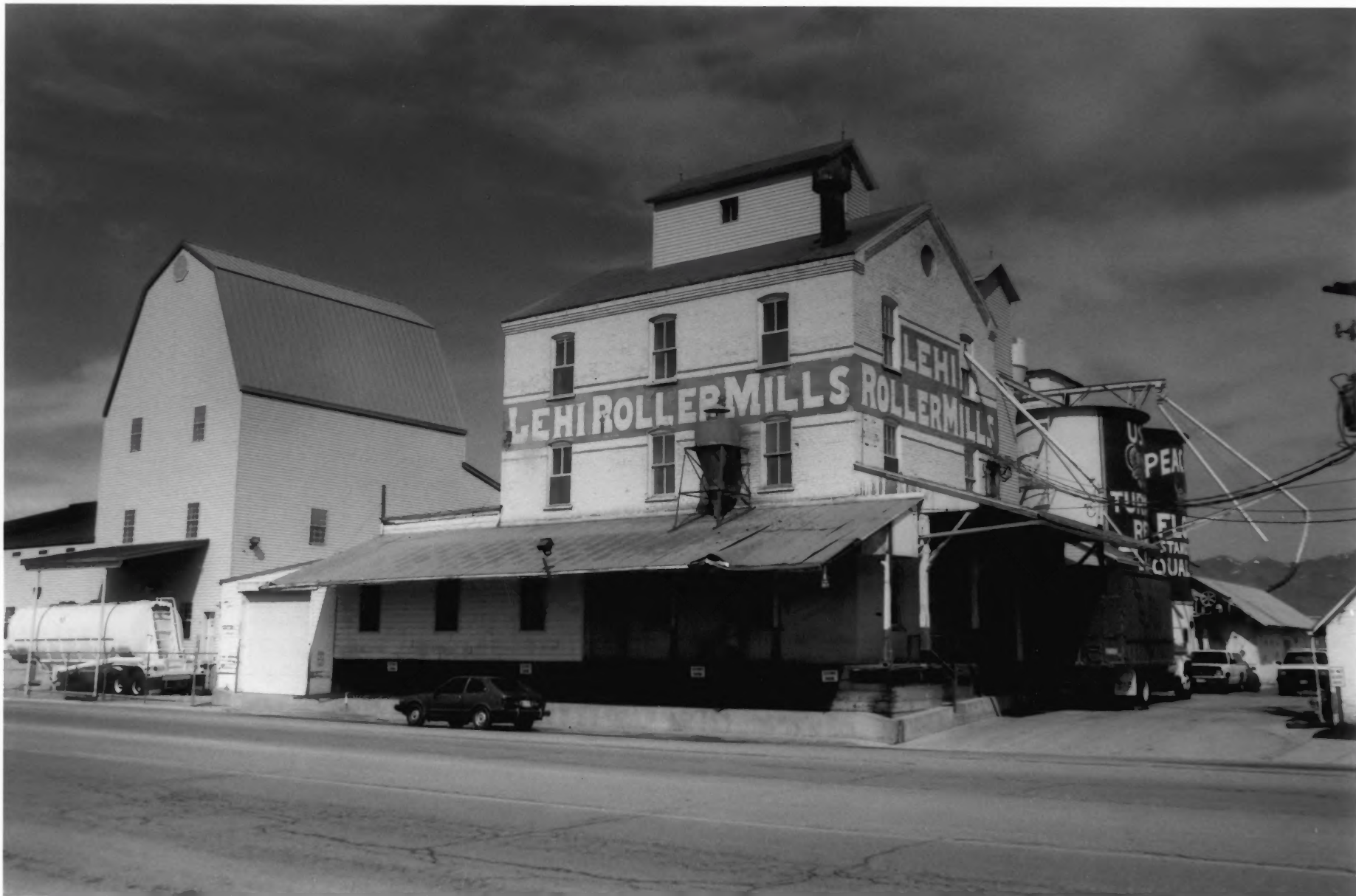
LEHI ROLLER MILLS LEHI, UTAH COUNTY, UTAH PHOTO # 2
