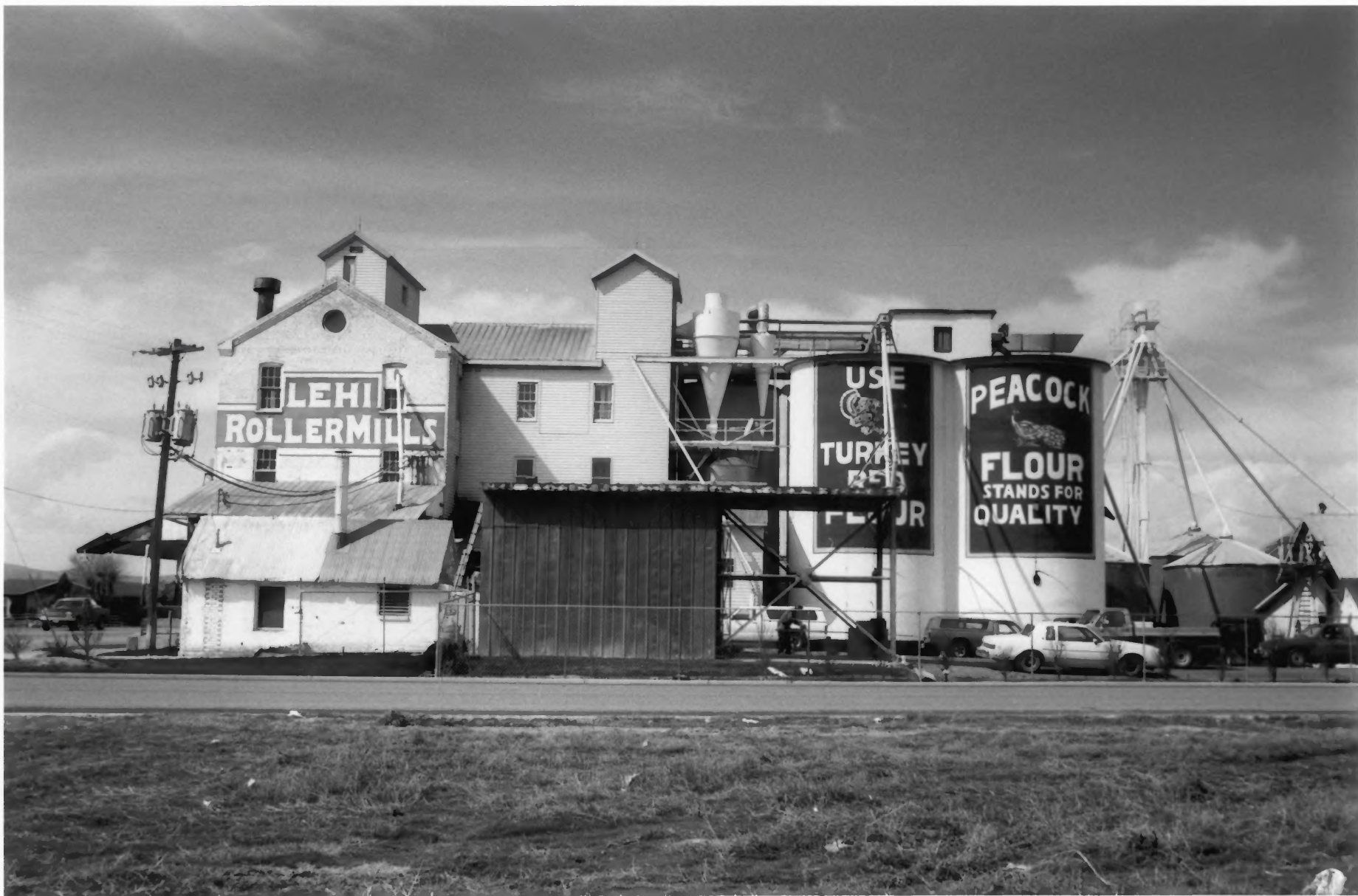
LEHI ROLLER MILLS LEHI, UTAH COUNTY, UTAH PHOTO # 1
