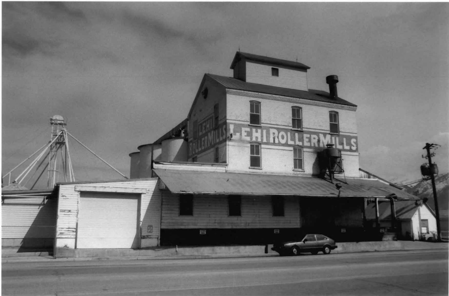
LEHI ROLLER MILLS LEHI, UTAH COUNTY, UTAH PHOTO # 3
